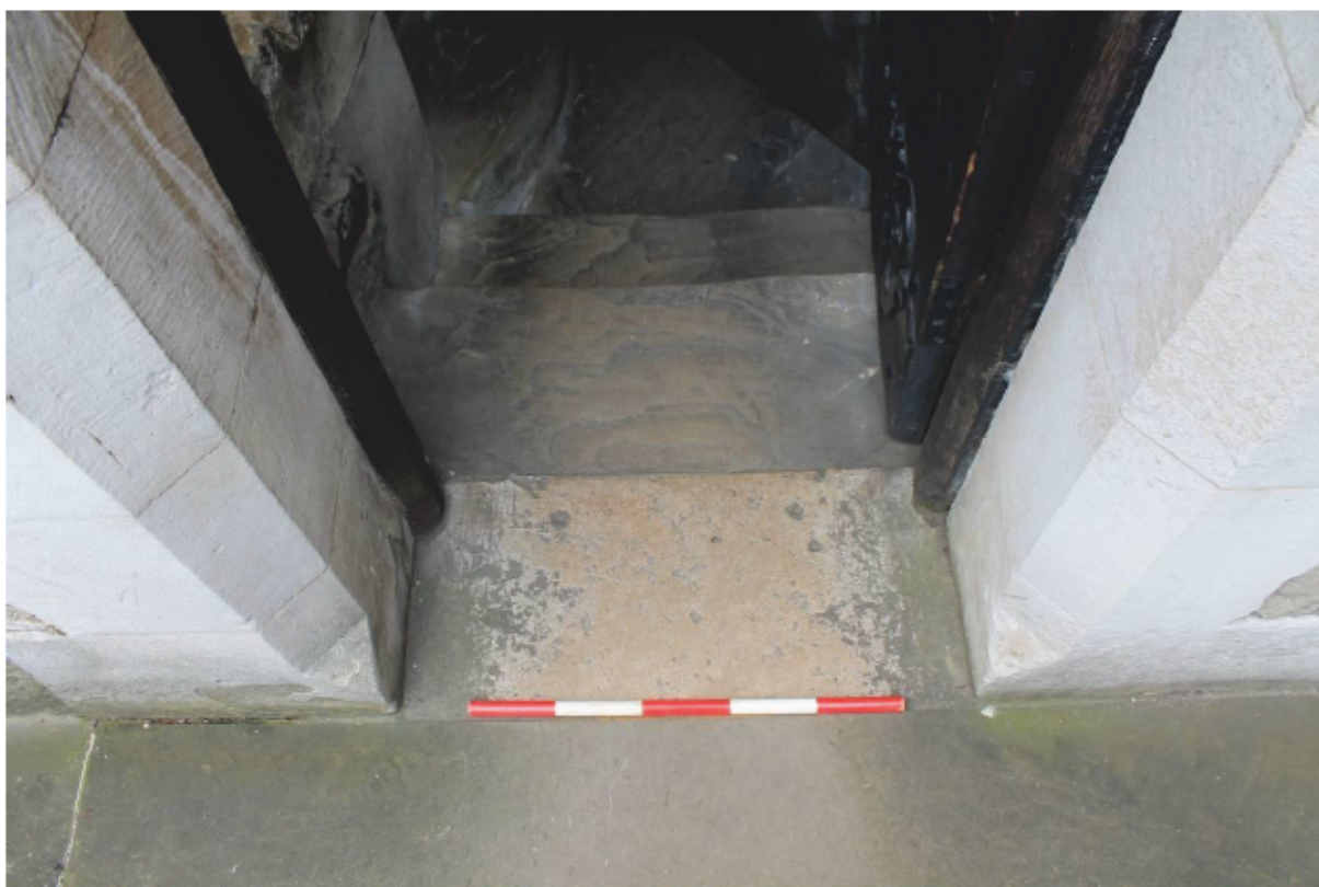
Plate 2 Flush threshold to northern first floor door opening looking south
