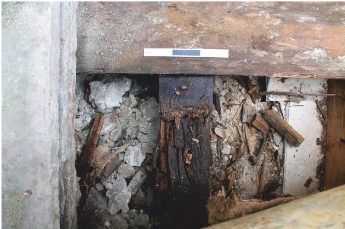
Plate 10 Decayed roofing joist to be replaced (note re-used plasterboard below adjacent joist), looking west
