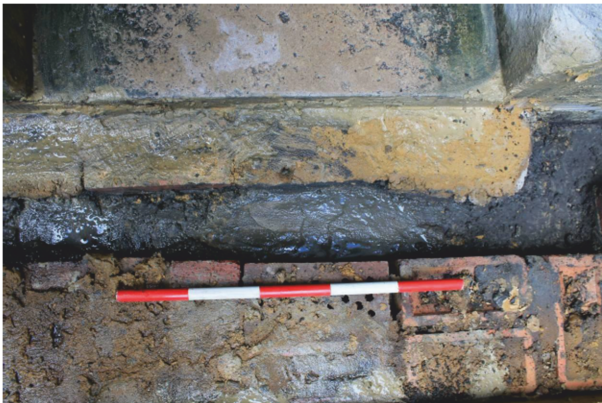
Plate 7 Yorkstone base to drainage gully
