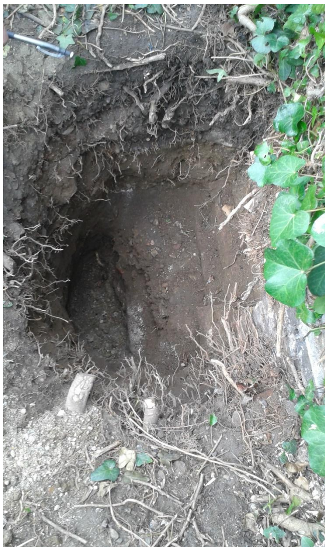
Plate 1: Test Pit 1 facing north. Concrete foundation is on the right of the base of the test and natural gravel is on the left.
