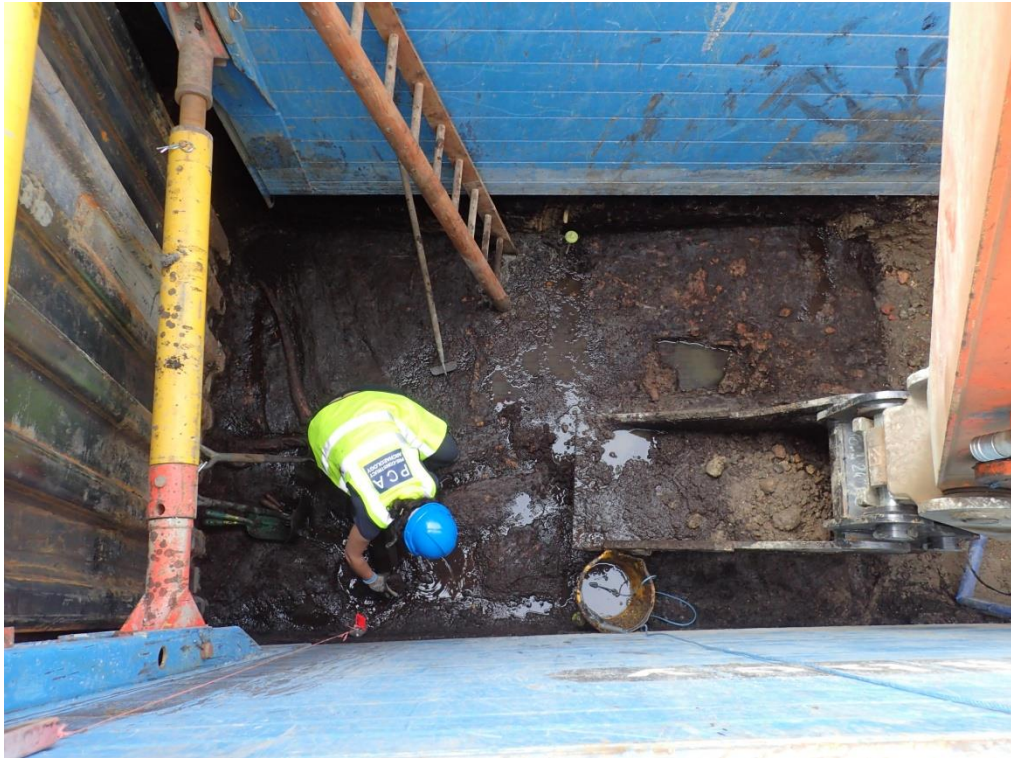
Plate 5: Trench 1C Working Shot, facing south
