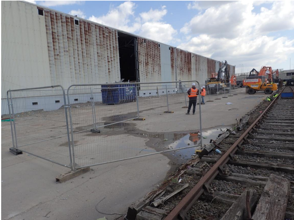
Plate 13: Trench 2 Location, facing north-east
