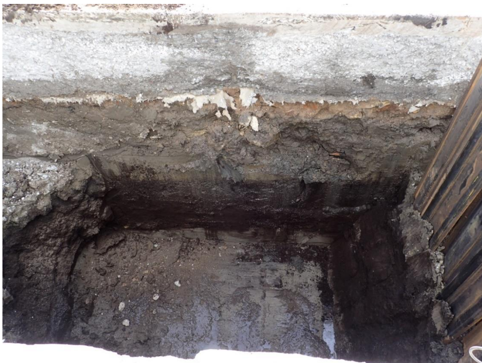
Plate 1: Trench 1A North Facing Section (Facing South)
