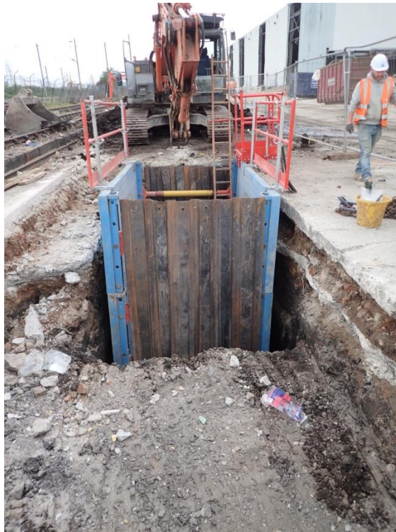
Plate 16: Working Shot of Shoring Box, facing west
