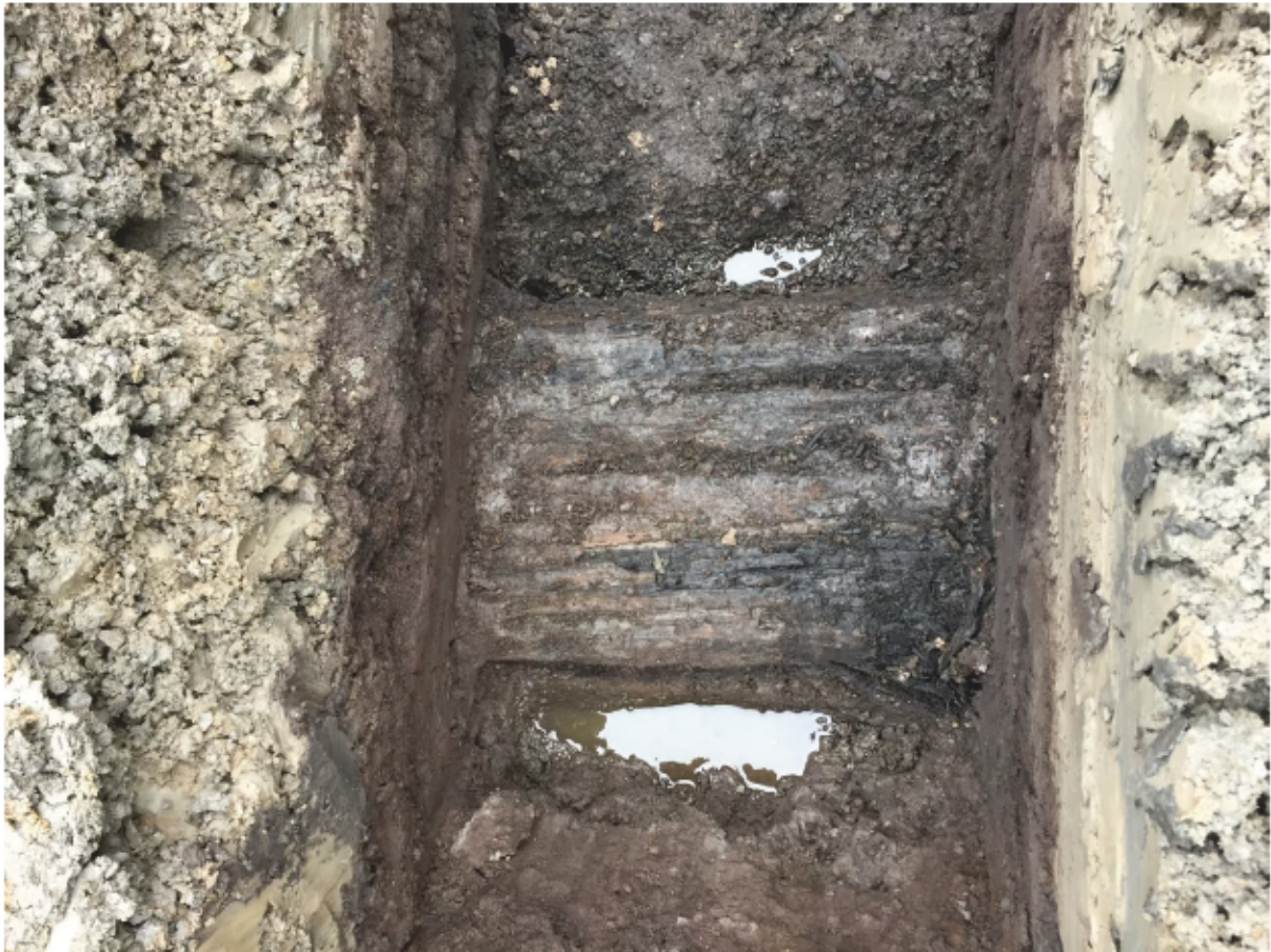
Plate 22: Trench 14 timber looking north
