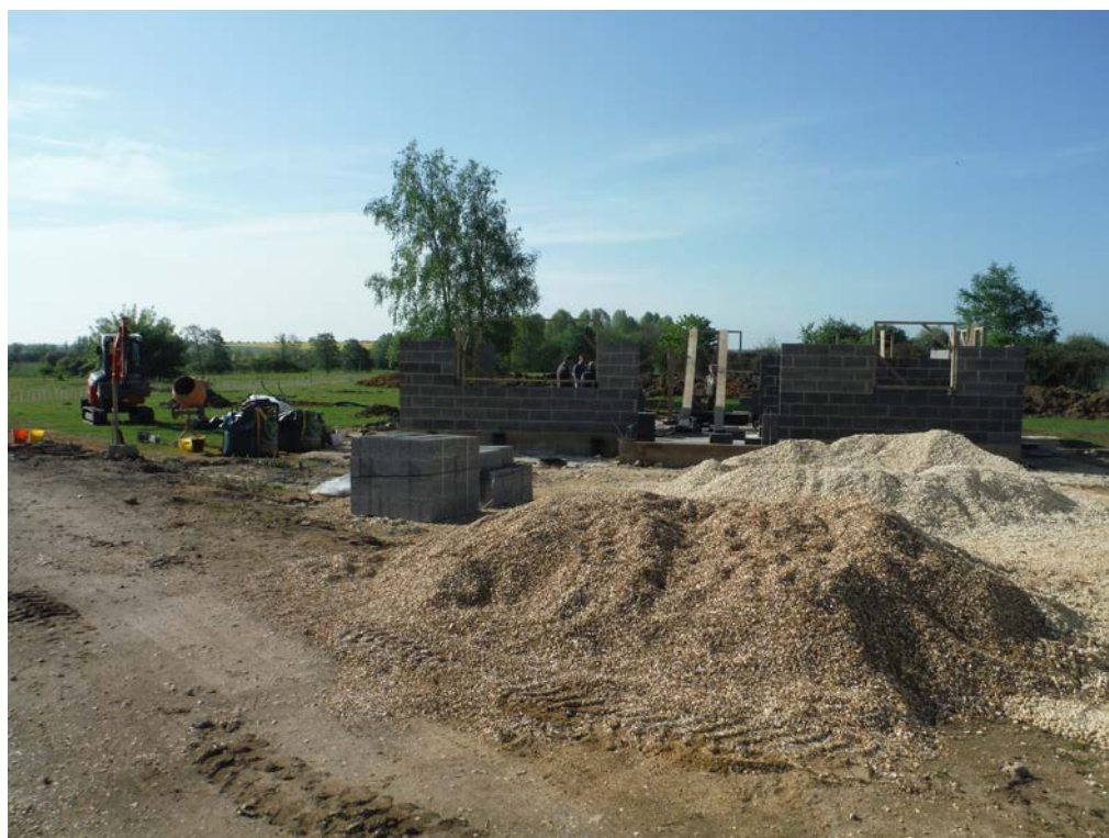
Plate 1: The site upon arrival, view south
