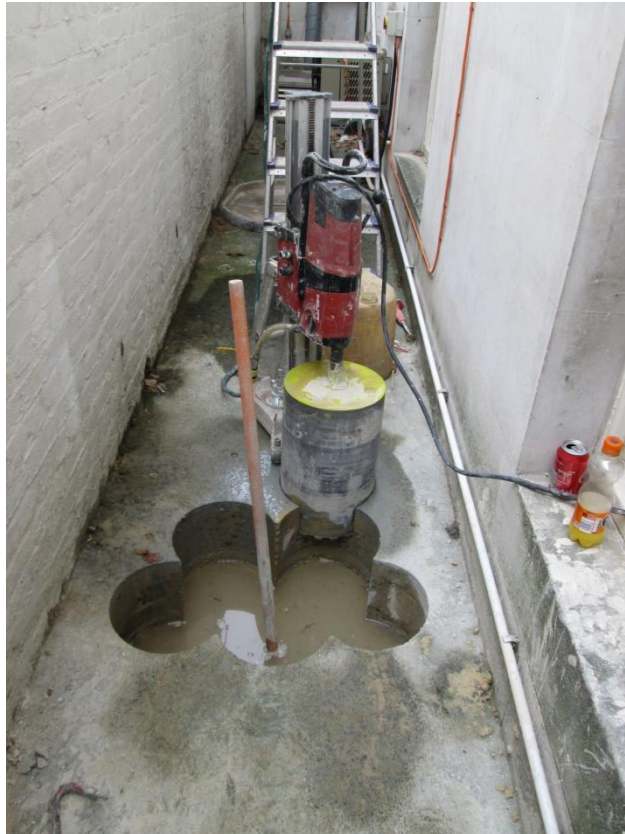
Plate 3: Test Pit 4 – concrete removal by corer, view to west
