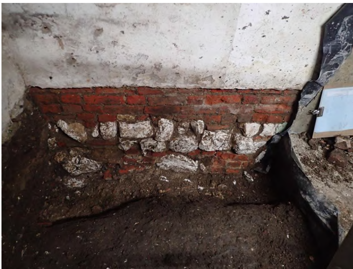
Plate 4: TR 2. South facing view of wall [11]
