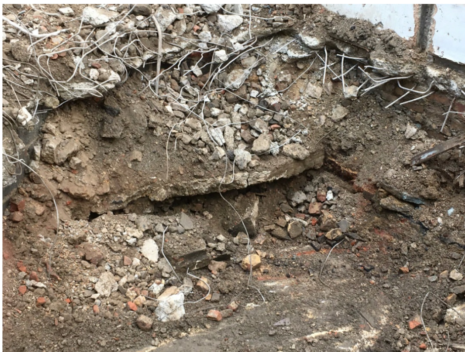
Plate 3: Basement level [18] overlain by made ground and concrete slab layers [1], [5], [9] and [10] during ground removal excavation
