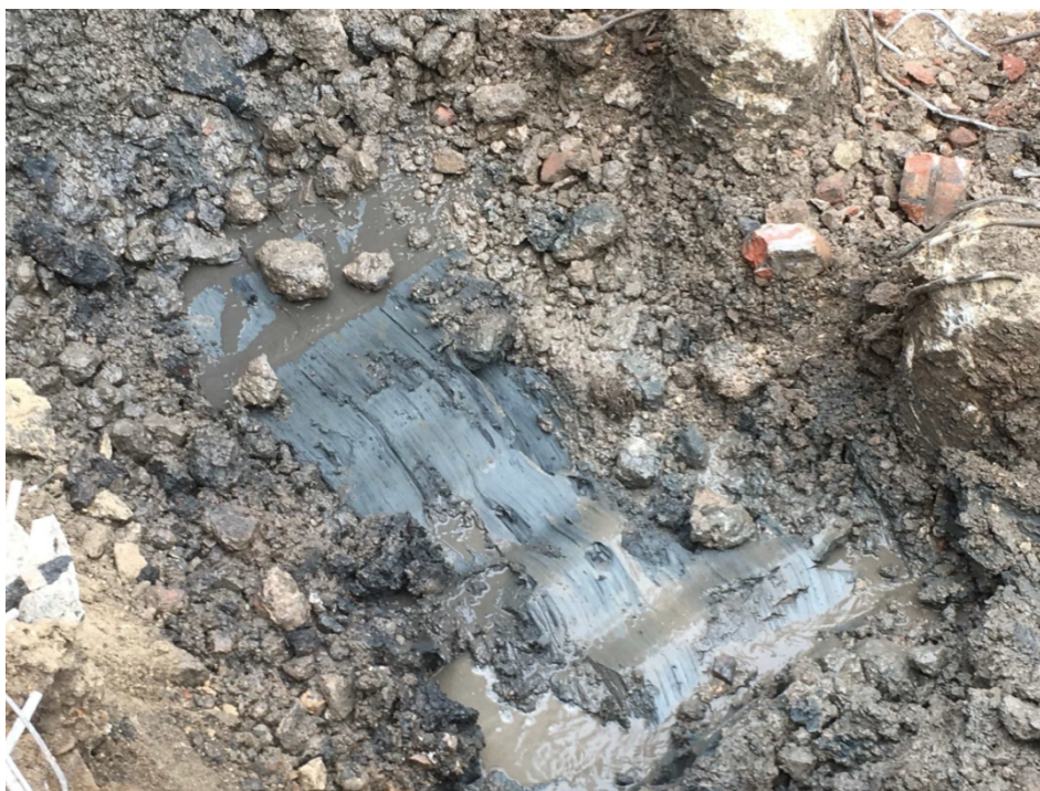
Plate 1: Alluvium layer [13] during ground reduction
