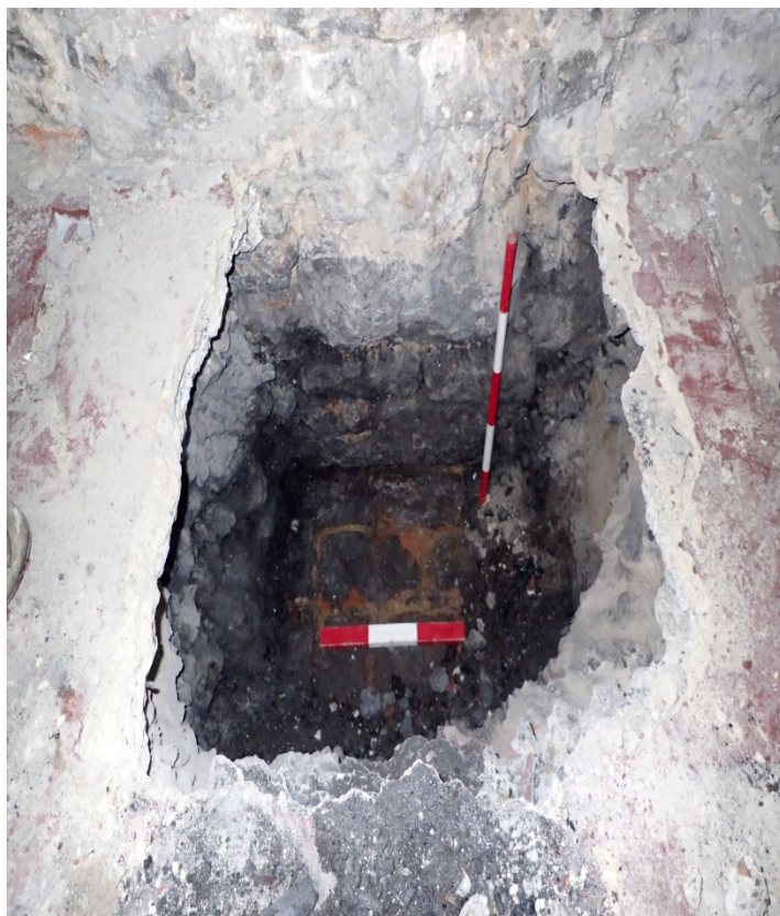
Plate 6: Test Pit 5, view to the north (scales 0.5m and 0.30m). The Great Kitchen wall [8] can be seen resting on the three regular courses of blocks [9] with the brick floor [10] inserted beneath them.
