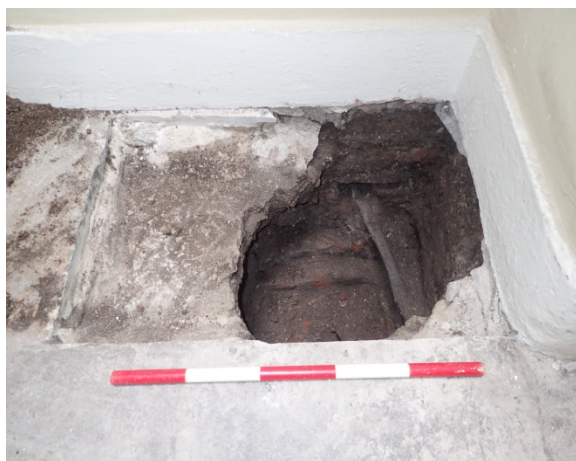
Plate 4a & 4b: Test Pit 4, view to the east (scales 0.5m & 0.3m). Plate 4a shows that the pit could only be partially opened due to a ceramic pipe in the northern half of the pit. A lead pipe is shown to the right of the pit. Plate 4b shows the red brick stepped foundations [24] below the north-south wall [23].
