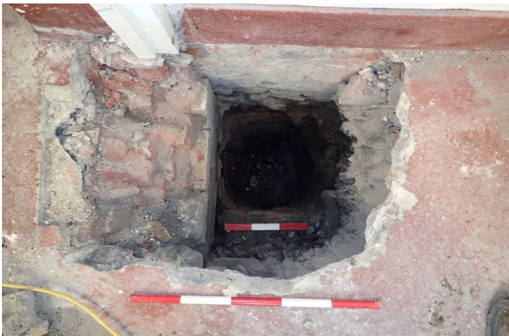
Plate 9: Test Pit 6, view to the south (scales 0.5m and 0.30m). The internal dividing wall [15] is to the left of the picture built upon the brick floor [16]. East-west wall [18] is visible at the top of the picture; regular brick courses become rougher 'mixed' stone towards its base. The 0.3m scale rests on brick floor [16].
