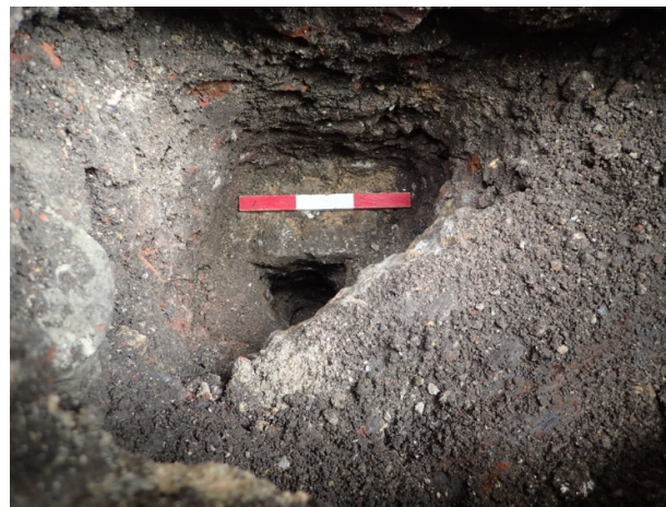
Plate 1a & 1b: Test Pit 1, view to the north. Plate 1a shows modern concrete footing [1] (0.5m scale) with earlier, stone-built footing [3] below it (0.3m scale). Plate 1b shows detail of footing [3] with squared, limestone blocks along with chalk and Reigate stone fragments set in a dark yellow mortar (scale 0.3m).
