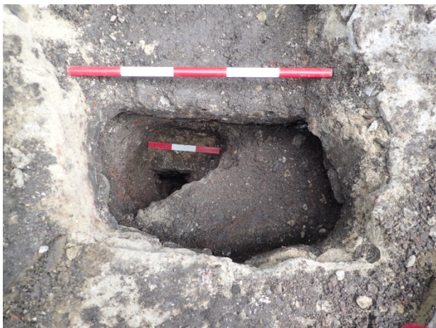
Plate 1a & 1b: Test Pit 1, view to the north. Plate 1a shows modern concrete footing [1] (0.5m scale) with earlier, stone-built footing [3] below it (0.3m scale). Plate 1b shows detail of footing [3] with squared, limestone blocks along with chalk and Reigate stone fragments set in a dark yellow mortar (scale 0.3m).
