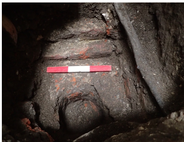
Plate 4a & 4b: Test Pit 4, view to the east (scales 0.5m & 0.3m). Plate 4a shows that the pit could only be partially opened due to a ceramic pipe in the northern half of the pit. A lead pipe is shown to the right of the pit. Plate 4b shows the red brick stepped foundations [24] below the north-south wall [23].
