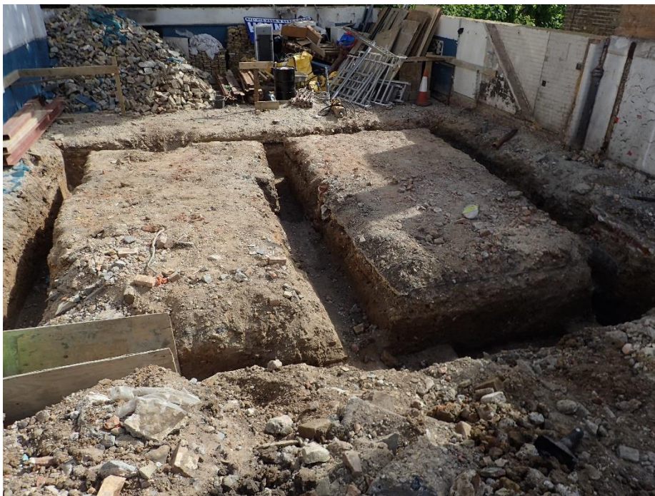
Plate 2: Foundation trenches, looking south-south-west
