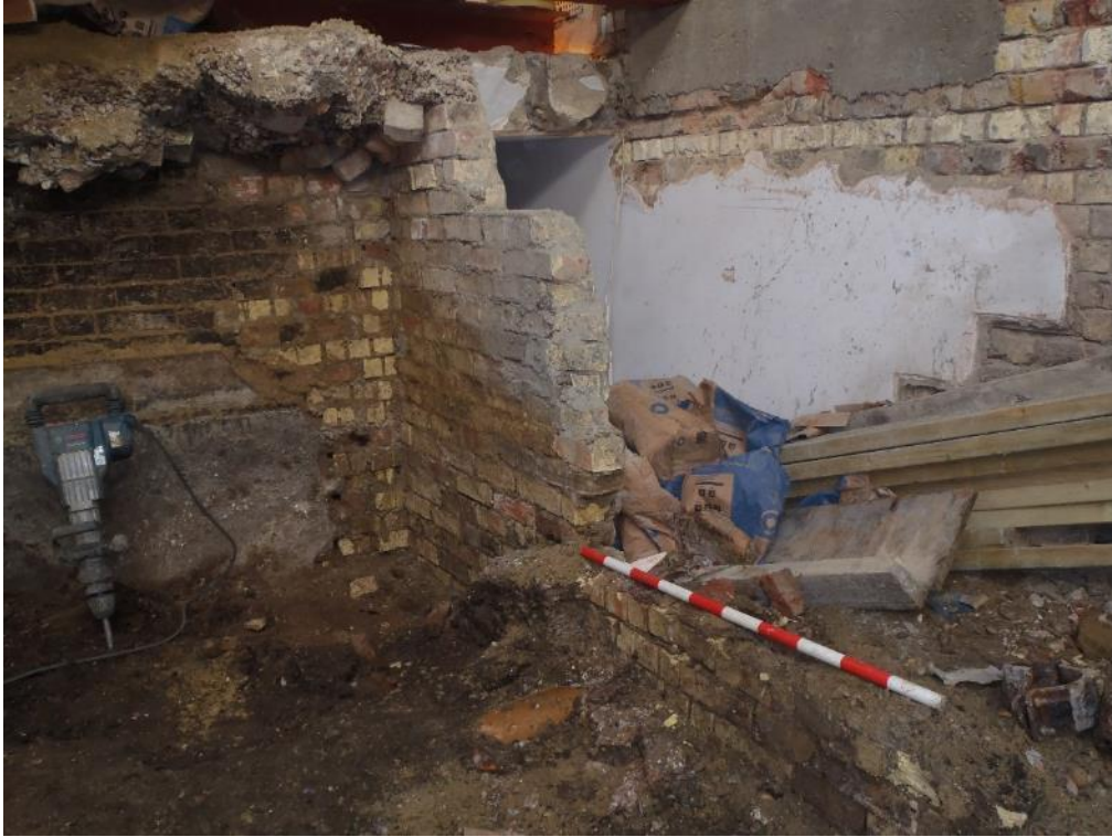
Plate 1: Wall [201] addition to earlier wall [125]. Facing south.
