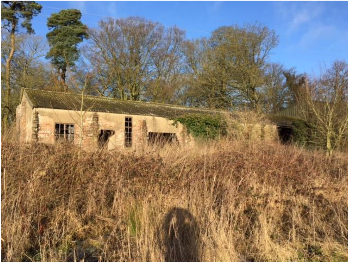
Plate A: Eastern elevation looking west (photograph provided by the Client)
