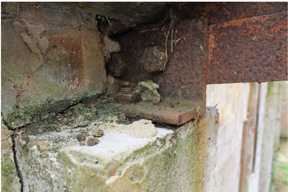
Plate 23 Bolted connection between pilaster and truss via L bracket
