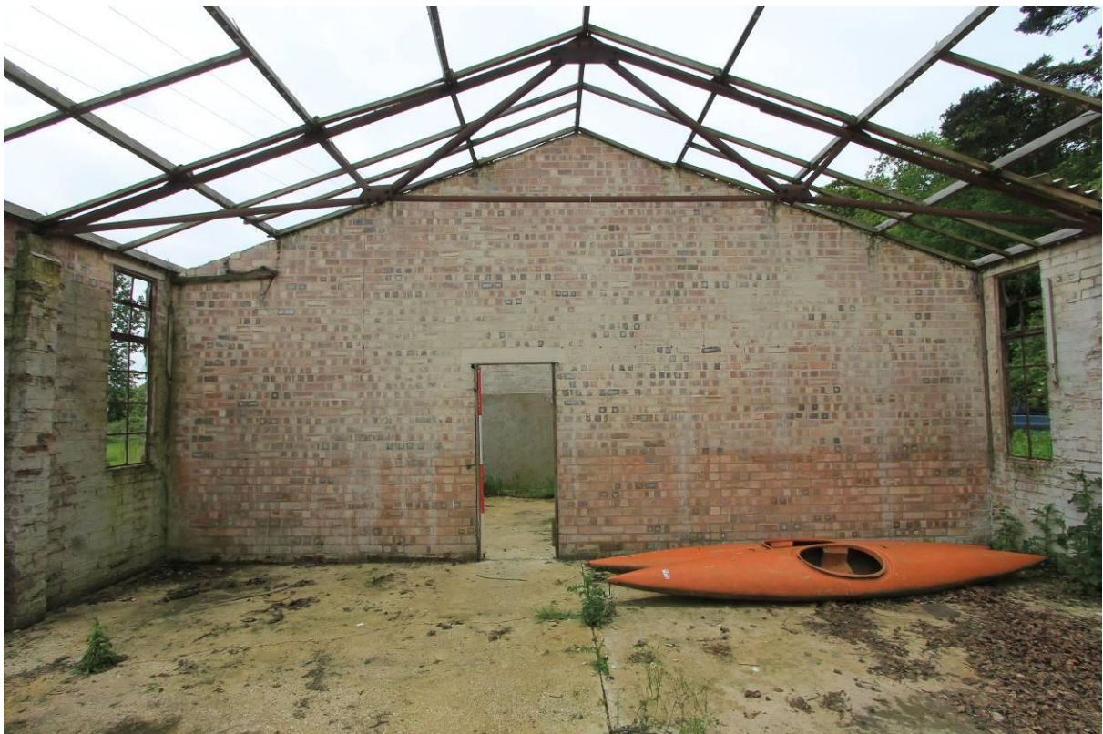
Plate 17 Internal dividing wall looking south
