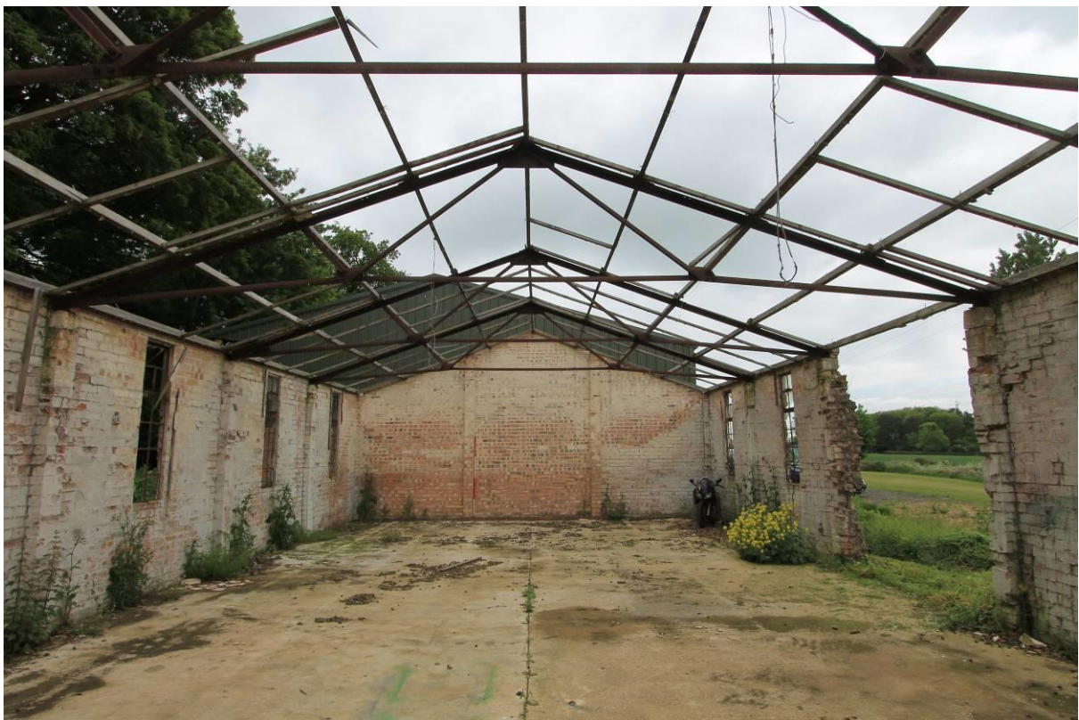
Plate 15 Interior (bays 3-9) looking north
