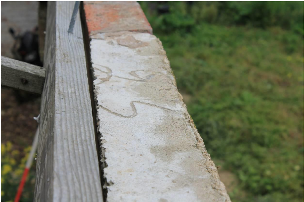
Plate 13 Batch/building number '25' scribed into top of window lintel
