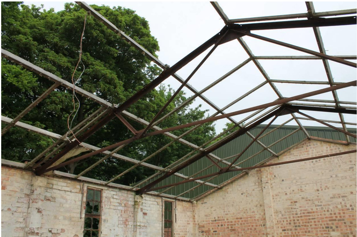
Plate 21 Triangulating truss looking north-west
