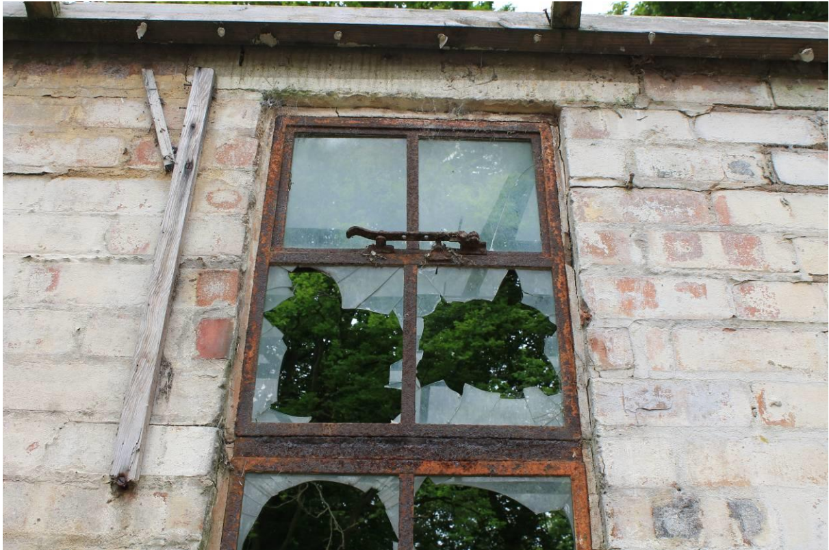
Plate 10 Upper (hopper) window and plain window stay (internal)
