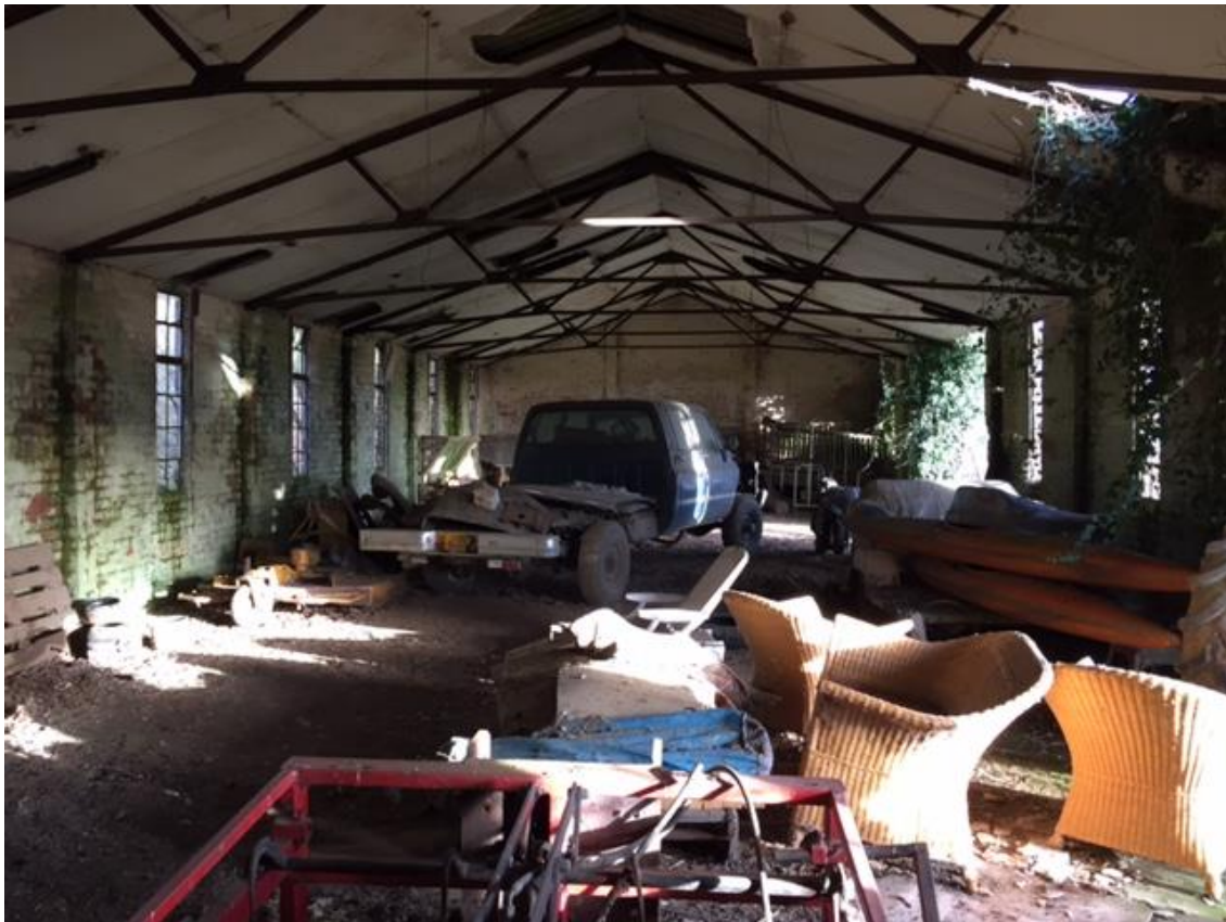
Plate B: Interior looking north (photograph provided by the Client)
