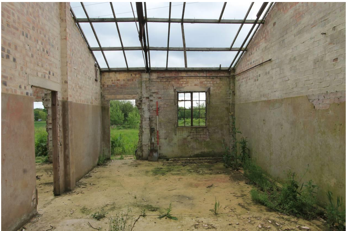
Plate 19 Bays 1-2 looking east
