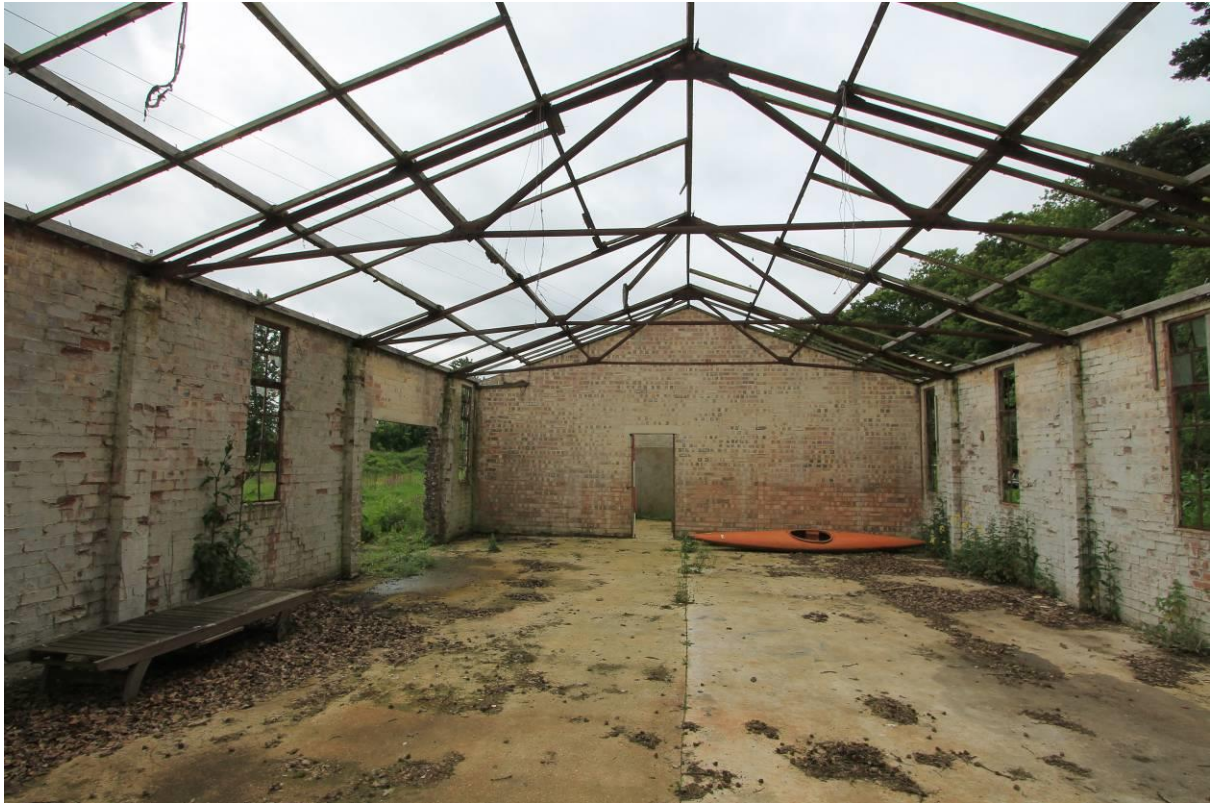
Plate 16 Interior (bays 8-3) looking south
