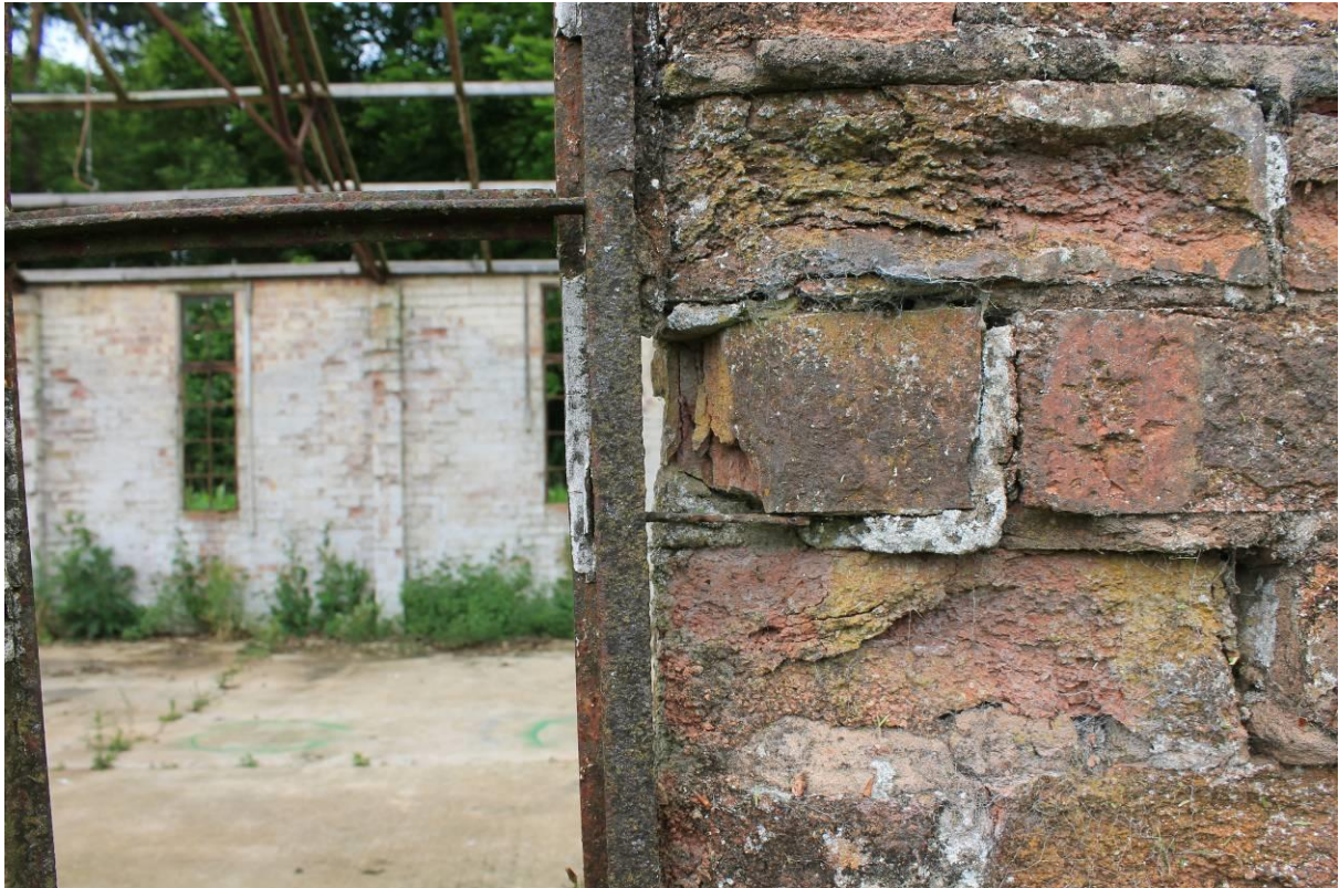
Plate 12 Integral metal tie built into brickwork
