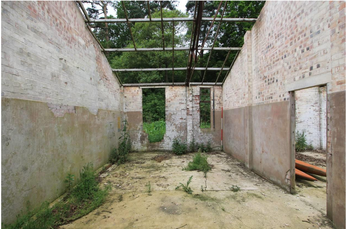
Plate 18 Bays 1-2 looking west, showing internal render
