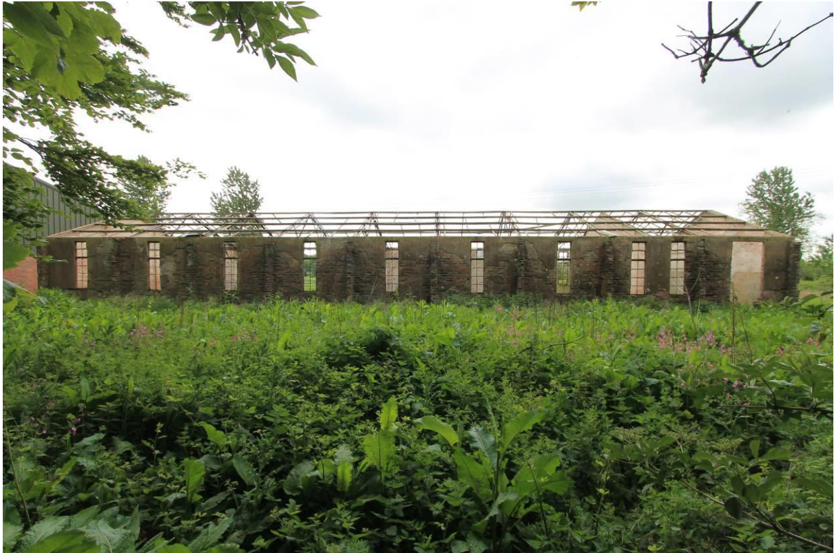
Plate 3 Western elevation looking east
