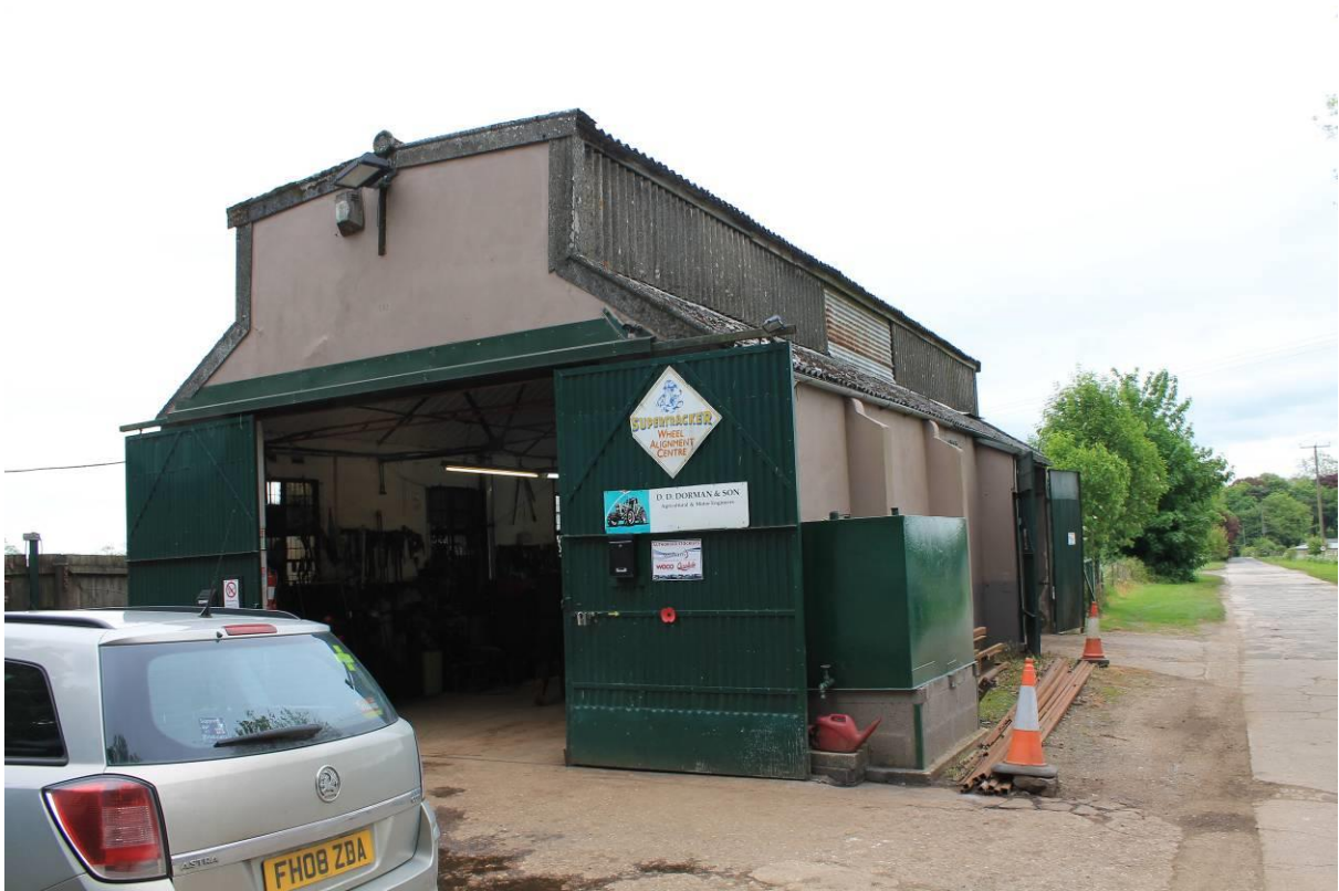
Plate 25 Former parachute shed (now car repair workshop) looking east
