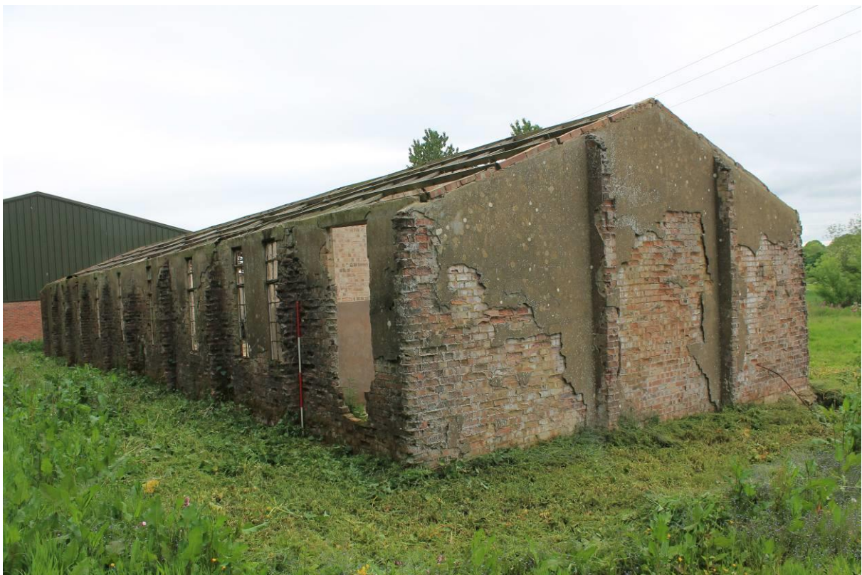
Plate 4 Western elevation looking north-east
