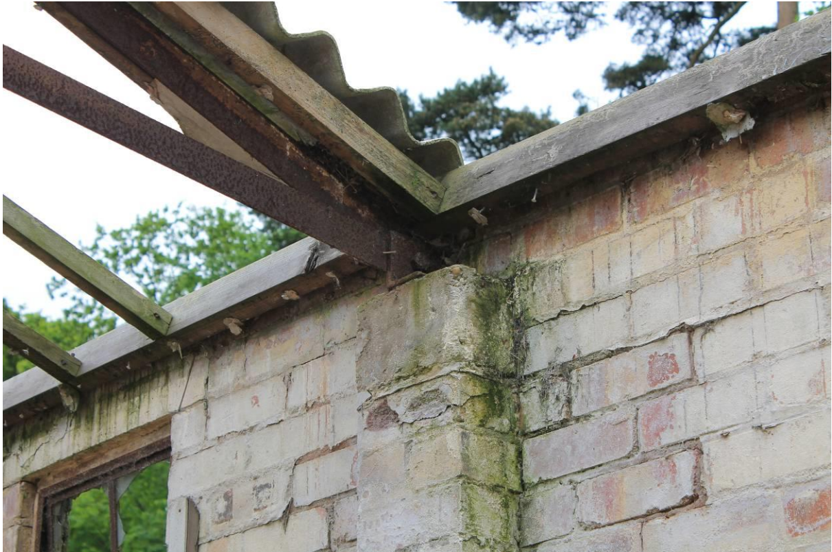
Plate 22 Concrete pad on top of pilaster
