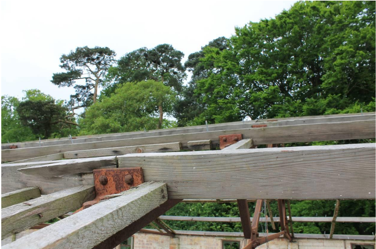
Plate 24 Brackets supporting softwood purlins
