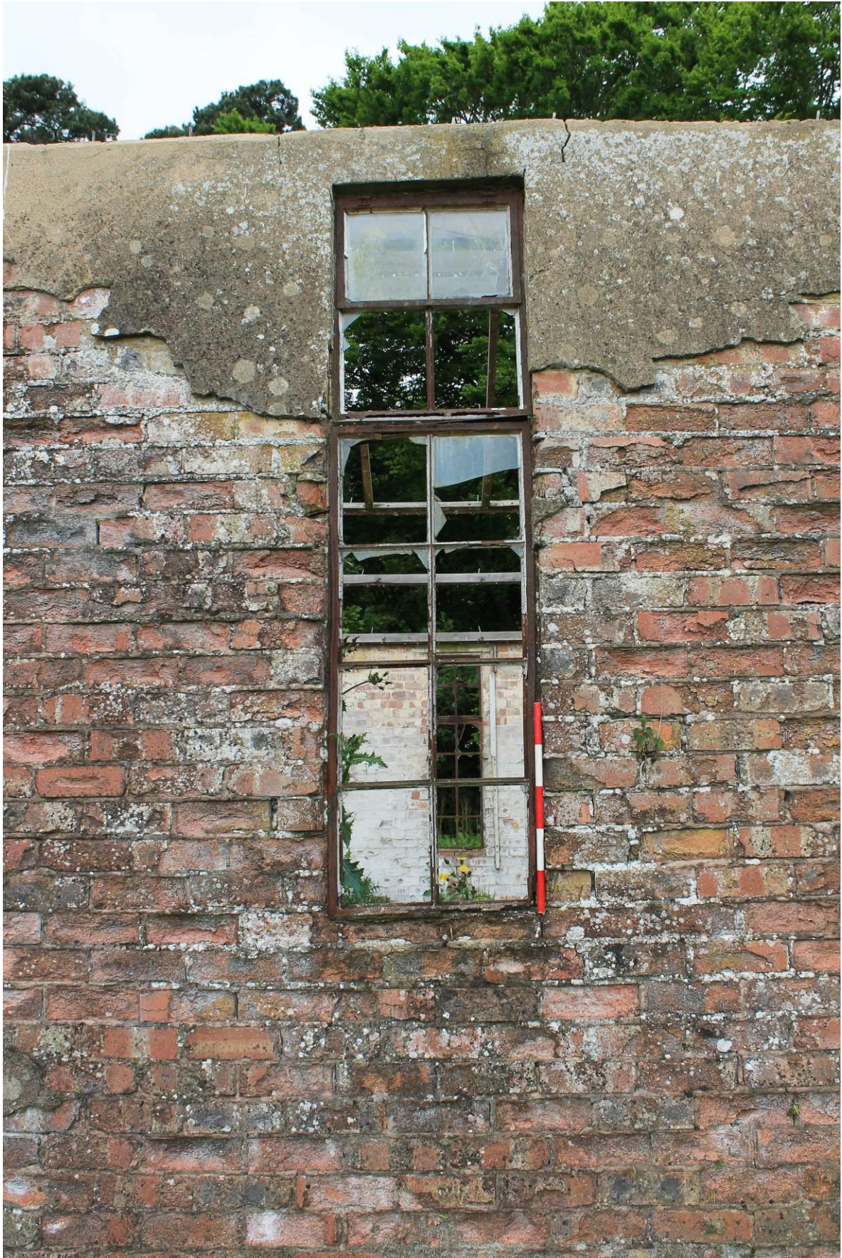
Plate 9 Typical tall window (external), looking west
