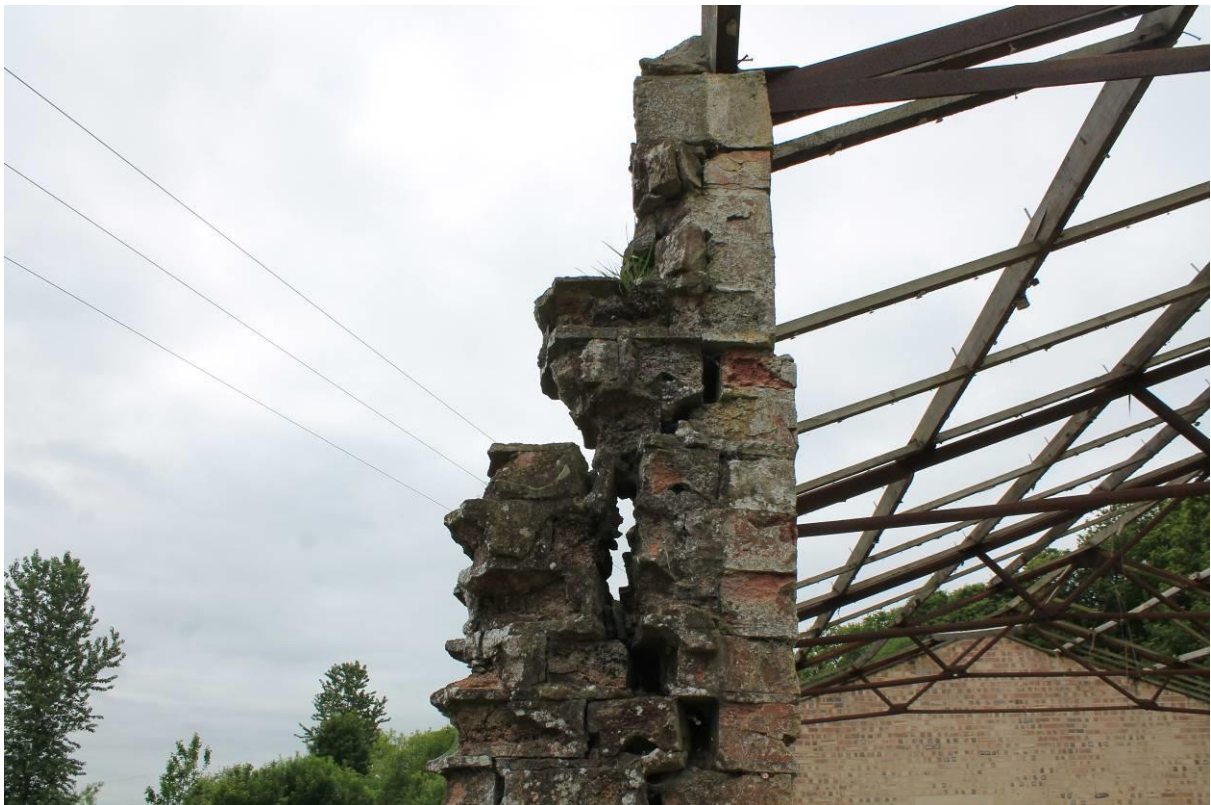
Plate 8 Spalled and detaching brickwork (bay 6) looking south
