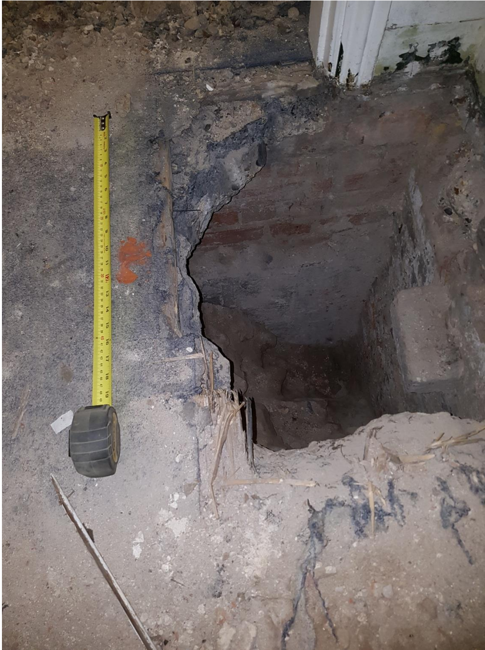
Plate 14 Brick walls and possible concrete foundation Geotechnical Pit 3 Scale 0.50m
