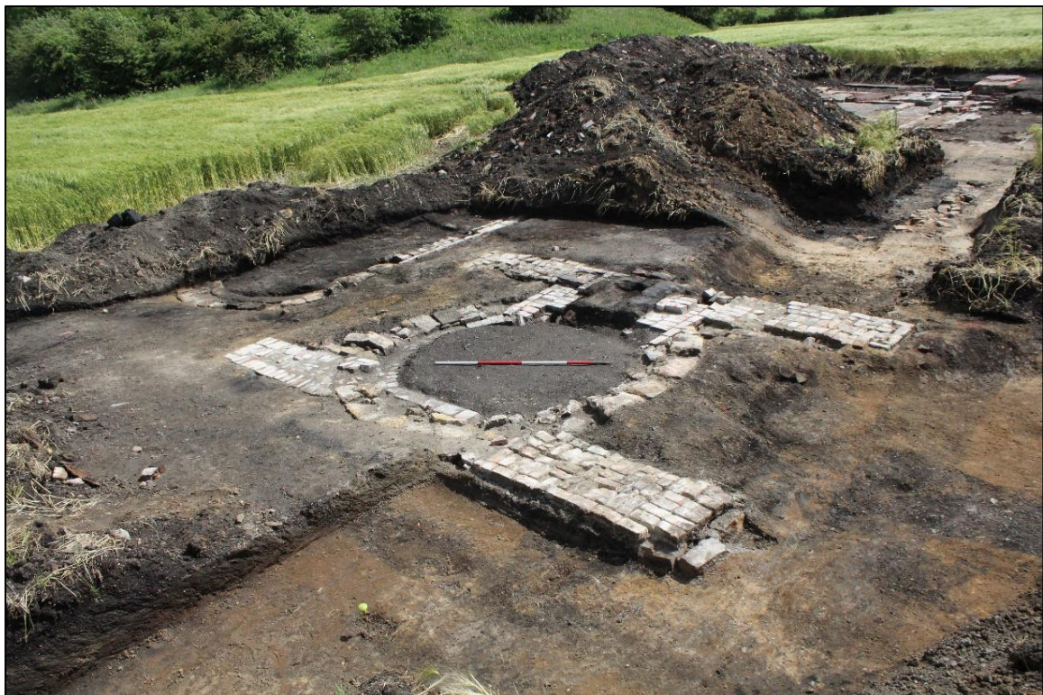
Plate 6. Trench 21, pithead structures including shaft [2131] within northern extension, looking south-east, 2m scale
