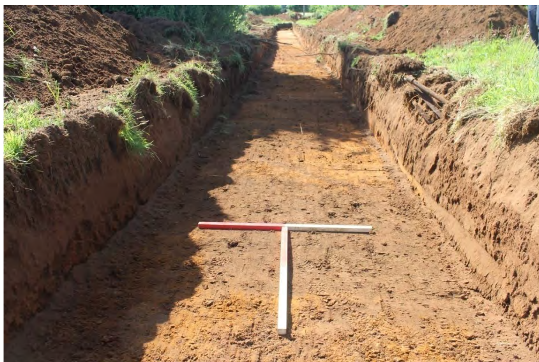
Plate 17: Trench 7, view south
