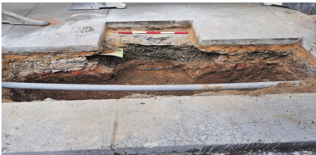
Plate 1: Trial Hole TH01 on St James's Street, view to the south-west with road kerb in the foreground. The grey plastic ducting and a black service cable can be seen. Underneath the modern concrete a layer of fragmentary brick [1] had been laid on compacted made ground [2]. Scale 0.5m
