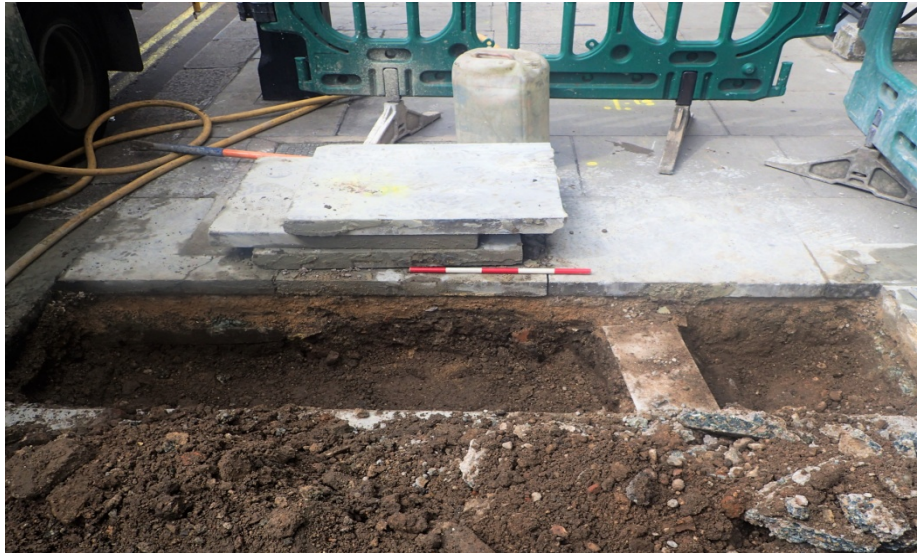
Plate 6: TH3:B3 view to the south-west, roadside kerb on the left of the photograph. The slab can be seen to the left of the photo directly below the bedding layer. To the right a steel plate protects live services. Scale 0.50m
