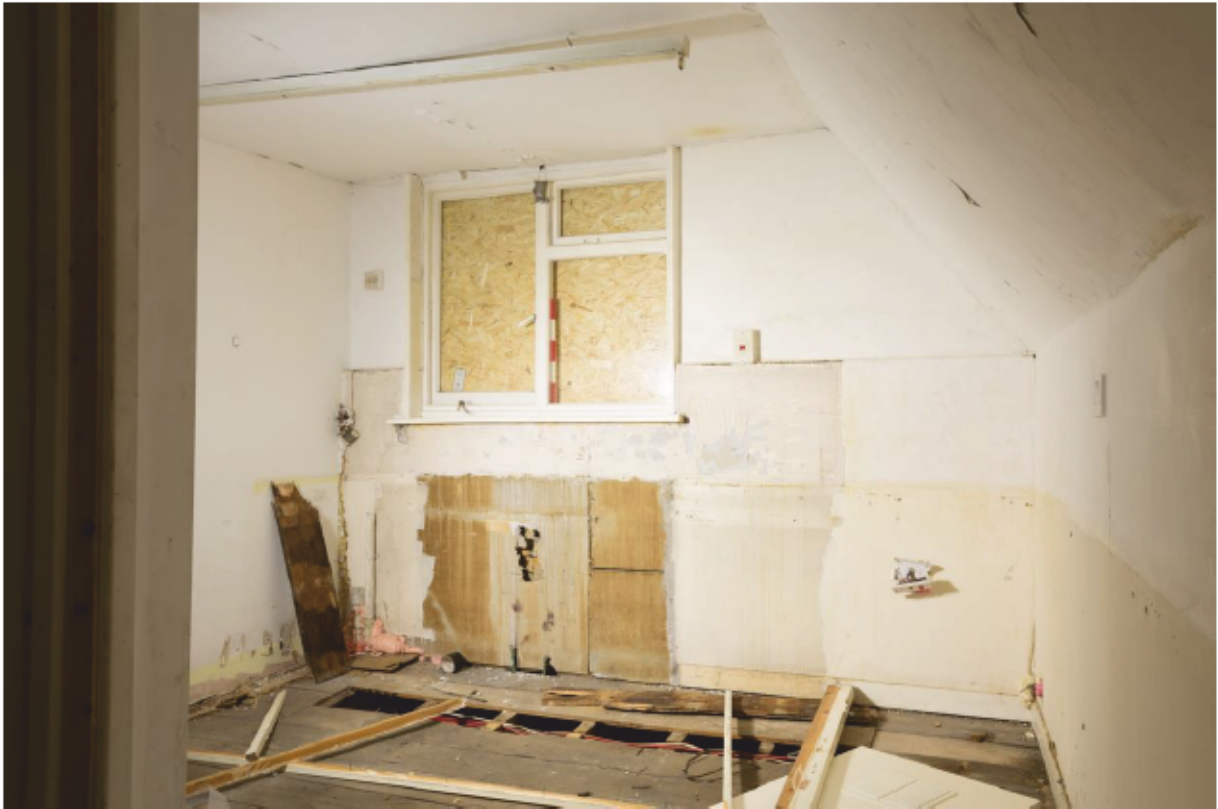
Plate 40 Former kitchen FF8
