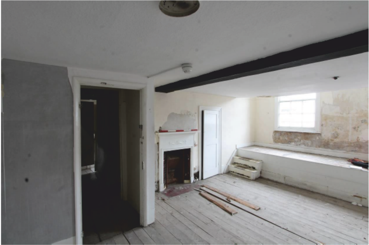
Plate 27 Room FF1 looking north-east
