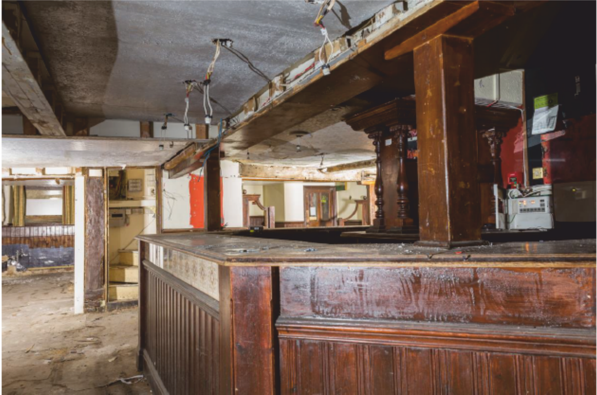
Plate 14 Bar counter, note winder stair and storey post (left).
