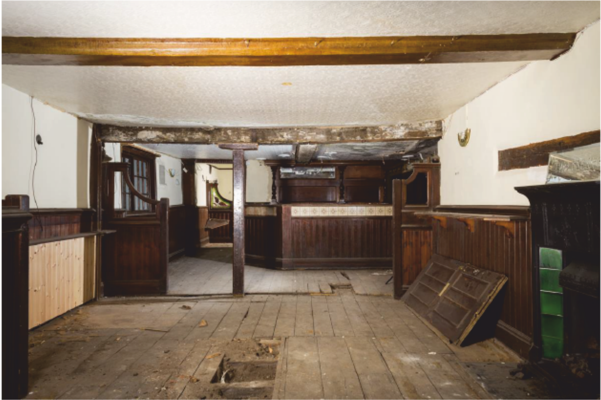
Plate 17 Bar, from GF1 to GF2, showing extant mid-rail (propped).
