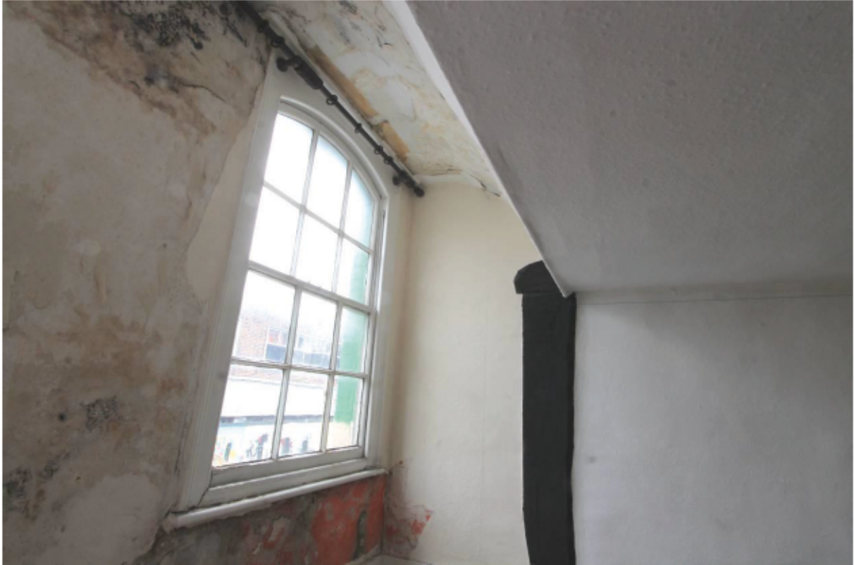
Plate 28 Storey post (FF1) in front main building and later Victorian re-fronting (showing higher windows)
