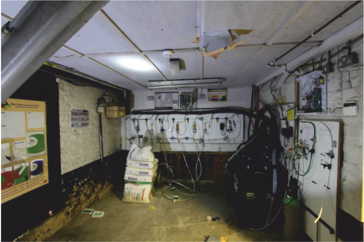
Plate 25 Beer Cellar (GF10)
