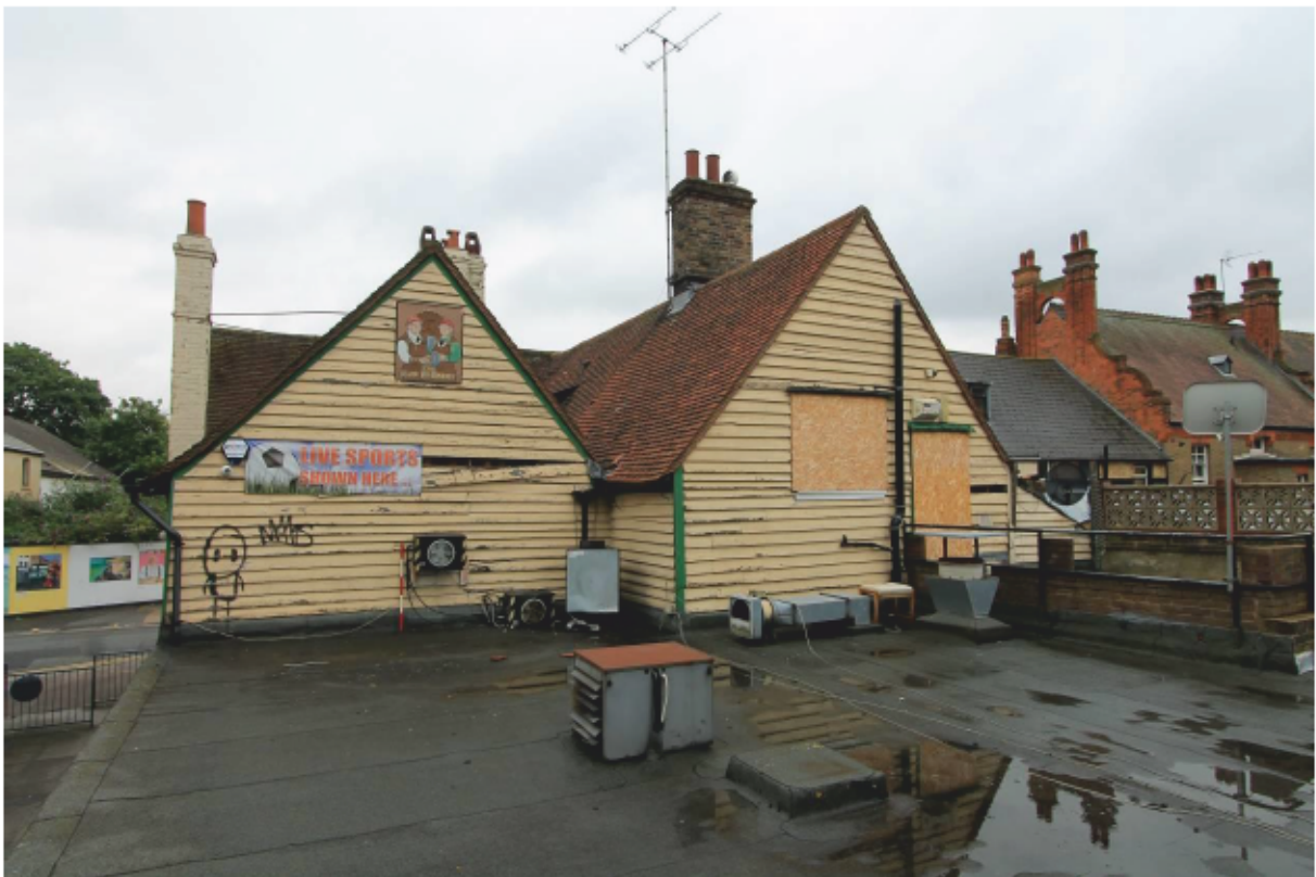
Plate 12 Northern and southern rear wings, looking east
