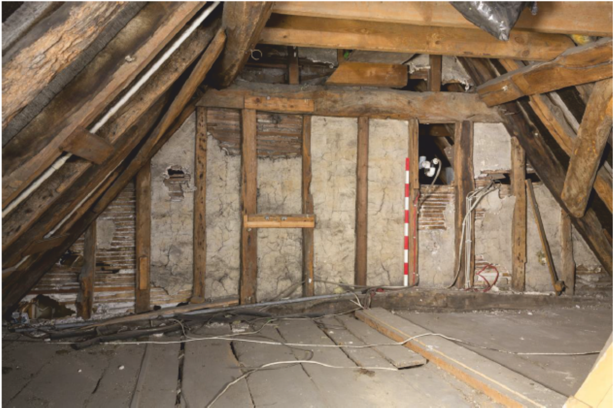
Plate 50 Lath and plaster panels (A4)
