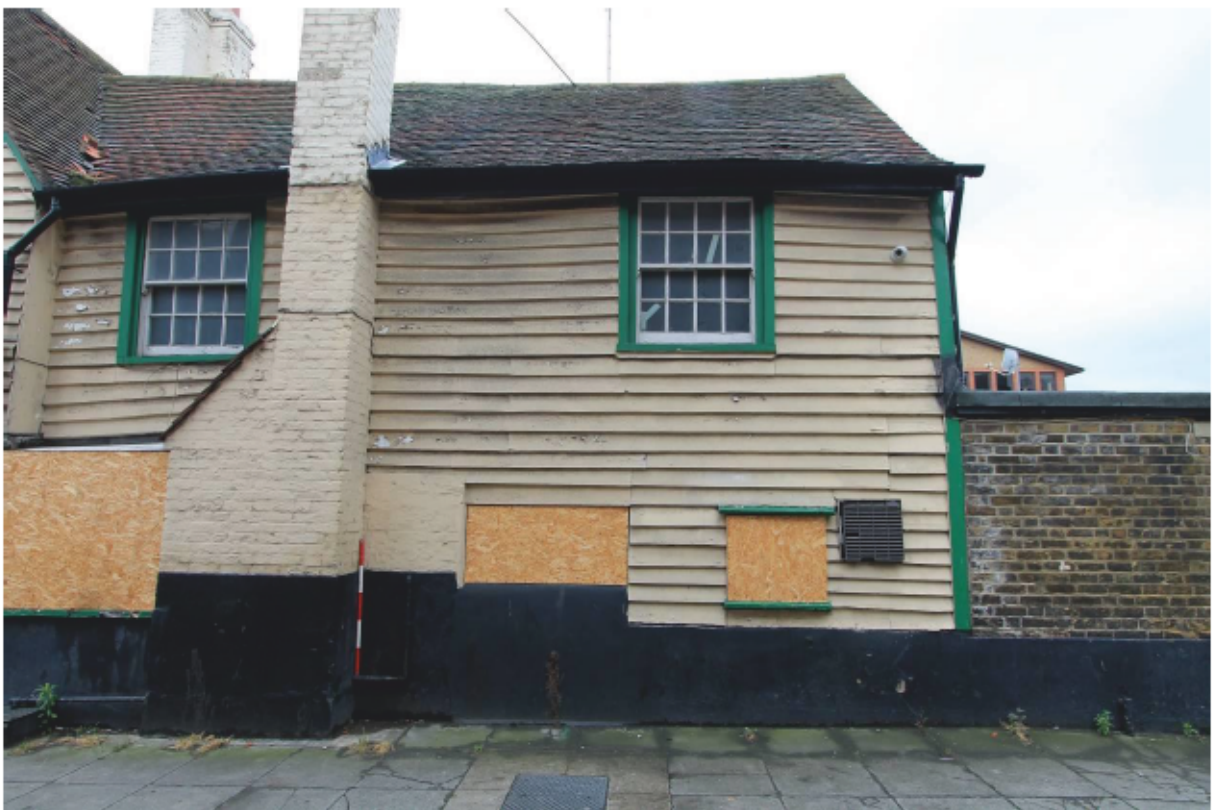
Plate 6 Northern elevation to rear north extension
