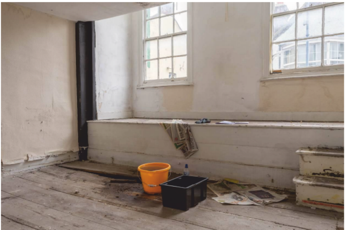
Plate 30 Room FF2 showing platform added to enclose heightened ground floor windows
