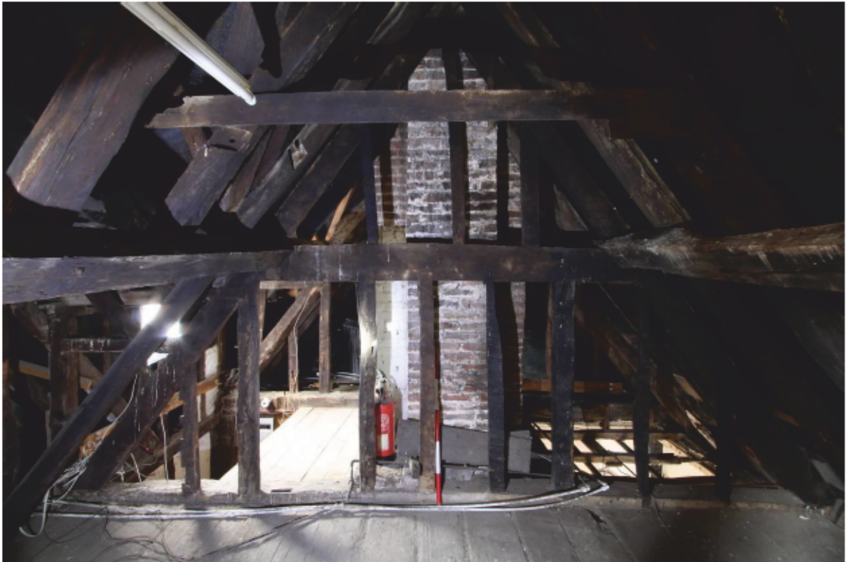
Plate 44 Attic (A1) looking north to central chimneystack
