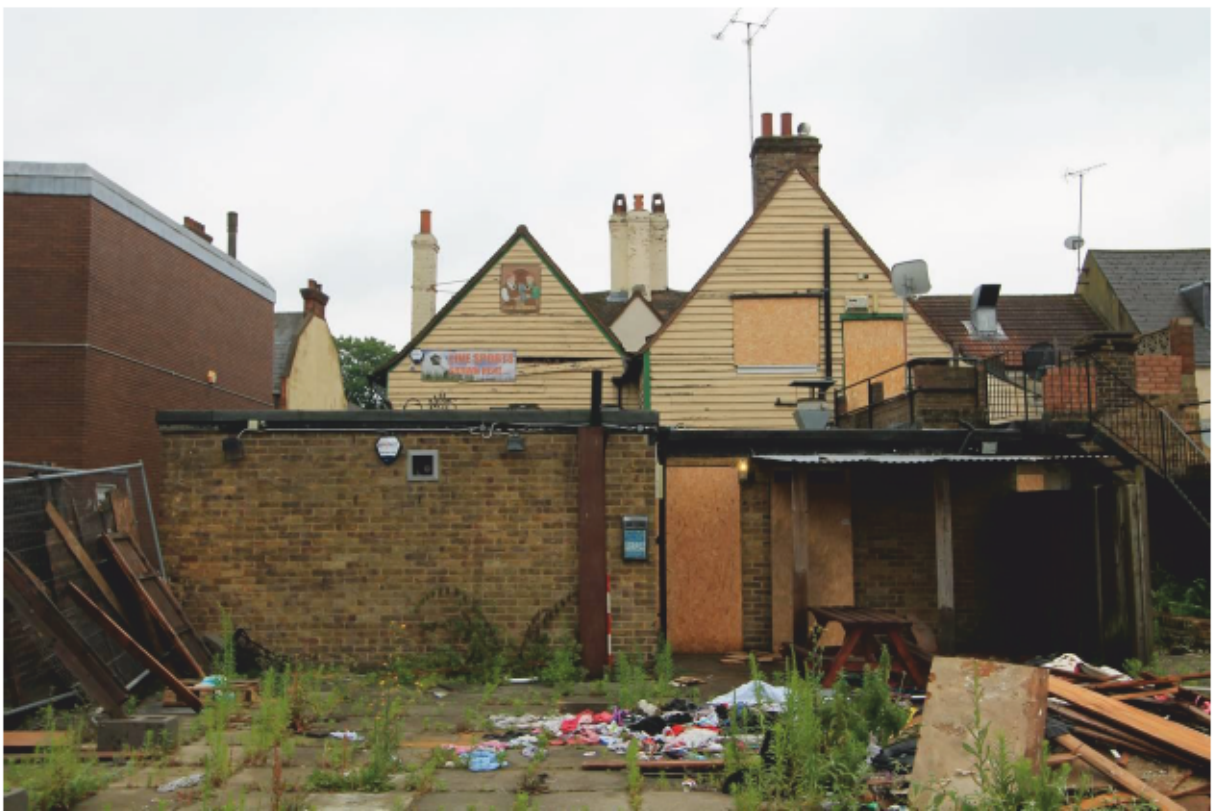
Plate 8 Rear elevations from rear yard
