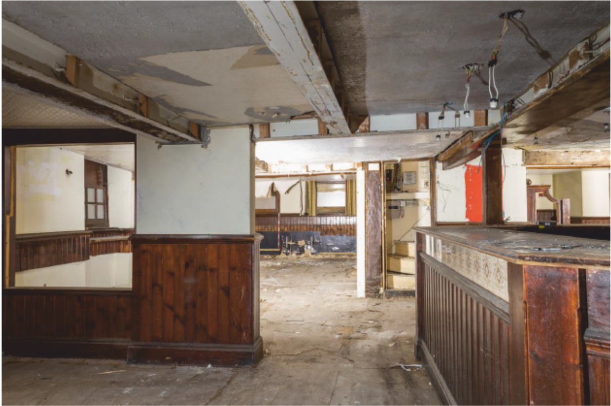
Plate 13 Bar, from GF5 towards GF3
