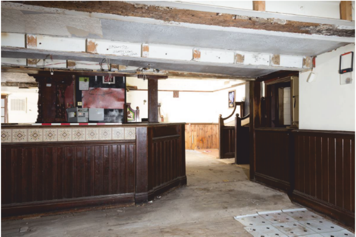
Plate 15 Bar, from GF5 to GF6
