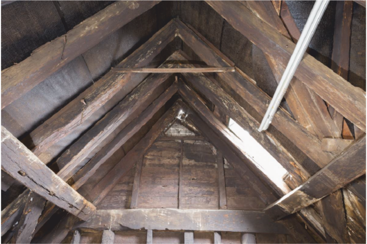
Plate 46 Pegged rafters (A1)
