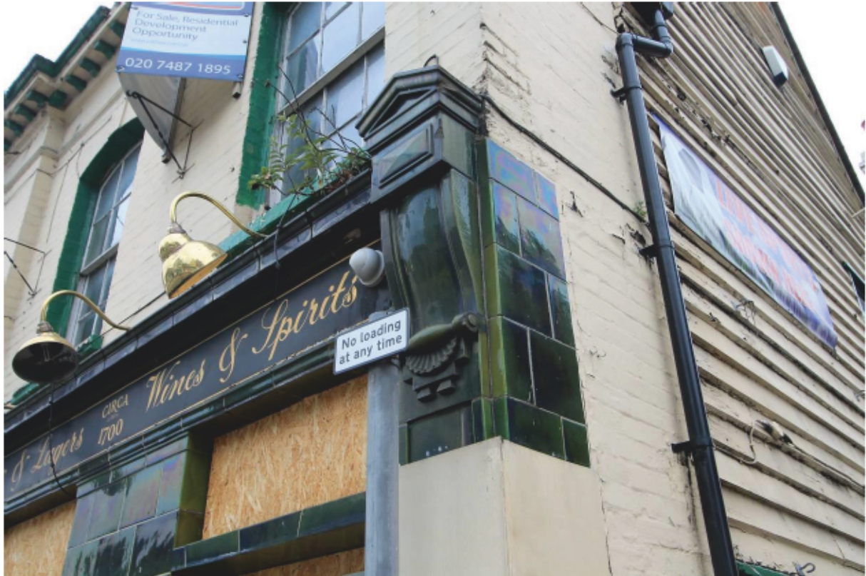
Plate 3 Decorative bracket to facade
