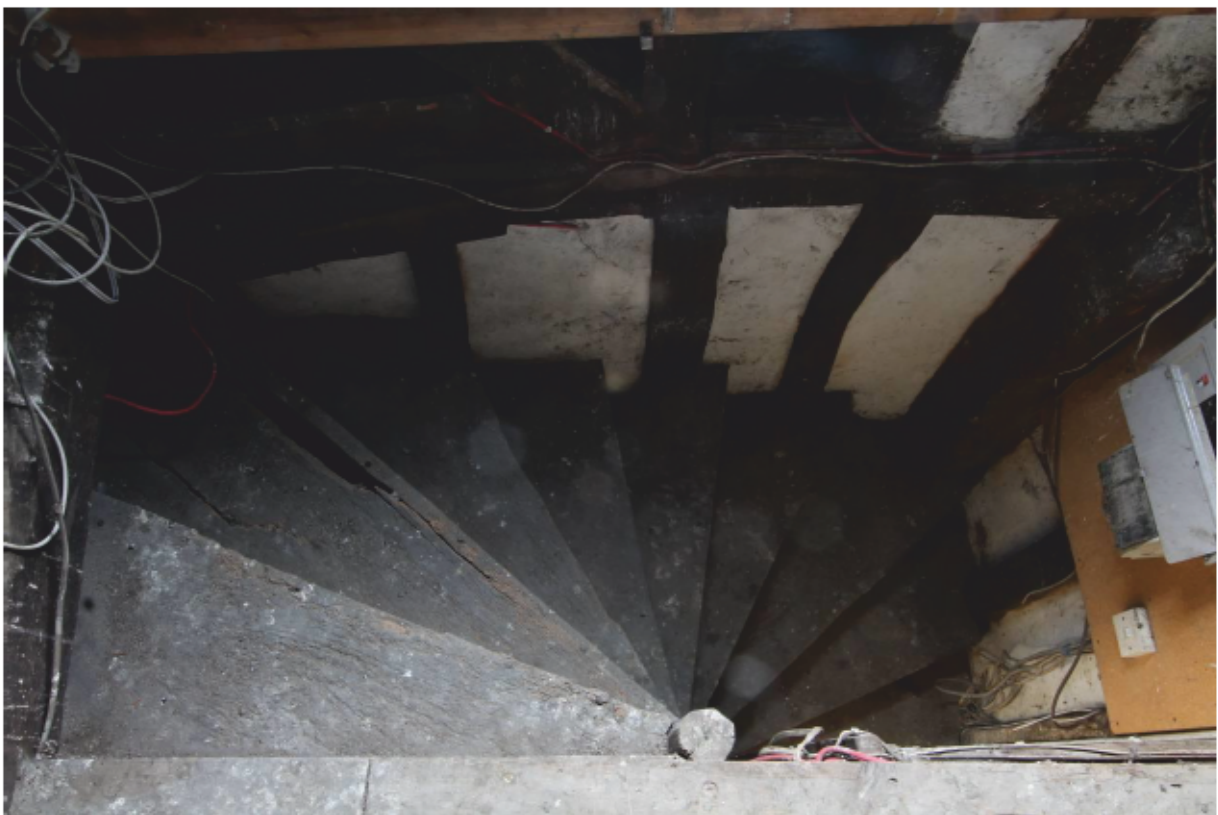
Plate 41 Winder stair to attic FF9
