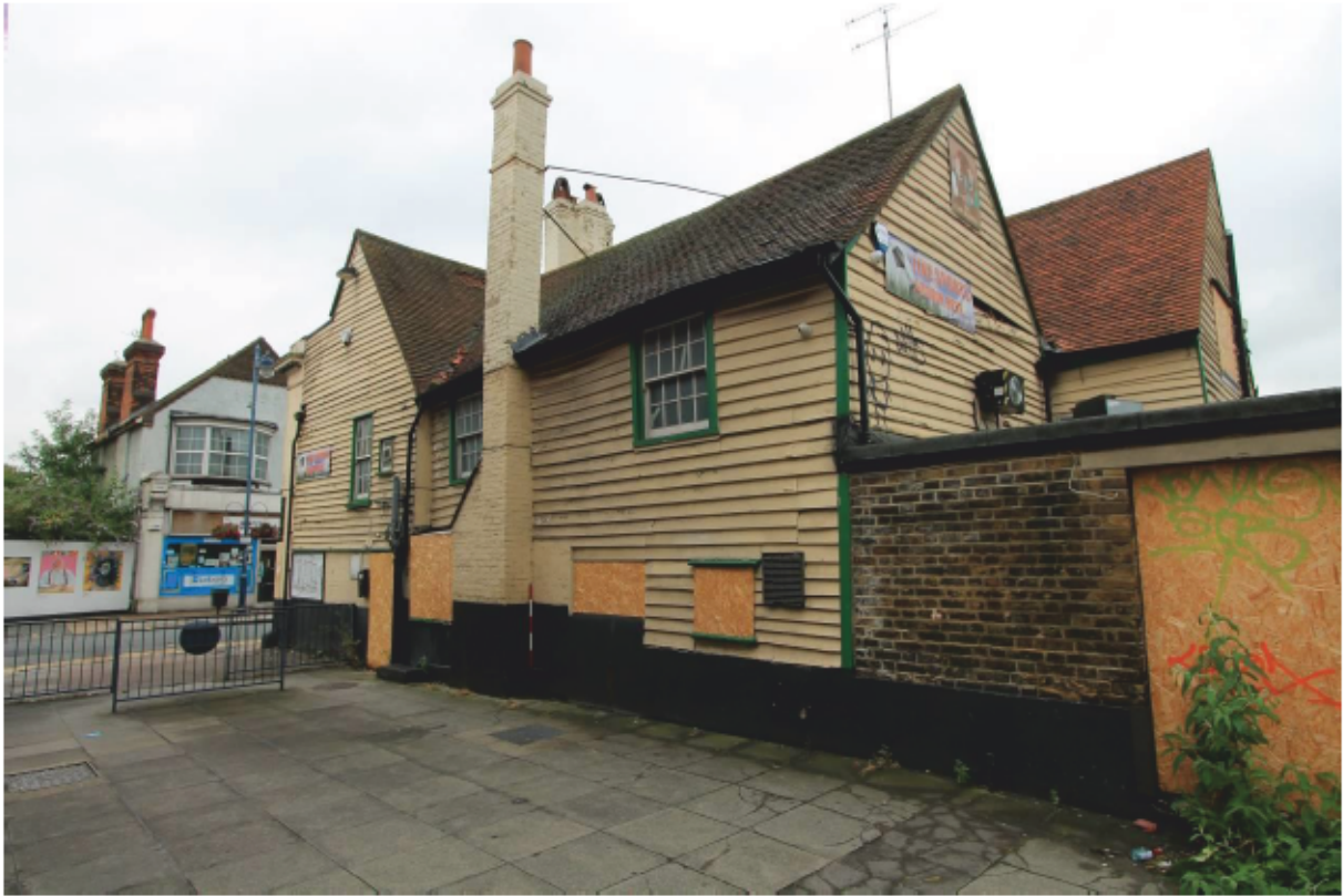
Plate 5 Northern elevation looking east
