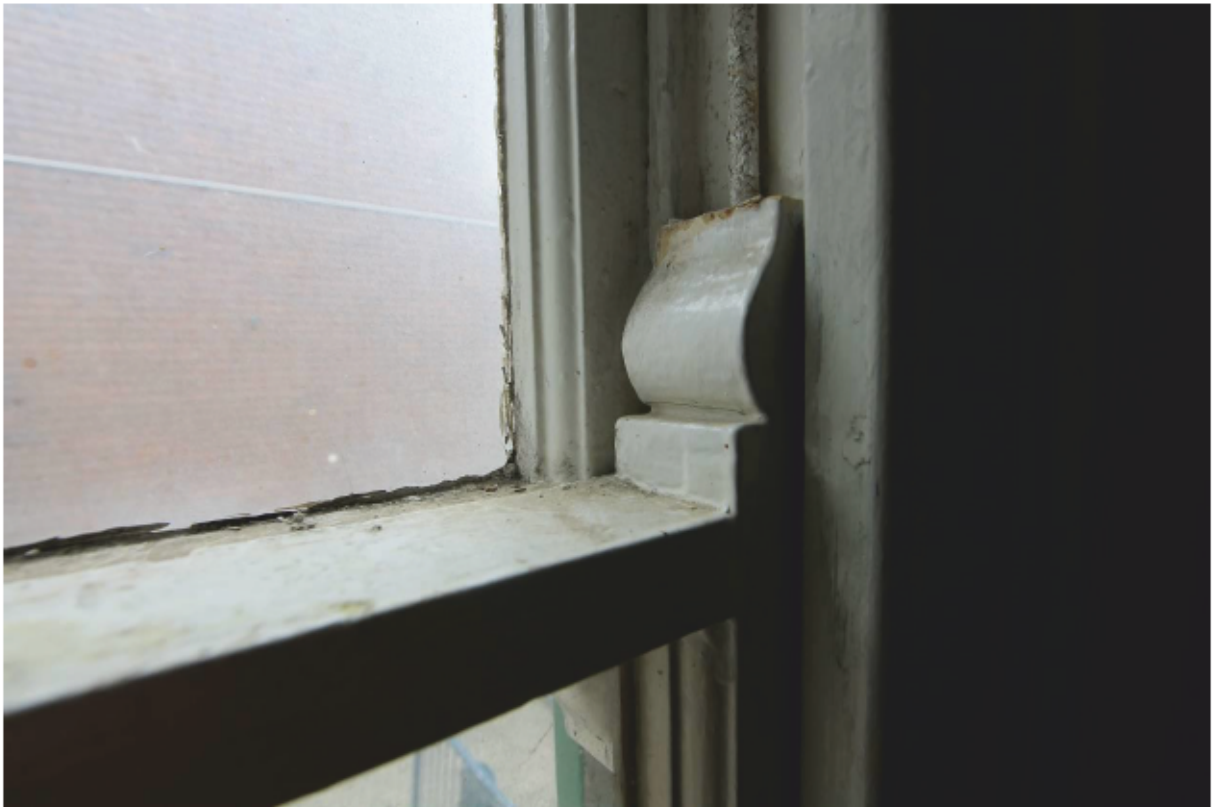
Plate 36 Detail of horned sash (FF5)
