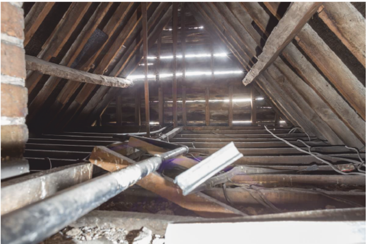
Plate 53 Roof over (A6) looking west
