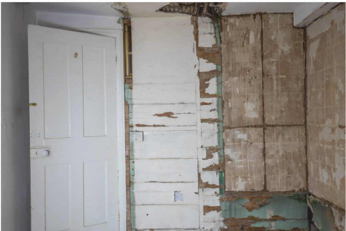
Plate 34 Matchboarding in FF3
