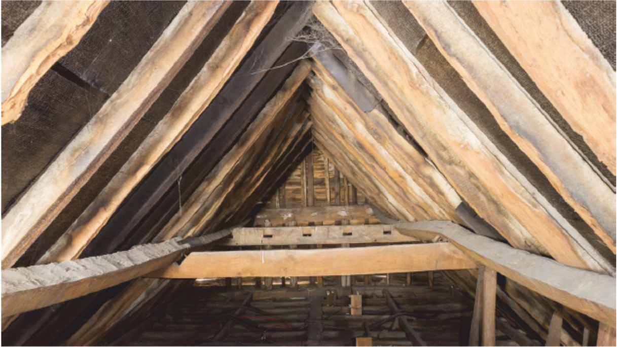
Plate 52 Roof over (A5) north rear extension, looking west
