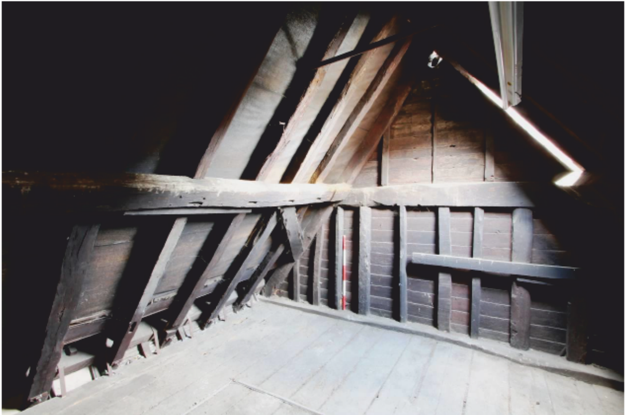
Plate 42 Attic (A1) looking south
