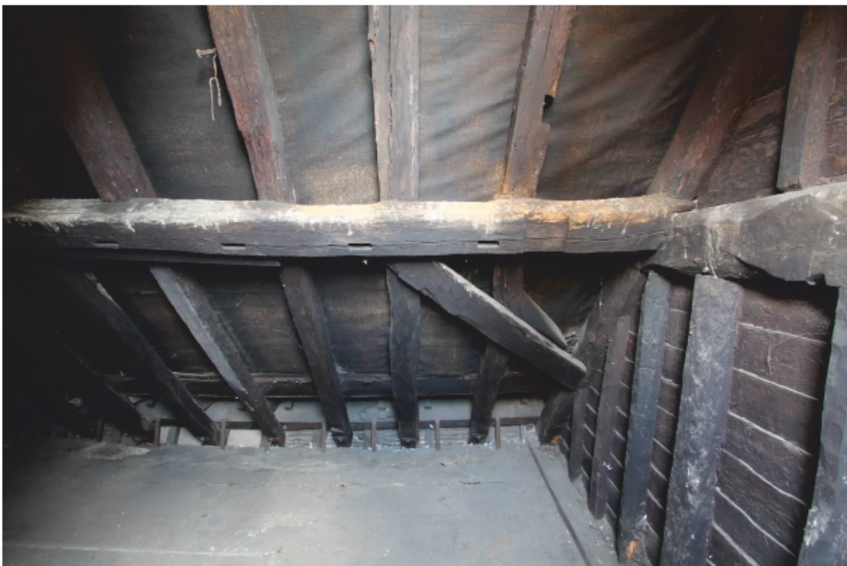
Plate 43 Attic (A1) windbrace
