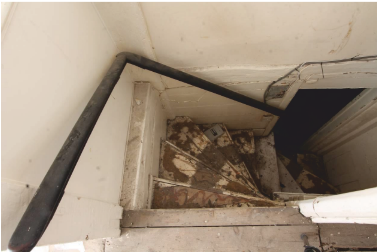
Plate 22 Winder stair (GF8) from first floor
