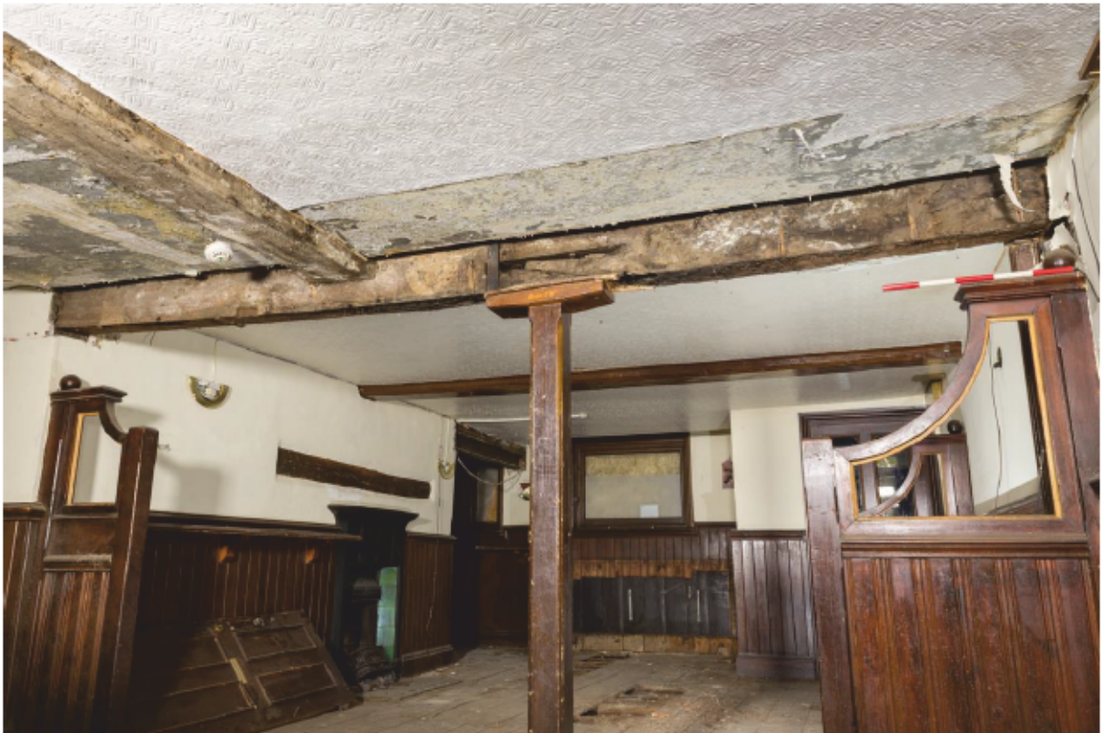
Plate 18 Mid-rail or girding beam and axial bridging joist from GF2
