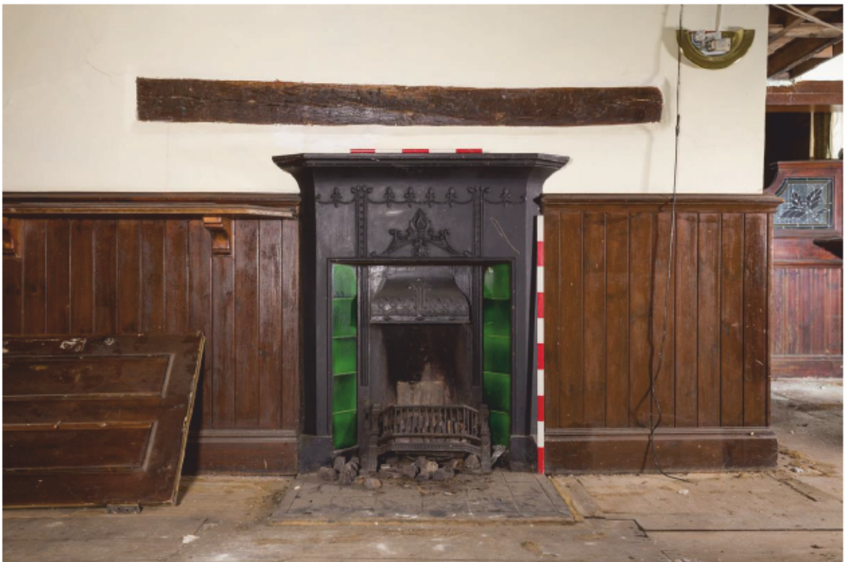
Plate 20 Victorian cast-iron fireplace in GF1
