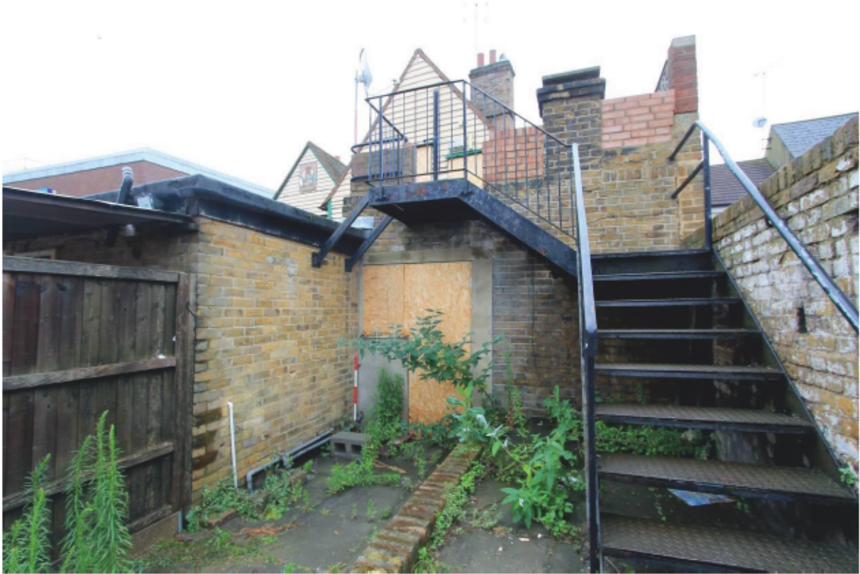
Plate 11 Modern extension and fire escape
