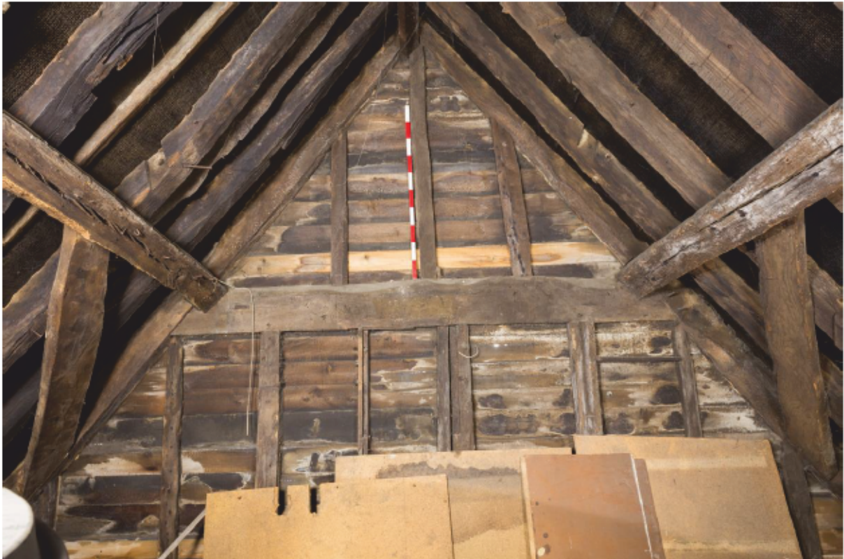
Plate 48 Attic (A3) looking north
