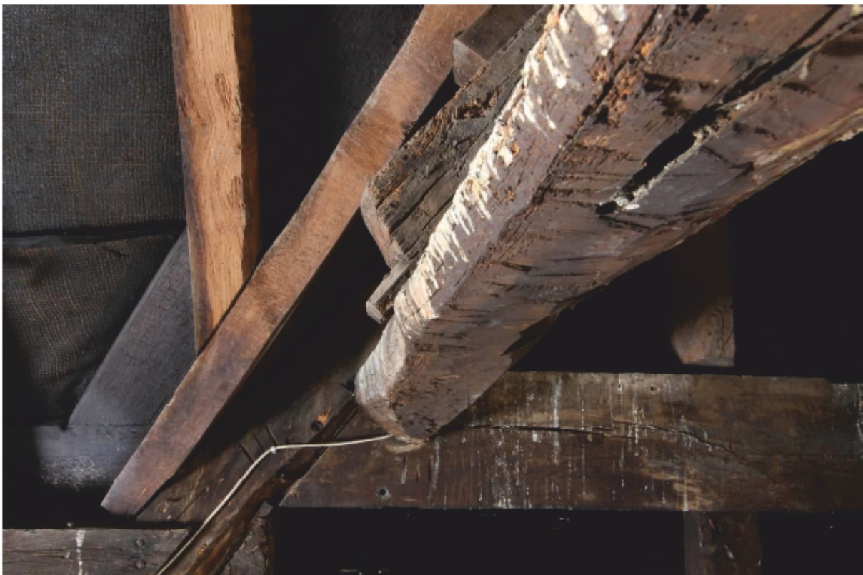
Plate 45 Attic (A2) cut away purlin and carpenters marks (III) on principal rafter and collar
