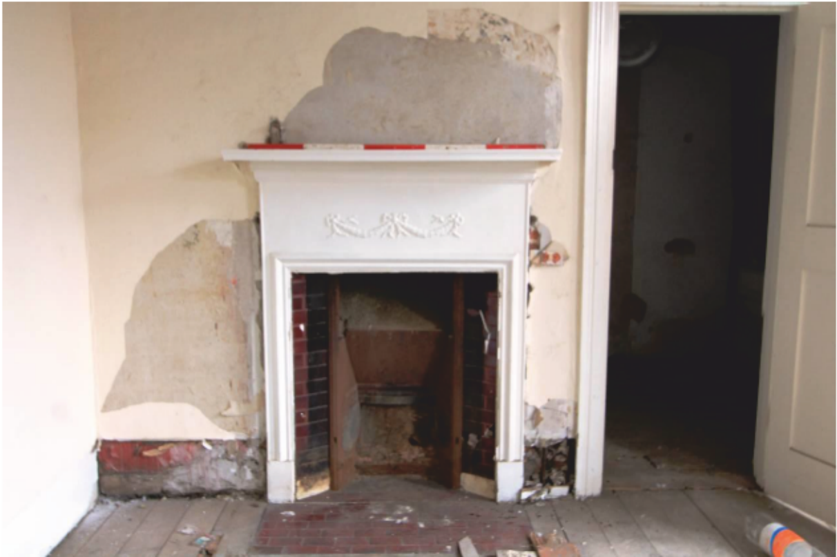
Plate 29 Detail of cast-iron fireplace (FF1)
