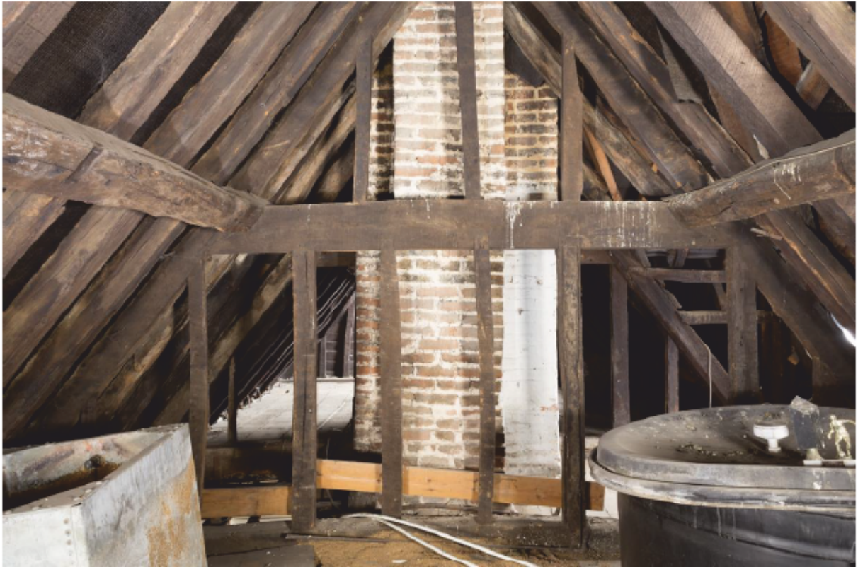
Plate 47 Attic (A3) looking south towards the chimneystack
