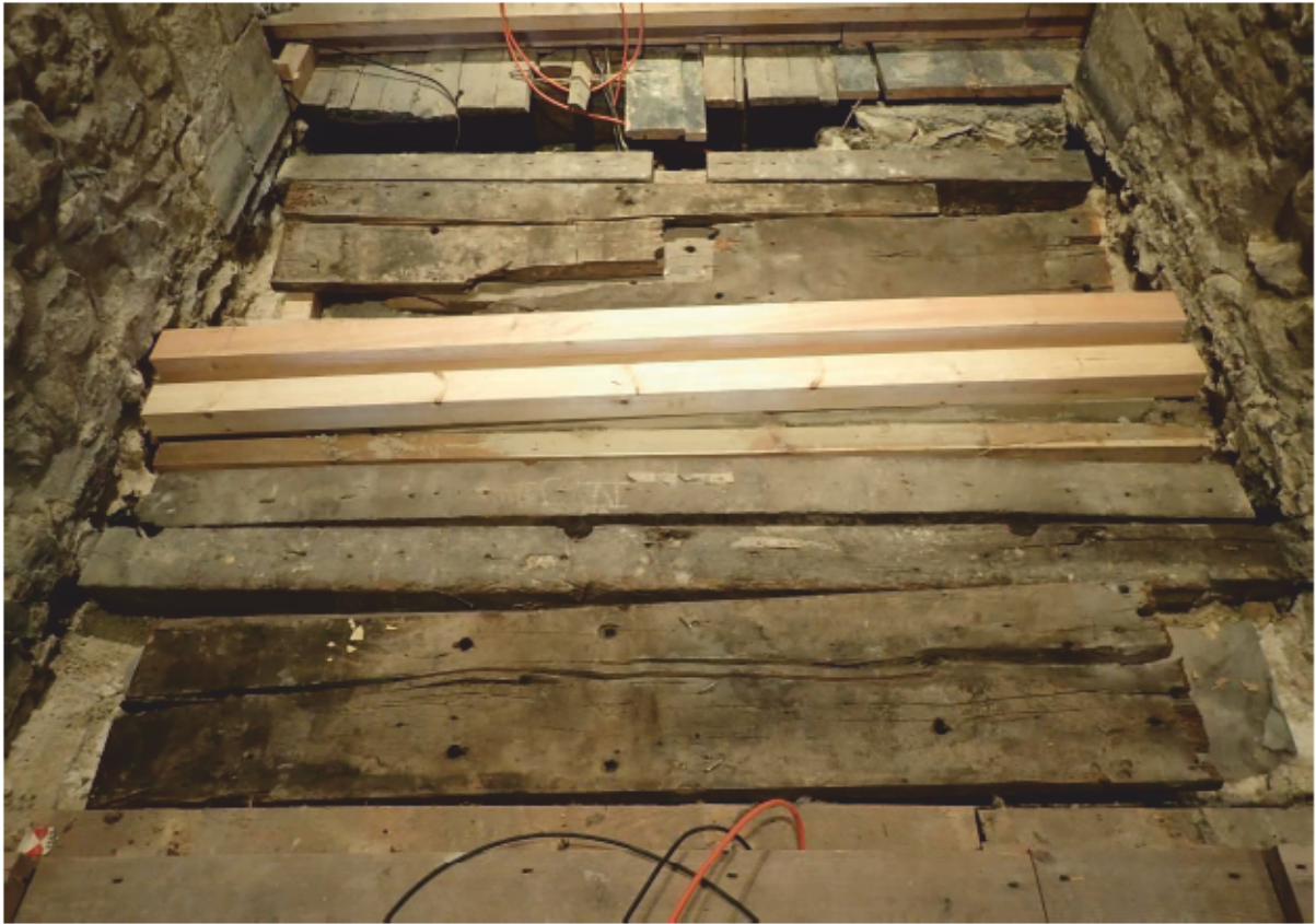
Plate 28 Bay IV Storage of Floorboards and Joists (intermediate stage)
