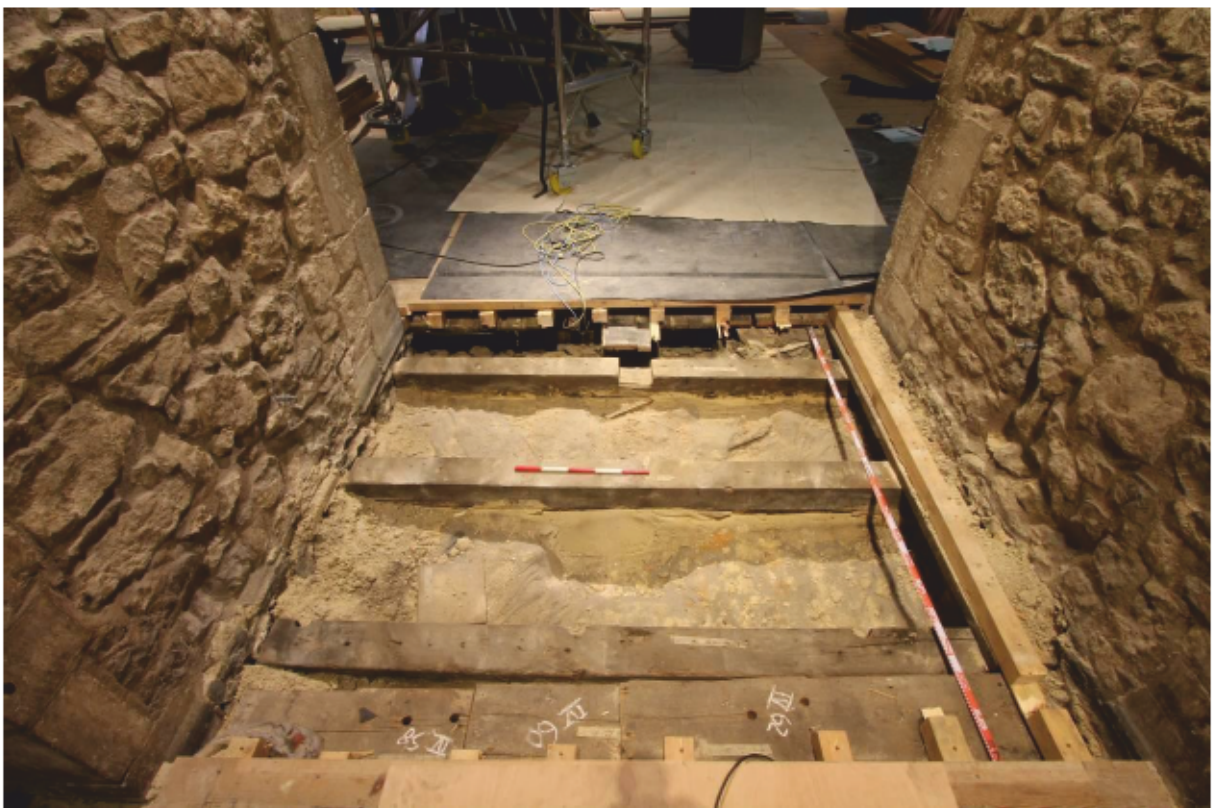
Plate 16 Bay IV Joists 1-3 looking east (2m & 0.5m scales)
