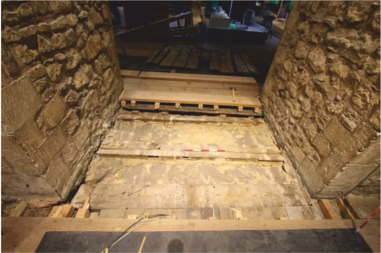
Plate 3 Bay II Joists 1-3 looking west (0.5m scale)
