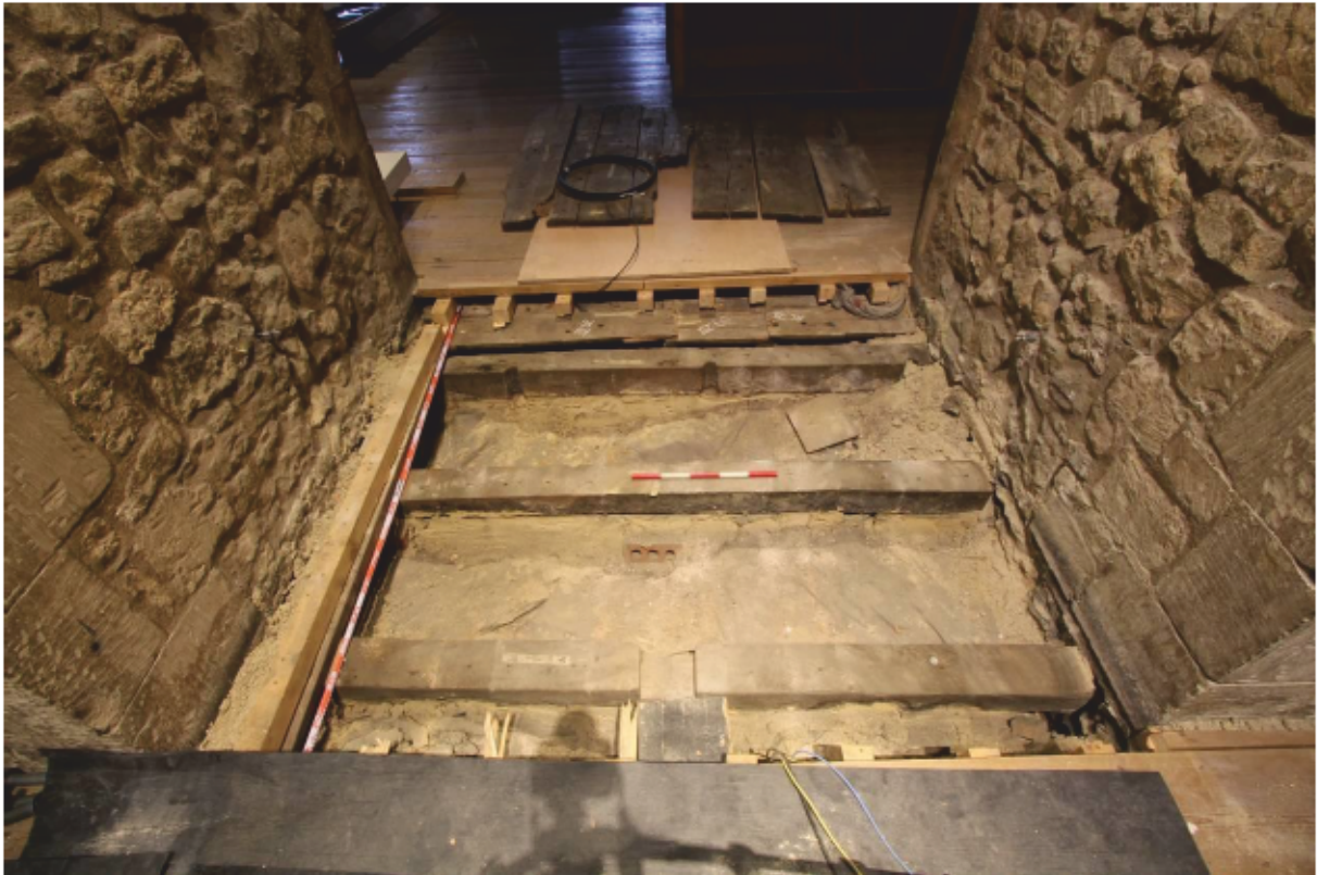
Plate 15 Bay IV Joists 1-3 looking west (2m & 0.5m scales)
