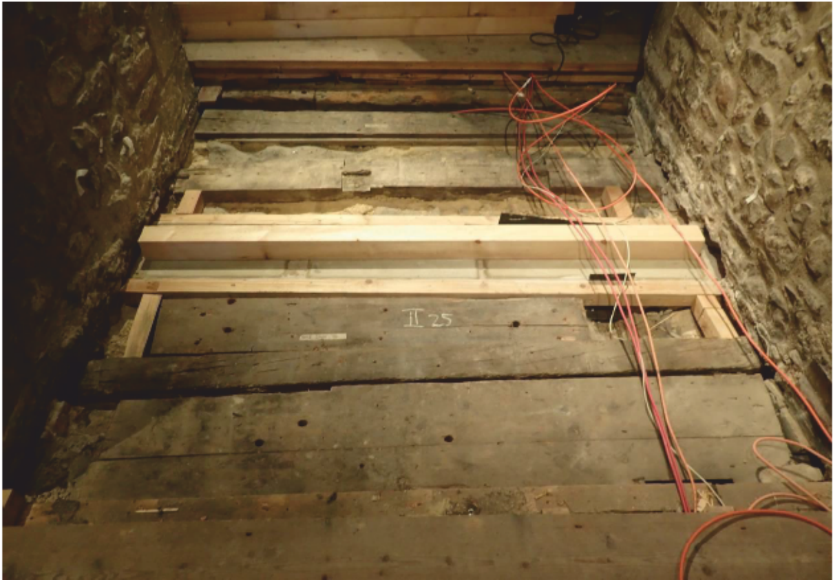
Plate 26 Bay V Storage of Floorboards and Joists (intermediate stage)
