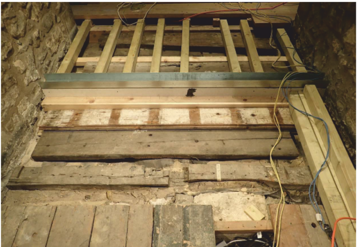
Plate 31 Bay III Storage of Floorboards and Joists
