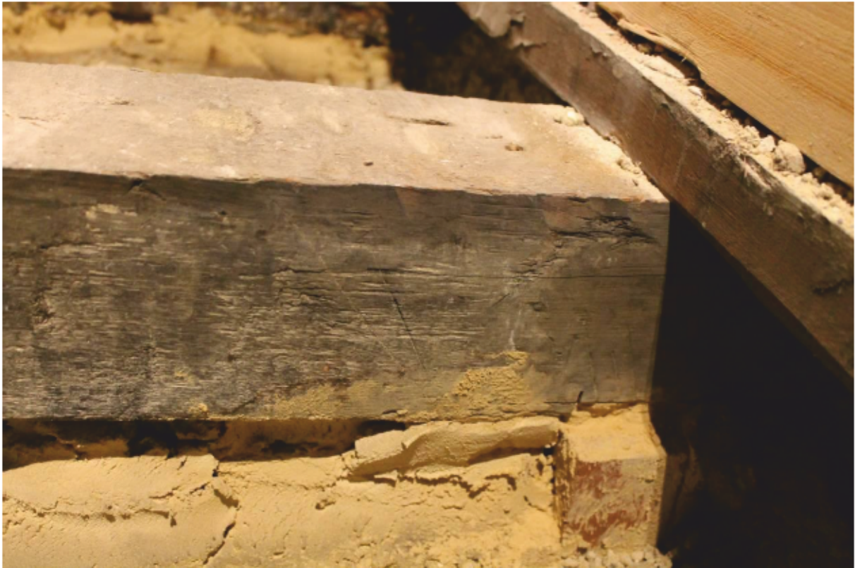
Plate 17 Bay IV Joist 2 fair-face mark
