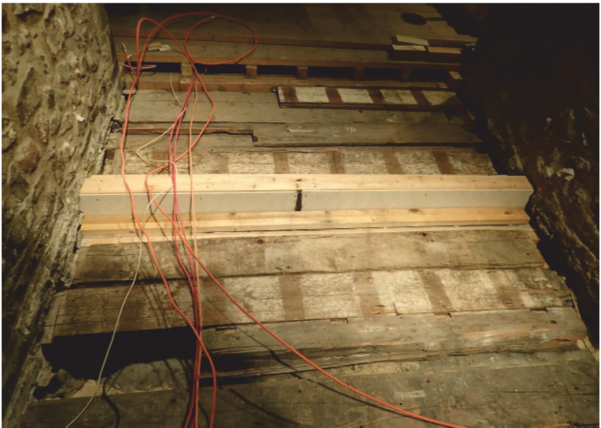
Plate 27 Bay V Storage of Floorboards and Joists
