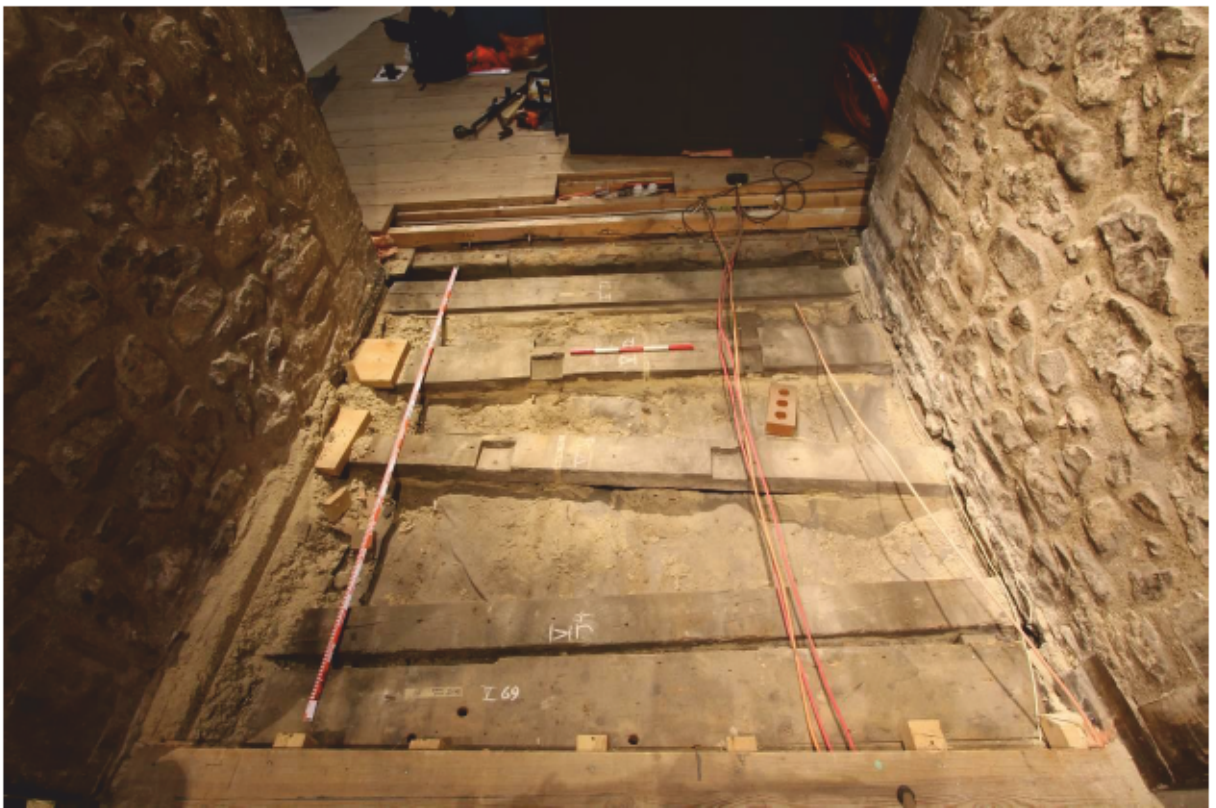
Plate 23 Bay V Joists 1-4 looking east (2m and 0.5m scales)
