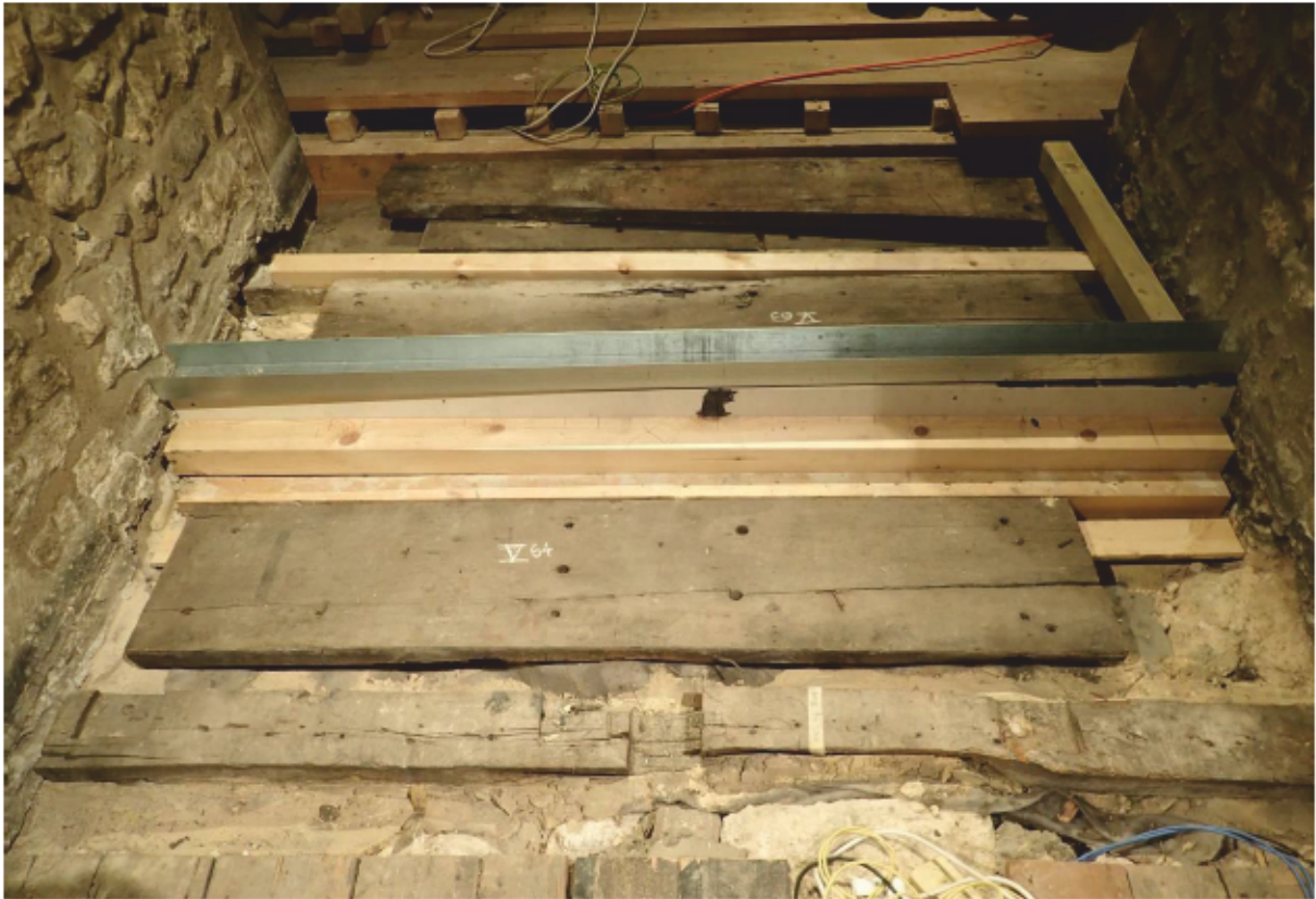
Plate 30 Bay III Storage of Floorboards and Joists (intermediate stage)
