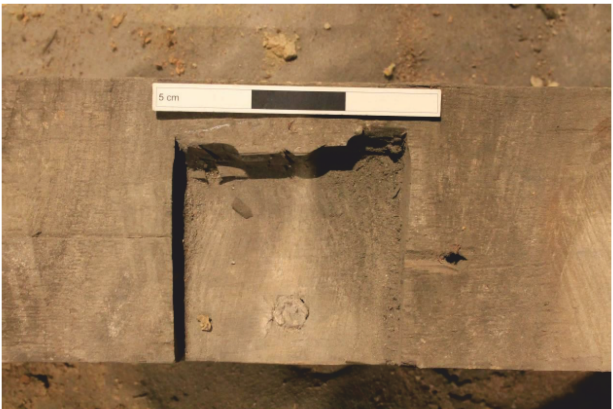
Plate 25 Bay V Joist 3 detail of southern rebate (0.15m)
