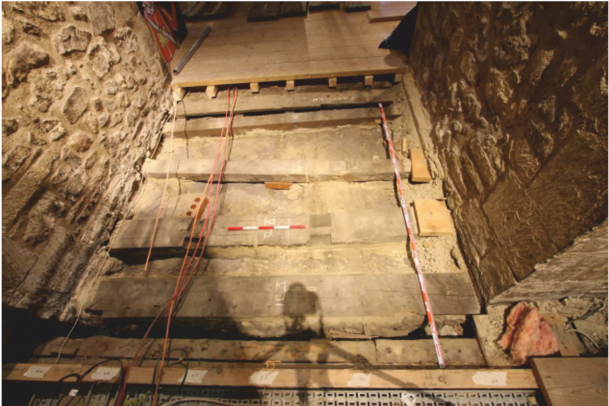
Plate 22 Bay V Joists 1-4 looking west (2m and 0.5m scales)
