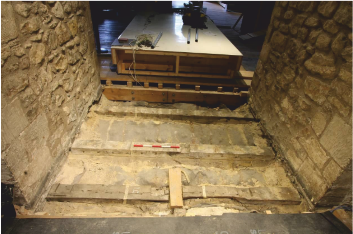
Plate 7 Bay III Joists 1-3 looking west (0.5m scale)
