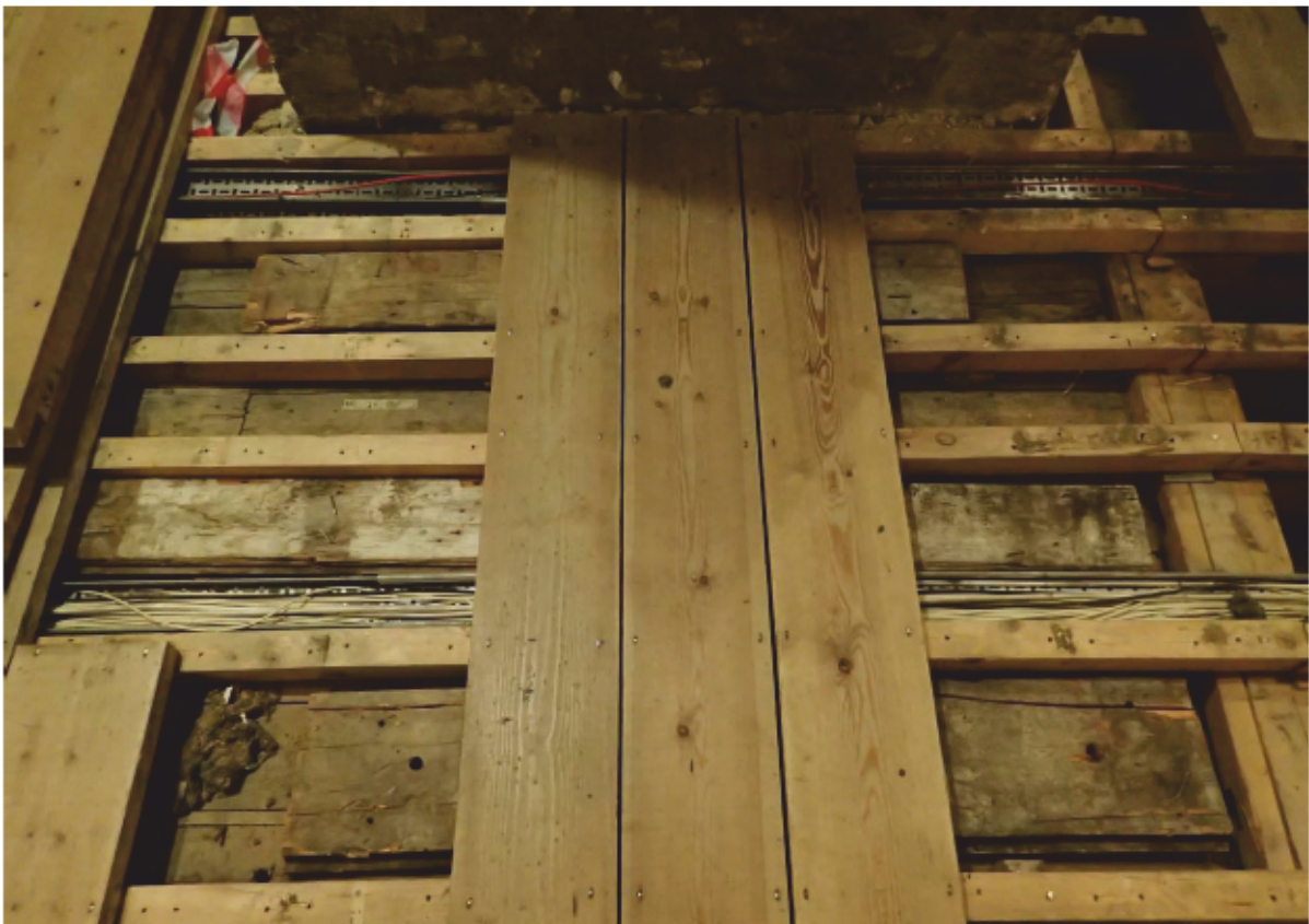
Plate 33 Bay I Storage of floorboards below modern floor structure
