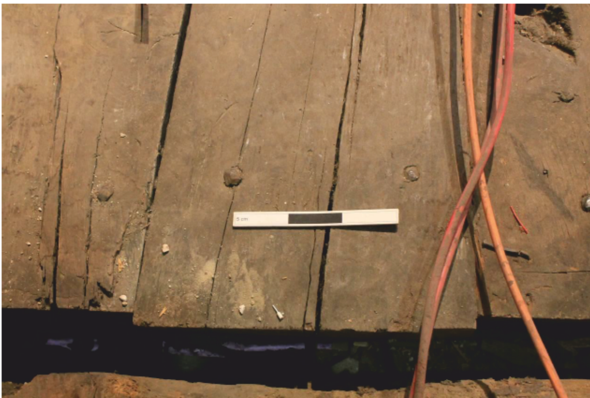
Plate 20 Bay V Floorboard V-67 and 68 (east) detail of nails (0.15m scale)
