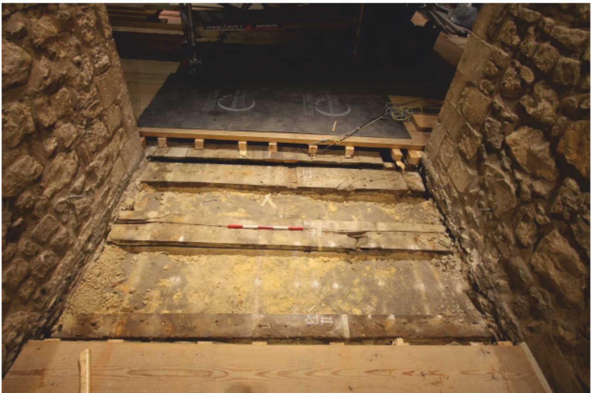
Plate 4 Bay II Joists 1-3 looking east (0.5m scale)
