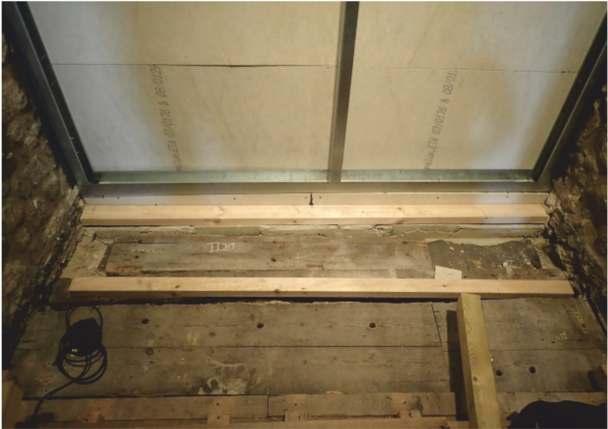
Plate 32 Bay II Storage of Floorboards
