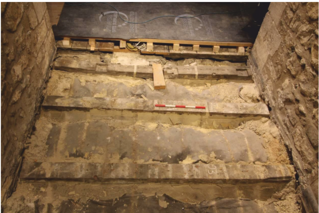
Plate 8 Bay III Joists 1-3 looking east (0.5m scale)
