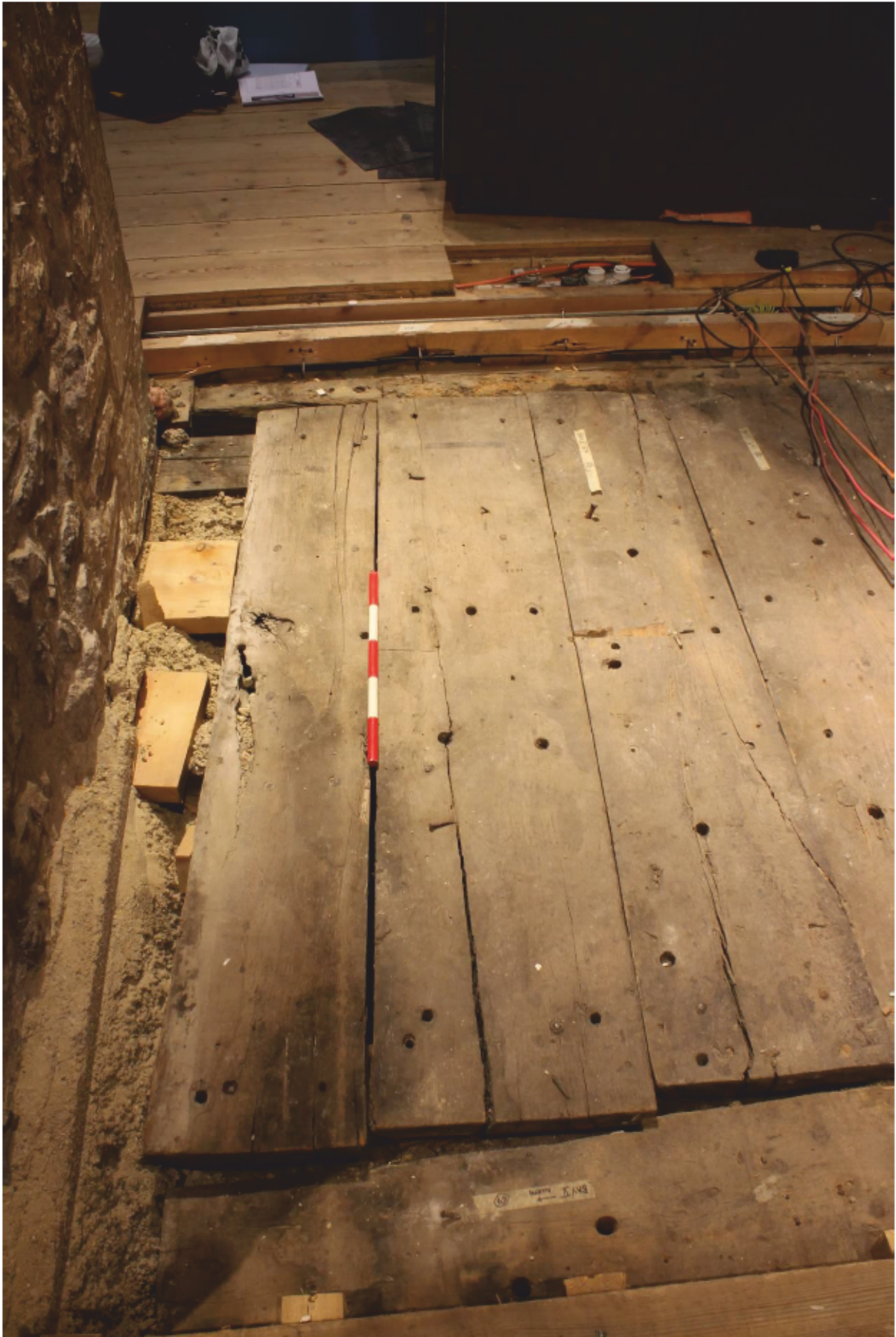
Plate 21 Bay V Floorboards V-63 to V-66 looking east (0.5m scale)
