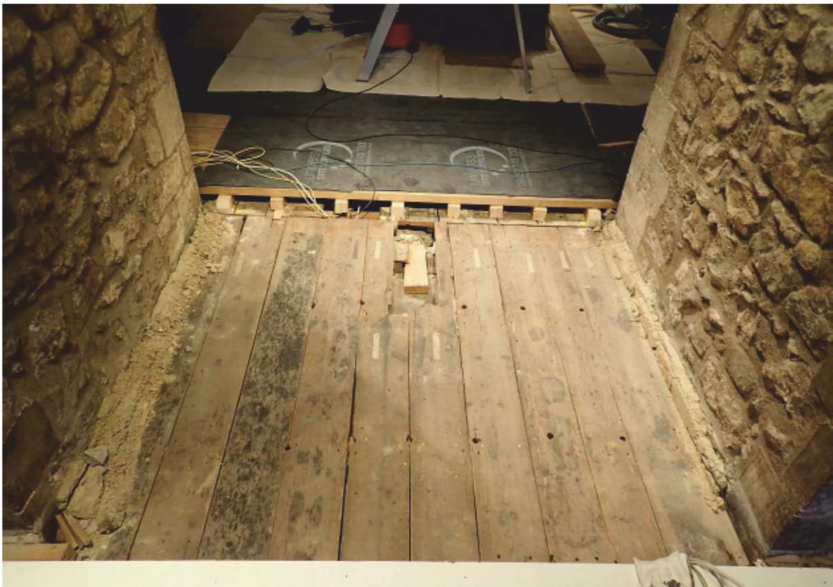
Plate 6 Bay III looking east
