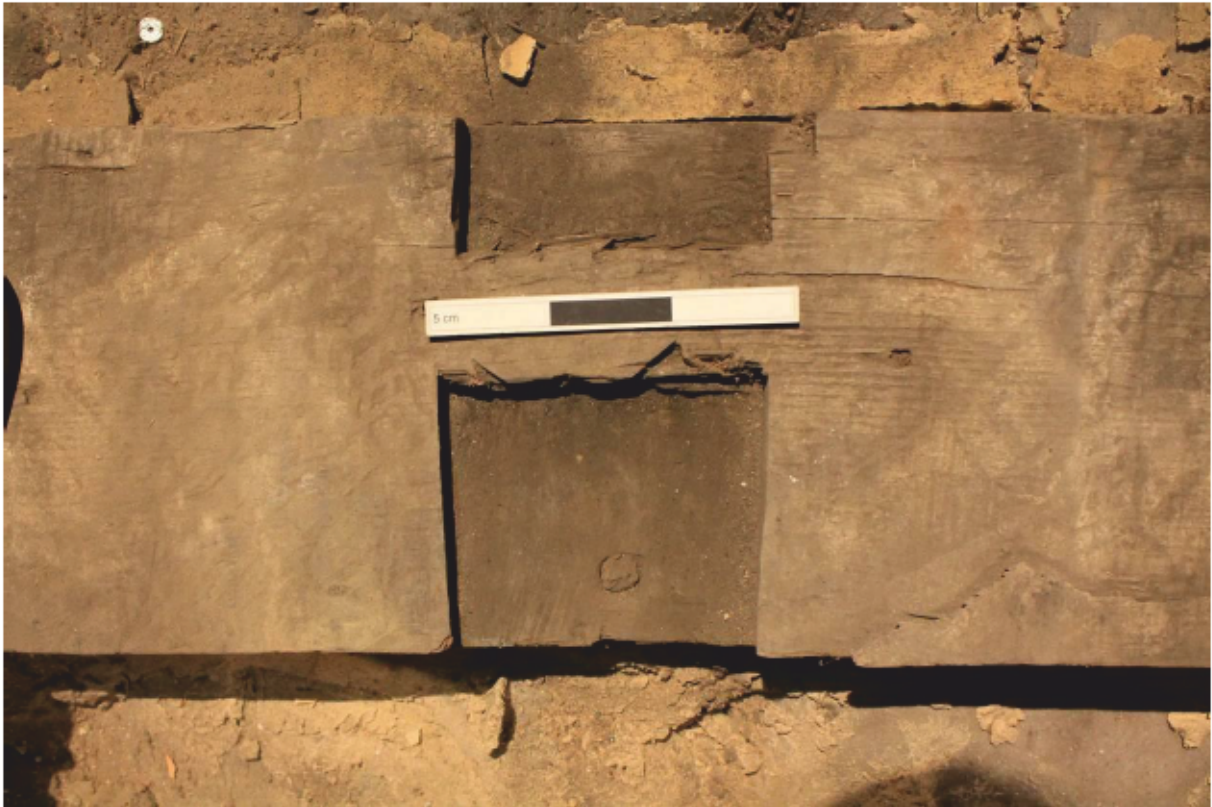
Plate 24 Bay V Joist 2 detail of northern rebate (0.15m)
