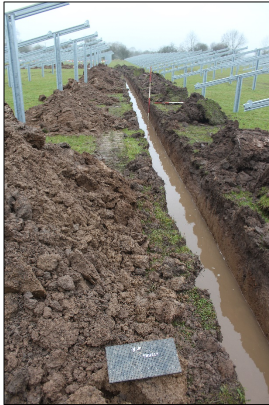
Plate 3: General shot of excavation of cable trench: view west
