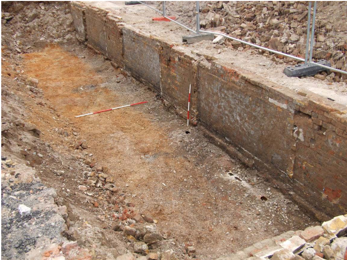
Figure 14: Trench 1, east cellar wall [5]
