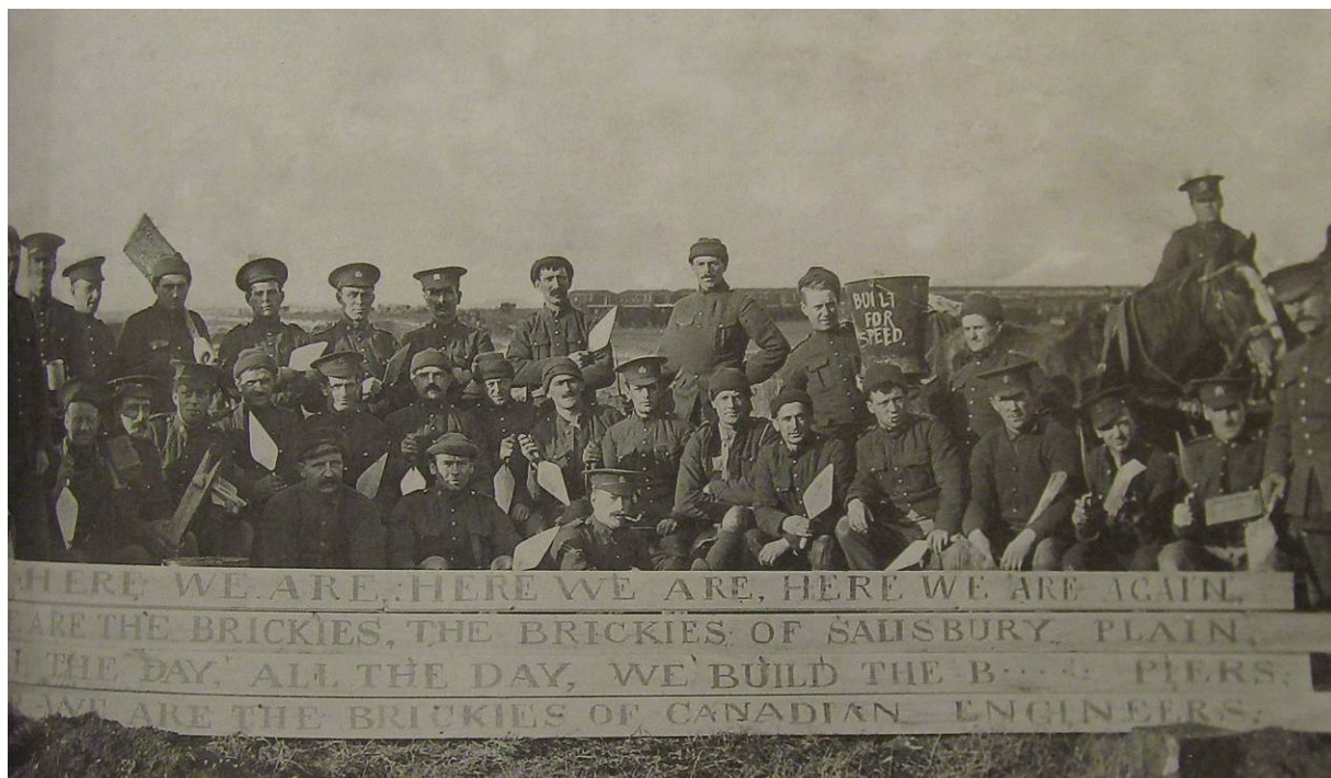
Plate E: Sappers of the Canadian Engineers engaged in building a hutted camp on Salisbury Plain, 1914/15 (© Crawford, T.S. 2012. The Canadian Army on Salisbury Plain: The First Canadian Contingent October 1914-February 1915)
