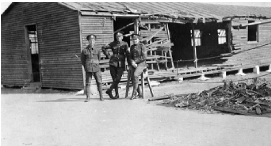
Plate I: Barrack hut at Shorncliffe damaged by enemy aerial bombing, 1917
