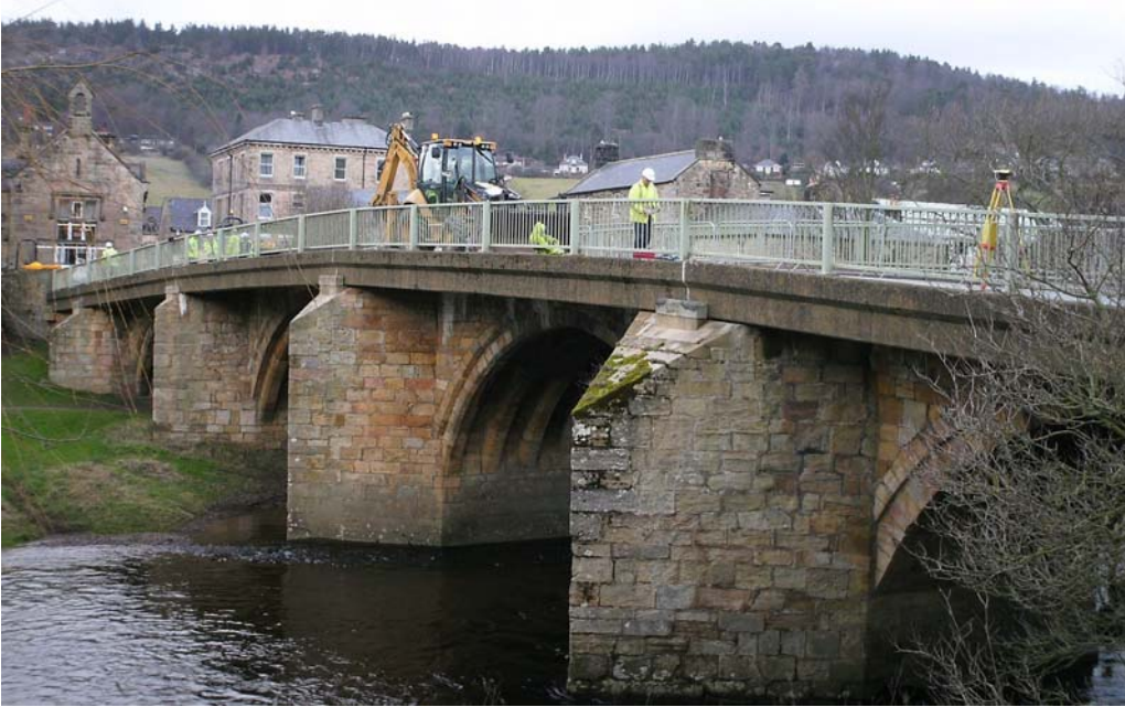
Plate 1. Rothbury Bridge, west side, from the south.
