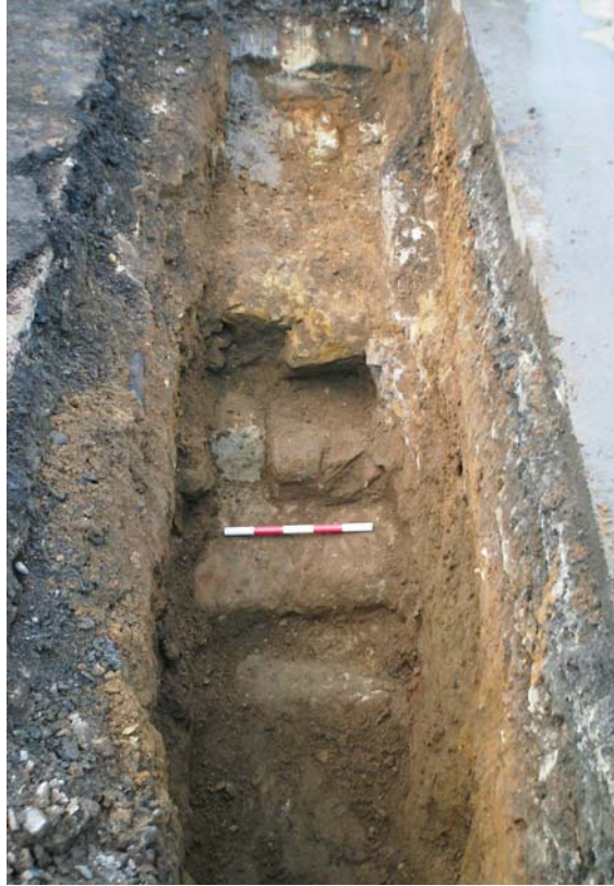
Plate 5. TH 15, masonry [1506], from the south (0.5m scale).
