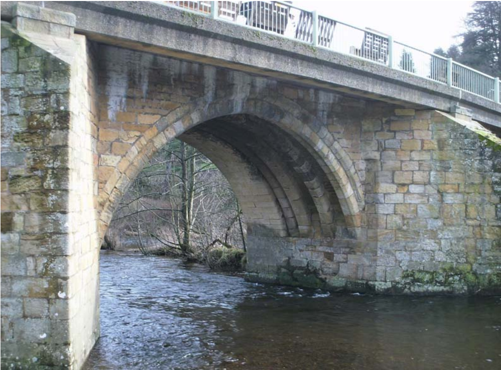
Plate 2. Arch 3 detail, from the west.
