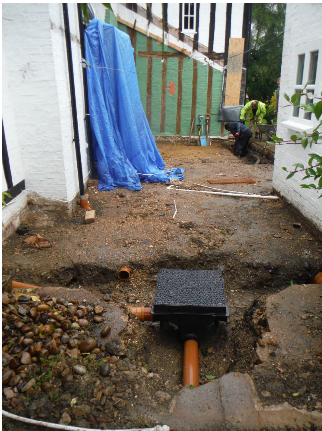
Plate 1: Overview of site, view north
