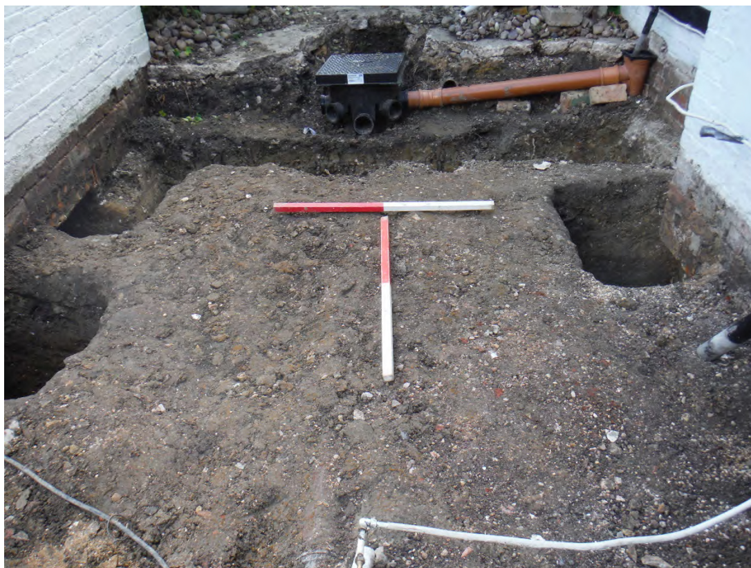
Plate 6: Overview of Footings 2, 3, 4 and 5, view south
