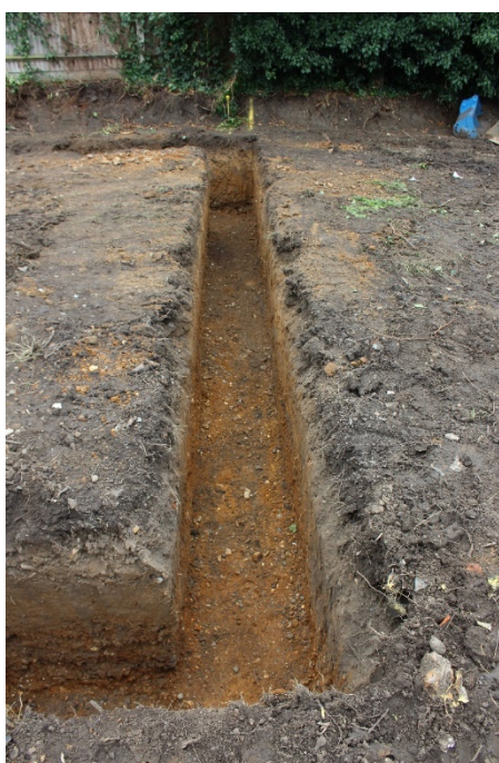
Plate 5: Strip footing, looking east
