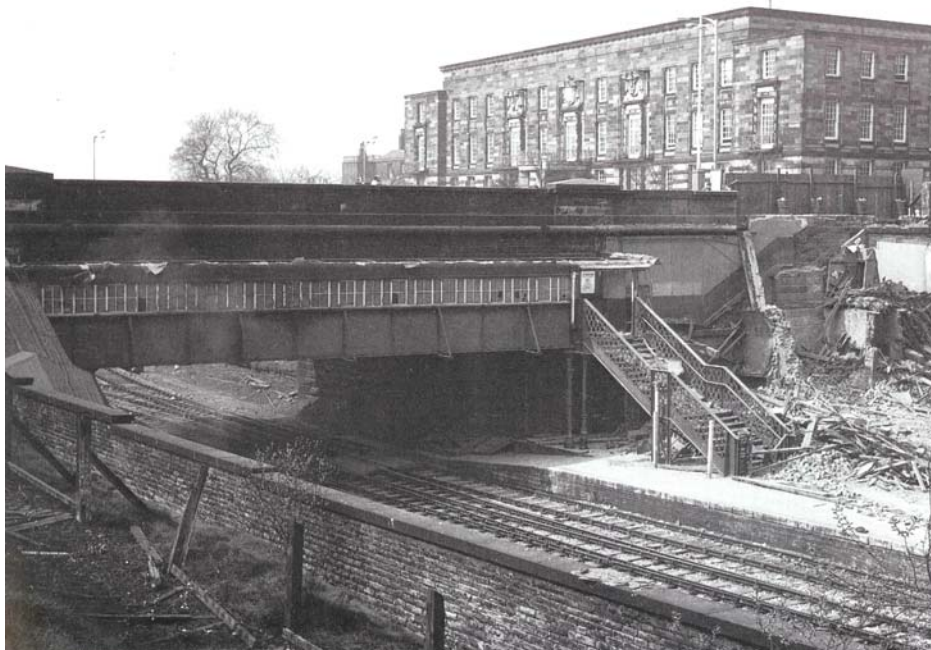
Plate D6. 'Up' platform and partly demolished station buildings, 1971, looking north-west.
