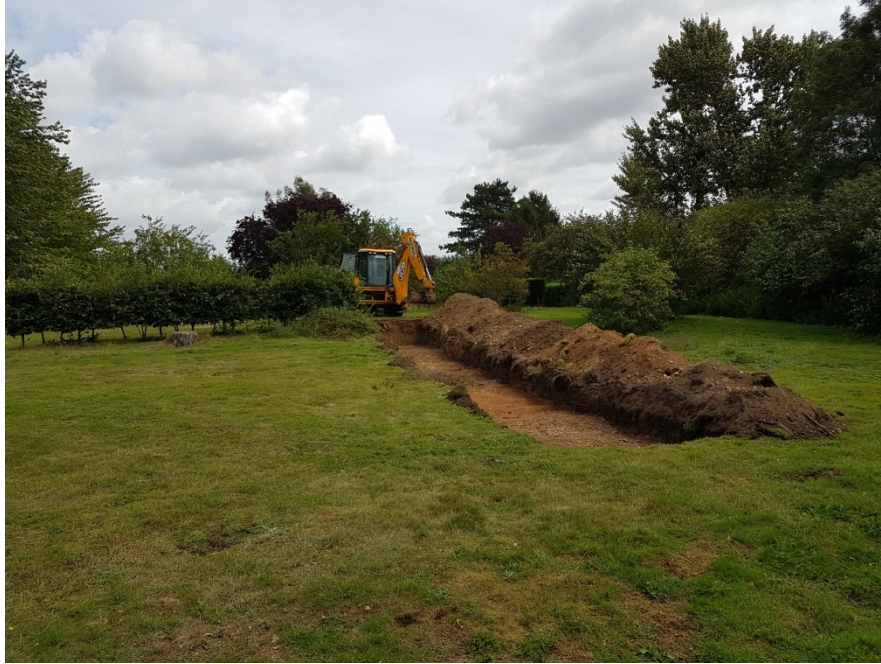
Image 1: East facing view of site
