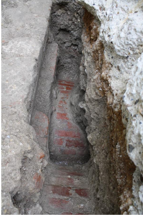
Plate 9: Test Pit 5, facing south. Culverts [11] and [12] and associated brick line [10].
