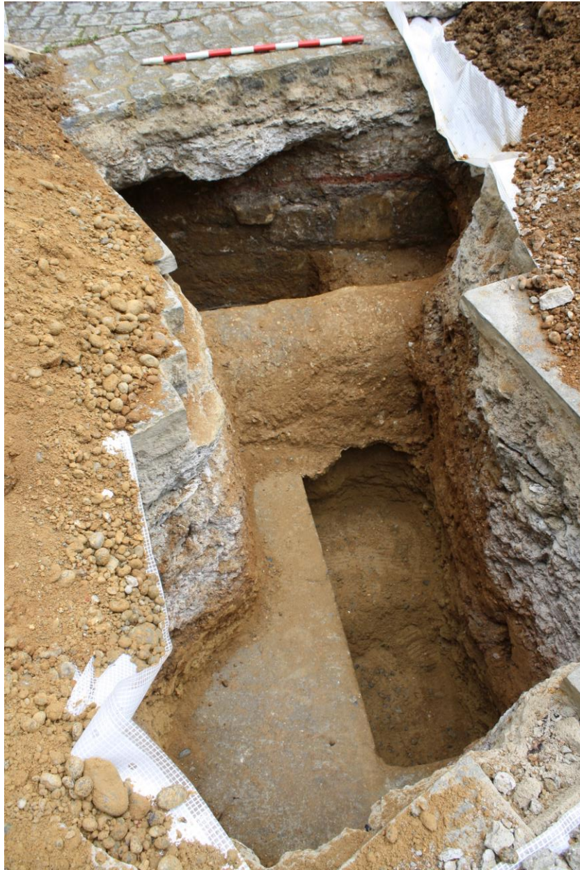
Plate 2: Test Pit 1 showing the concrete associated with the underground car park and services, facing south-west.
