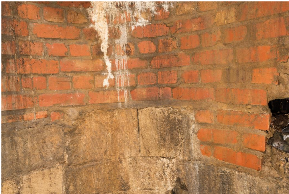
Plate 6: Investigation 4, the well. Point where modern bricks were used to rebuild part of the structure, facing north-west.
