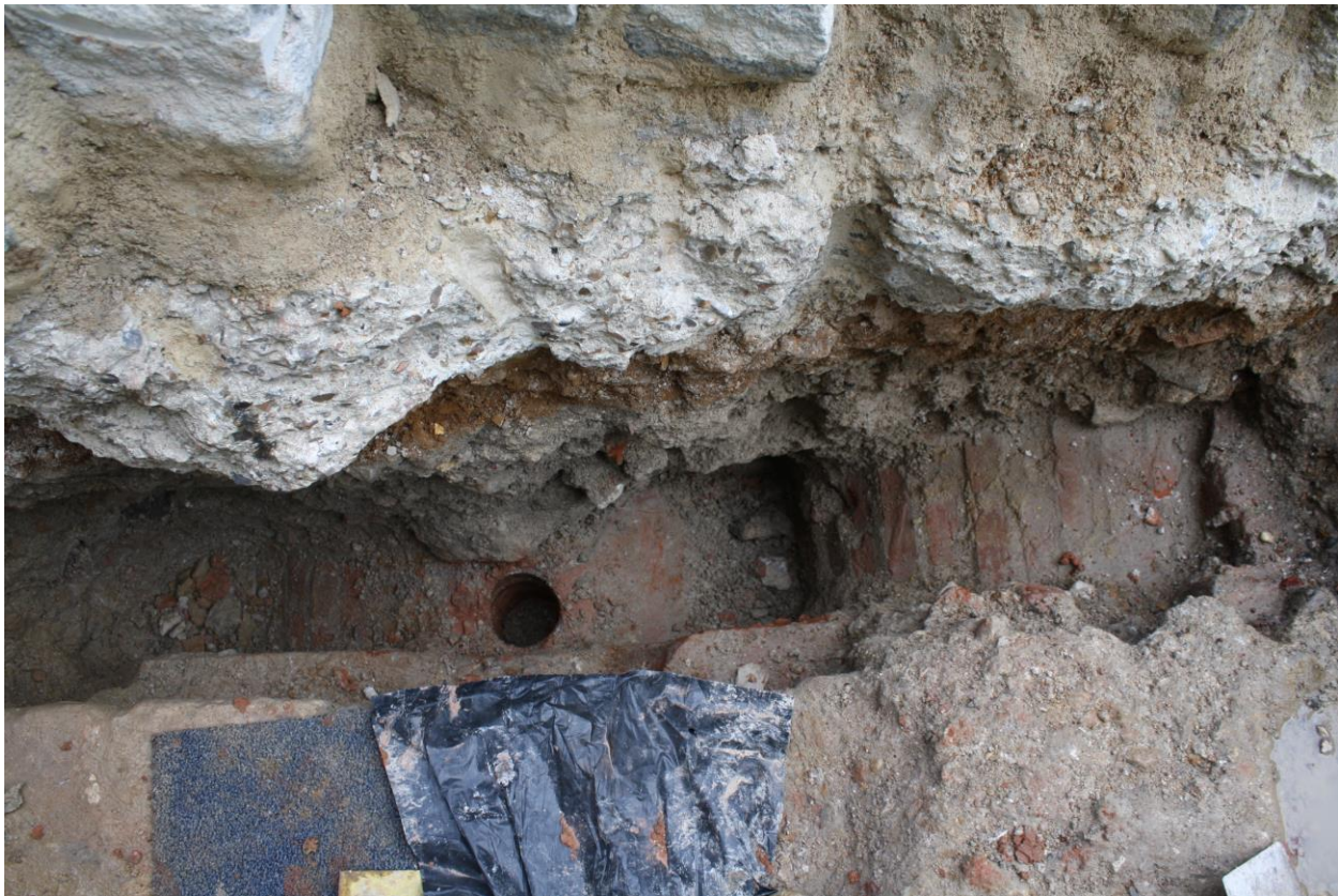
Plate 10: Bore hole in culvert [12] in Test pit 5, facing west.
