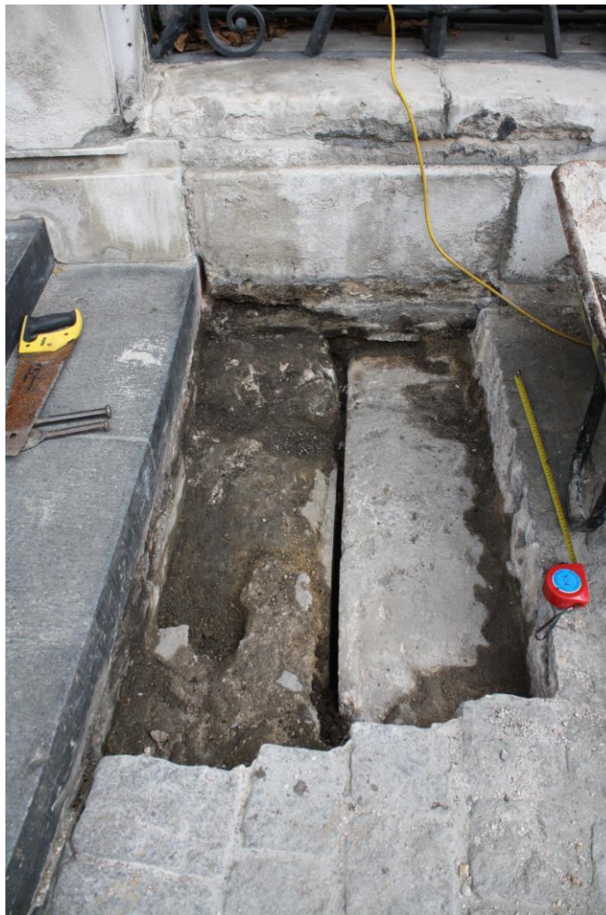
Plate 5: Test Pit 3, the Cathedral's foundation can be seen to the left.
