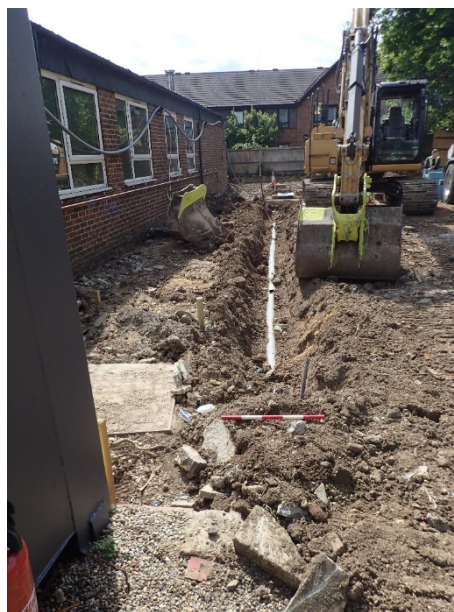
Plate 2: Drainage Excavation, Facing West
