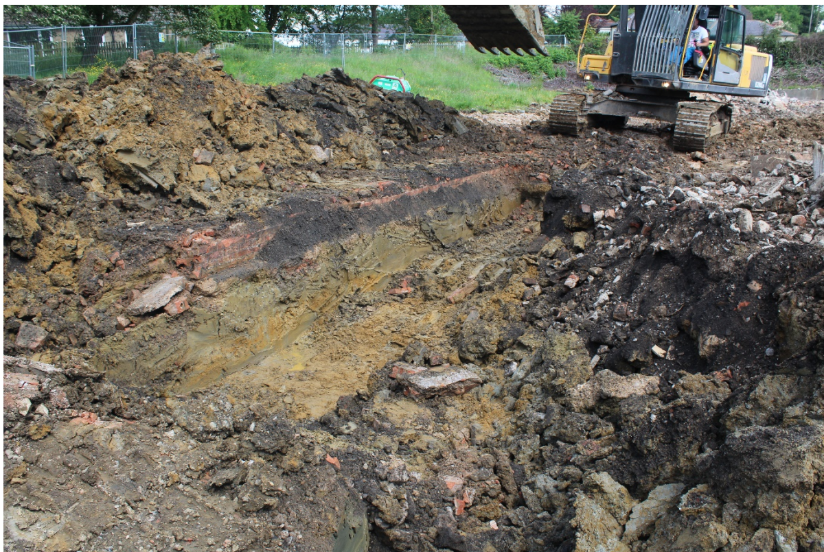
Plate 1: Northwest facing view of removal of remains of previous development.
