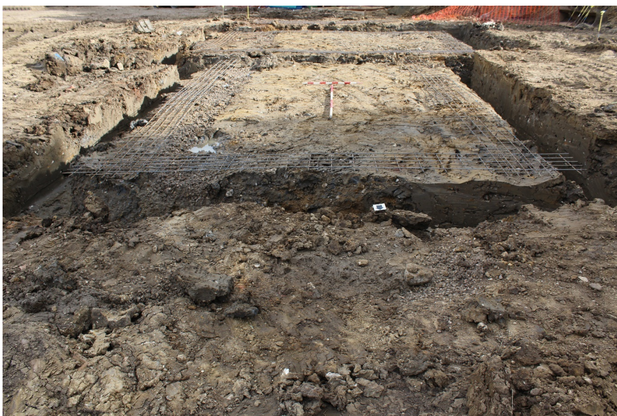
Plate 8: South facing view of Plot B footings.
