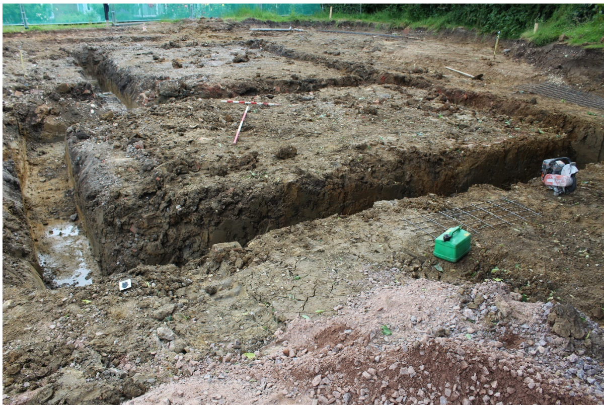
Plate 7: South facing view of Plot A footings.
