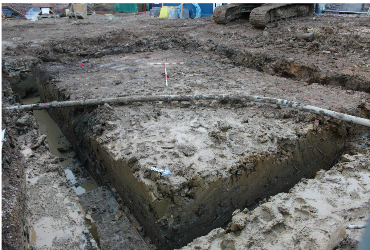
Plate 10: West facing view of Plot H footings.
