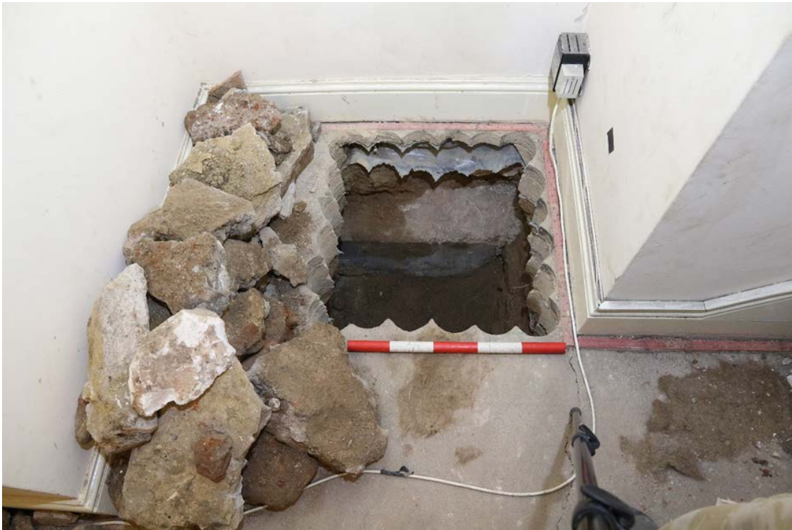
Plate 4: Test Pit B01 West facing section showing removed rubble and underpinning
