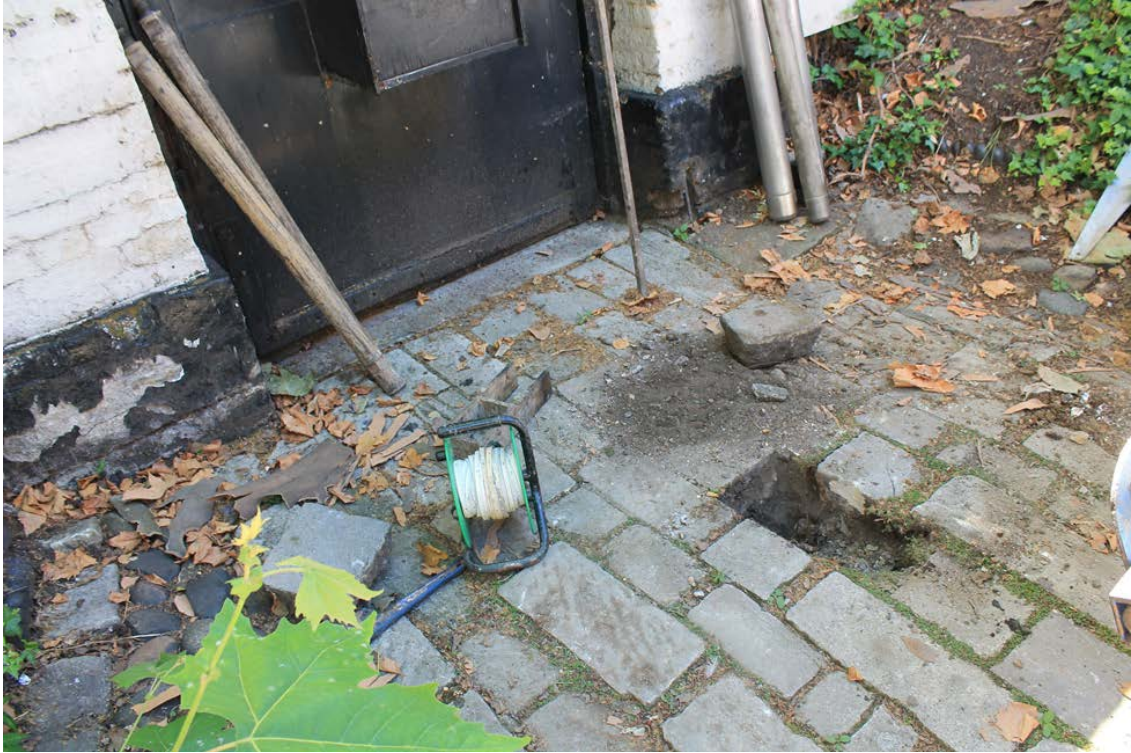
Plate 1. Location of Borehole X01 looking south east towards boundary wall
