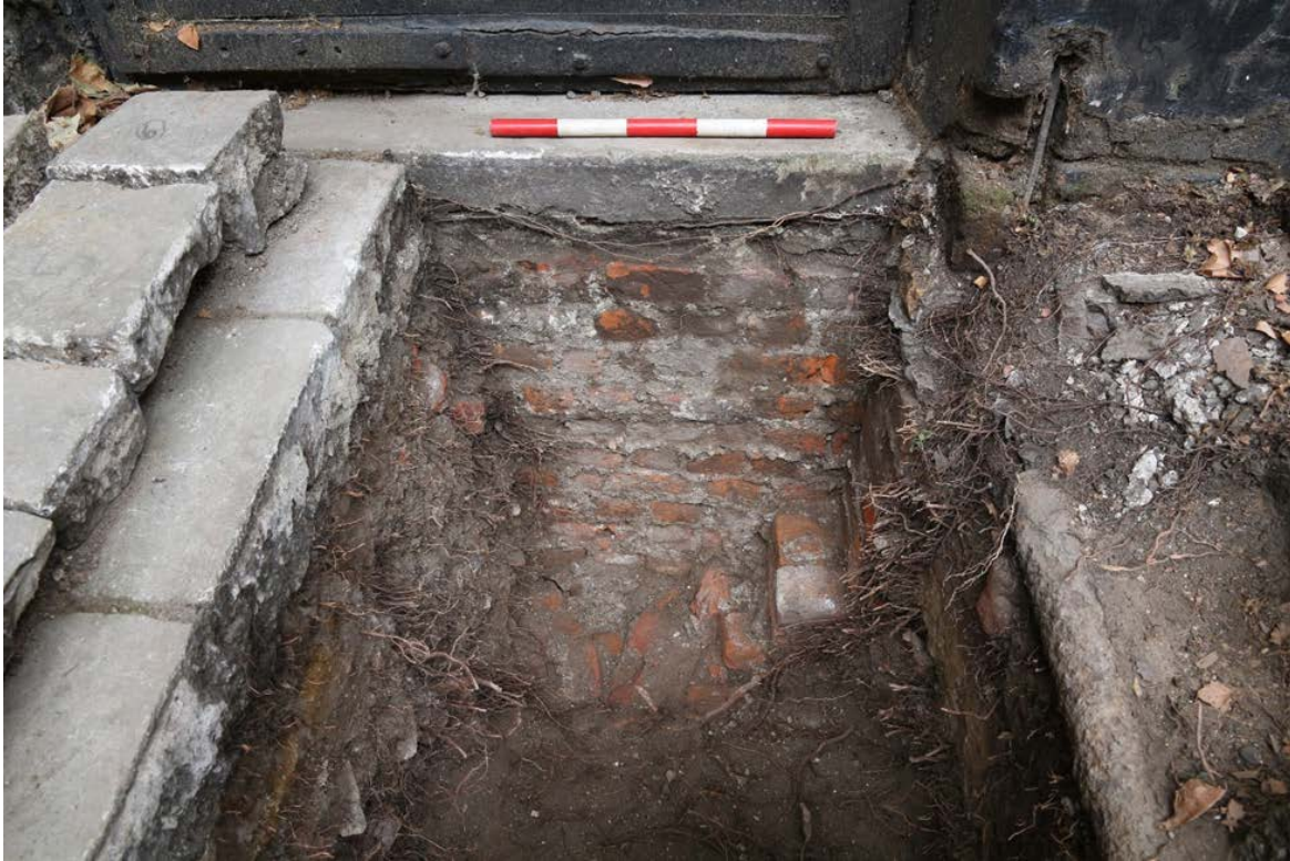
Plate 3. Test pit X01 west facing section showing [8] boundary wall foundation.
