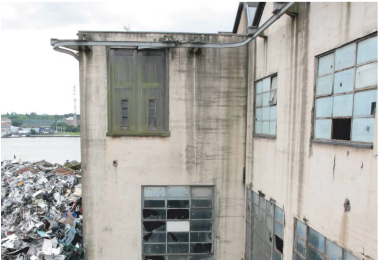
Plate 54 Doors and external track for cradle at second floor
