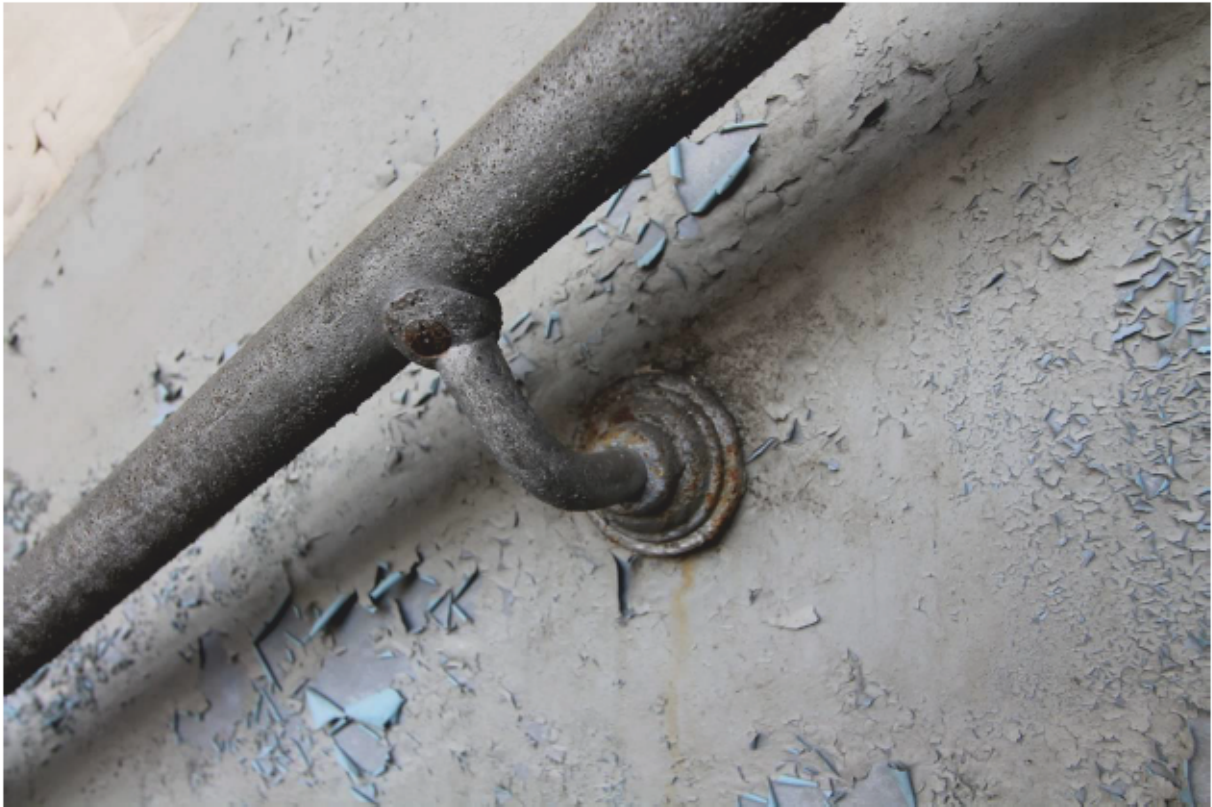
Plate 24 Detail of handrail at first floor level
