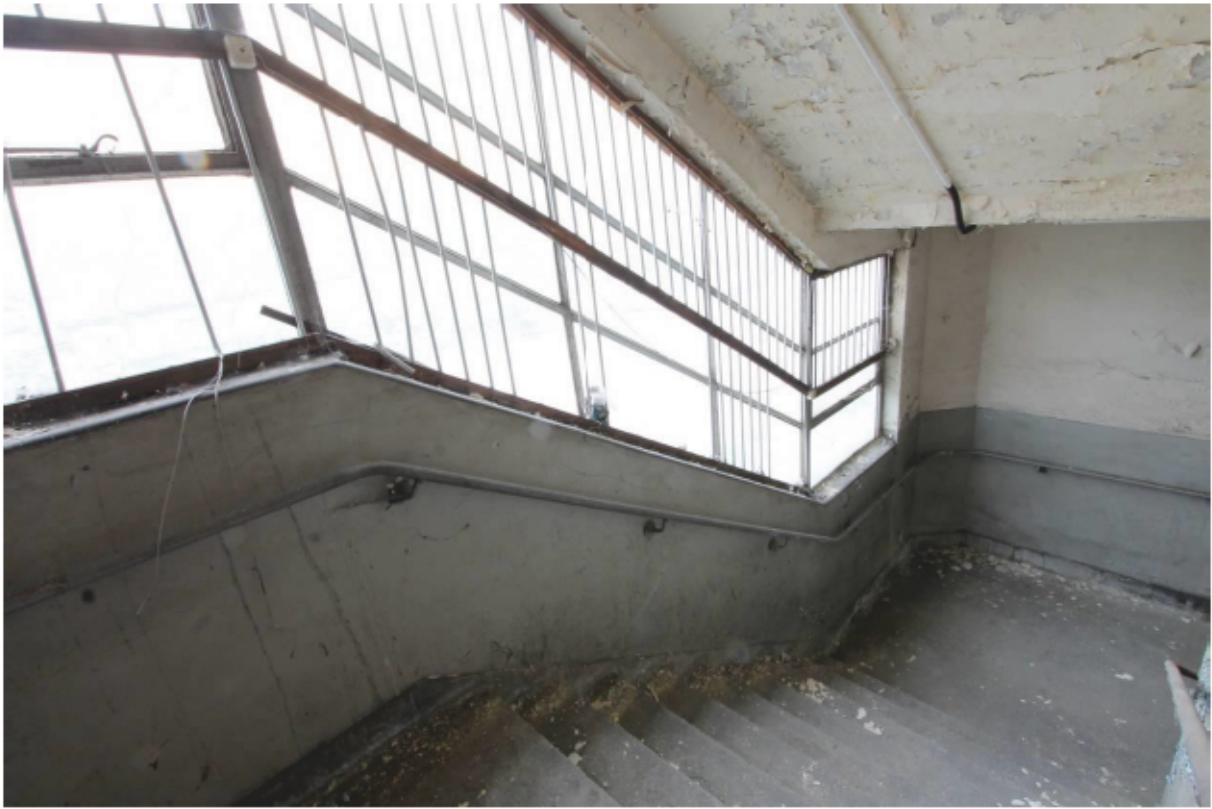
Plate 23 Stairwell and fenestration at first floor level
