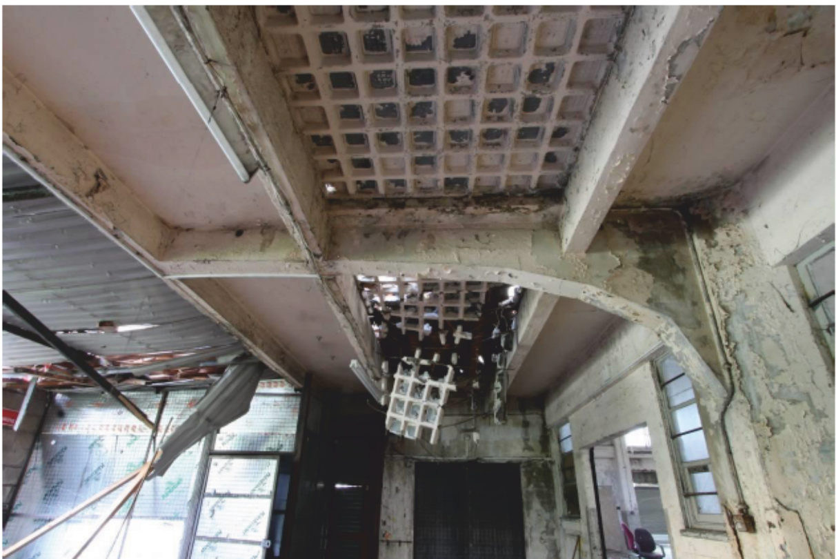
Plate 27 cantilever and glass block lights, looking north
