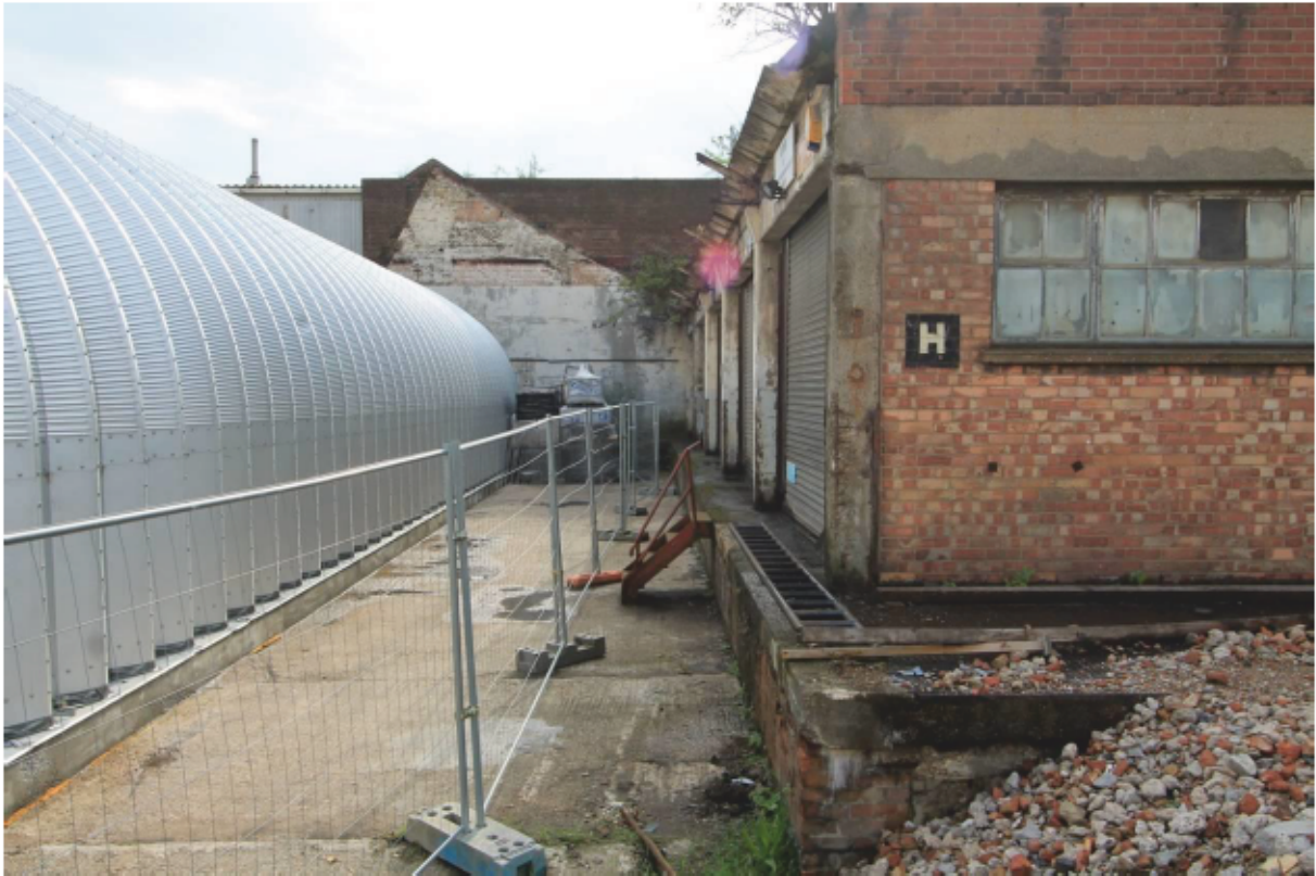
Plate 12 Scar of former bay, later removed
