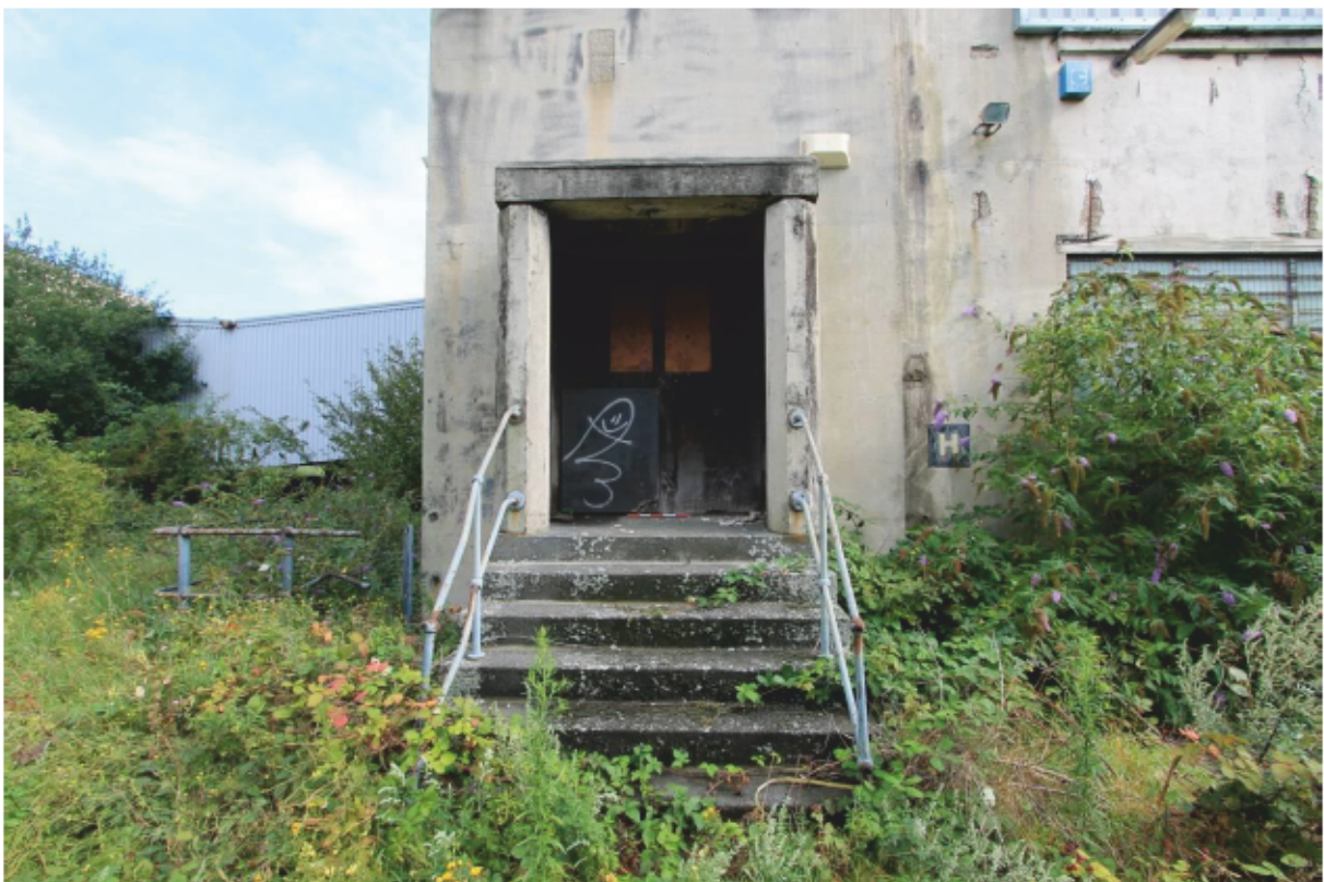
Plate 15 Door opening to southern stairwell
