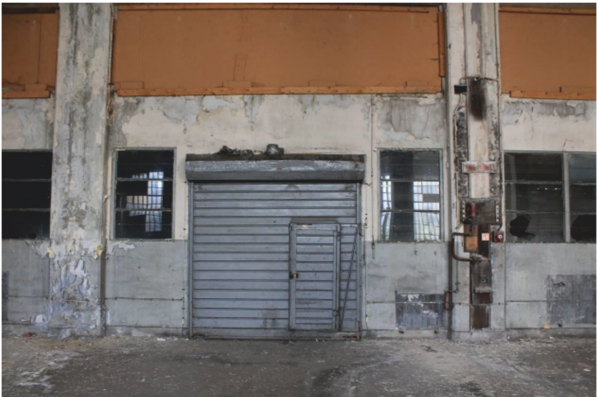
Plate 25 Typical opening to western loading bay
