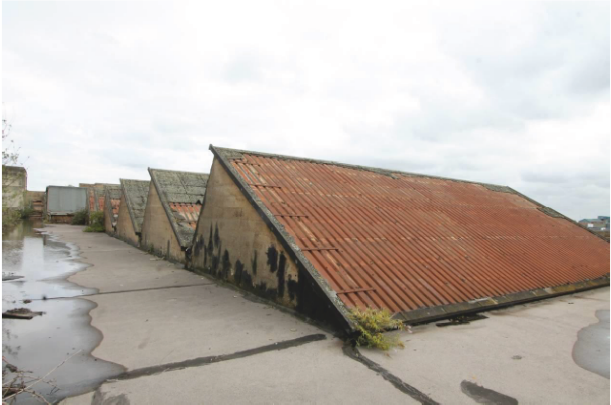
Plate 55 North-light roof looking north-east
