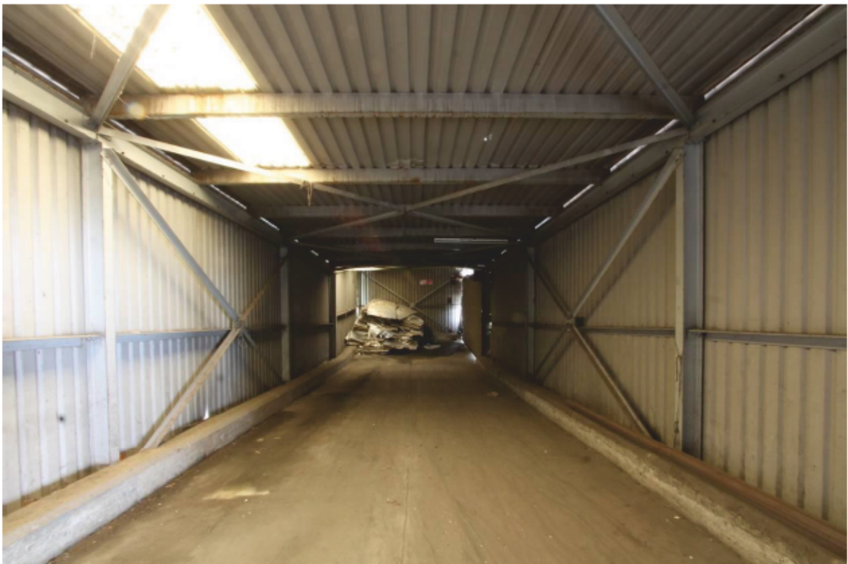
Plate 45 Modern ramped loading bay
