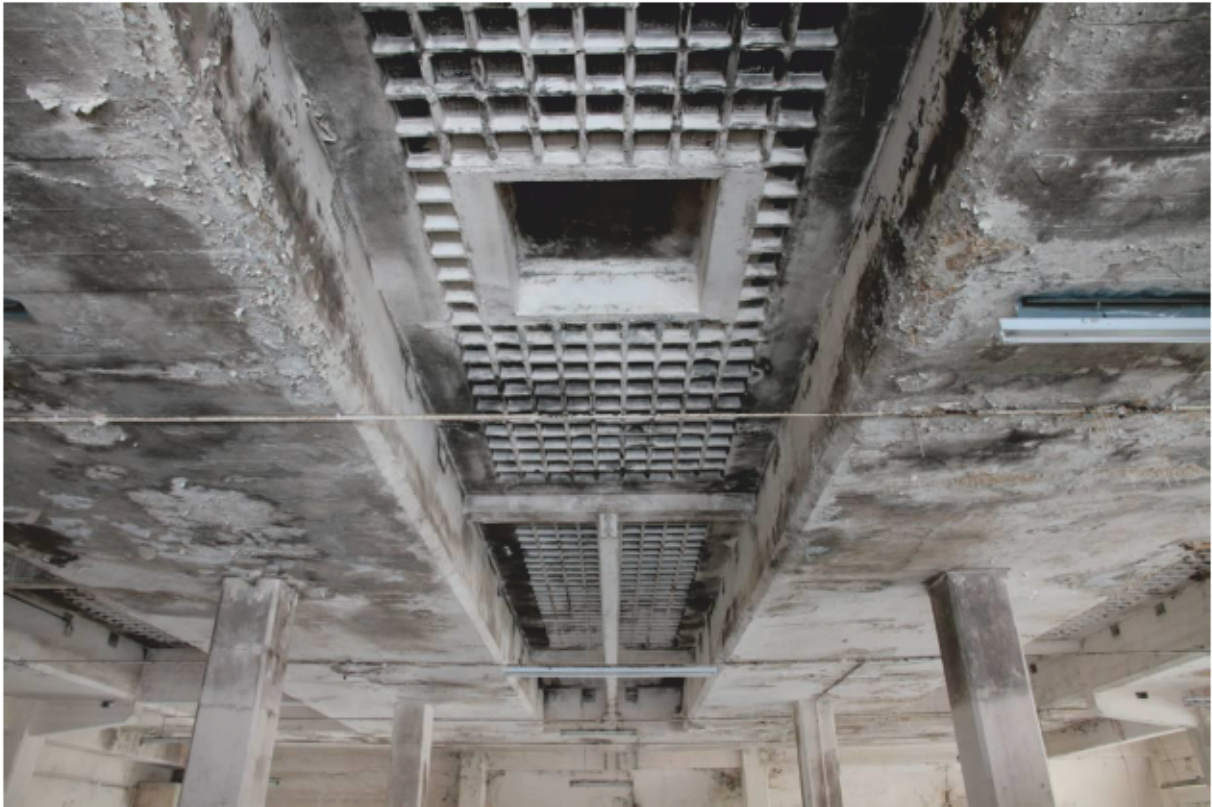
Plate 46 Glass block lights in ceiling over raised northern bays
