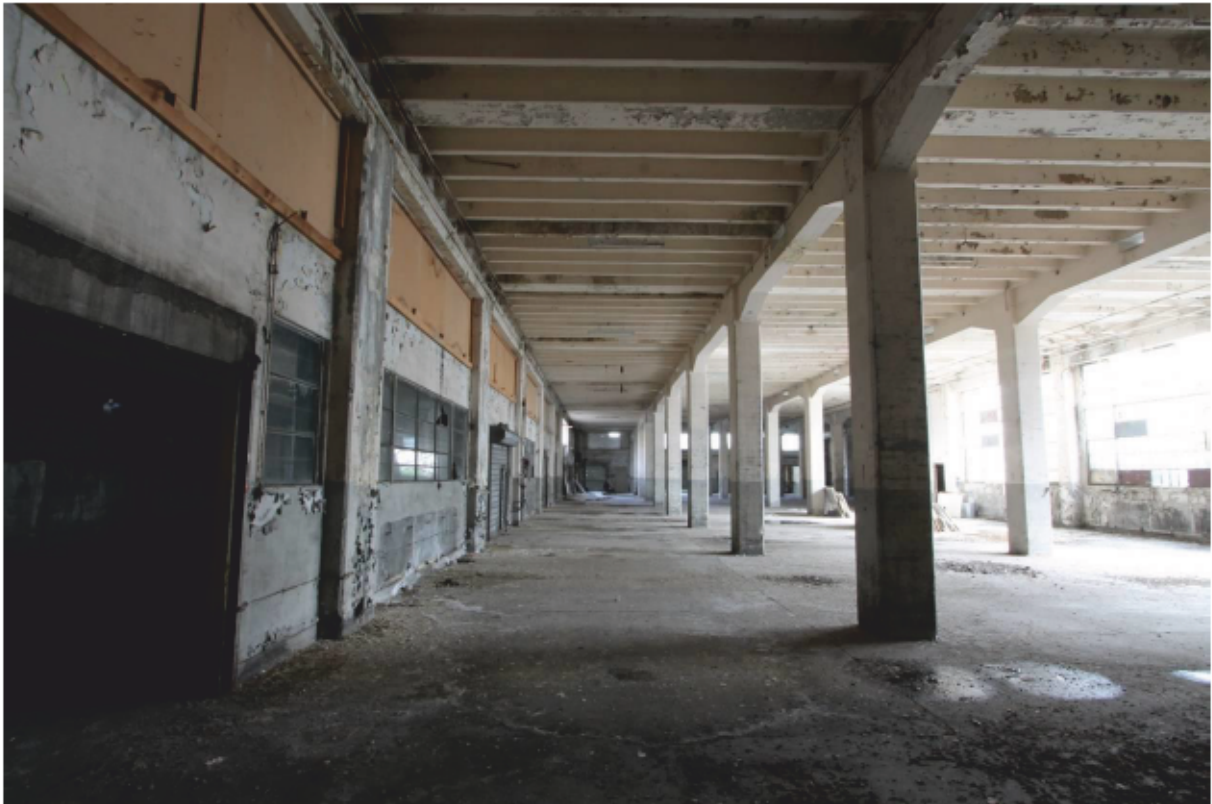
Plate 18 Ground floor, looking north
