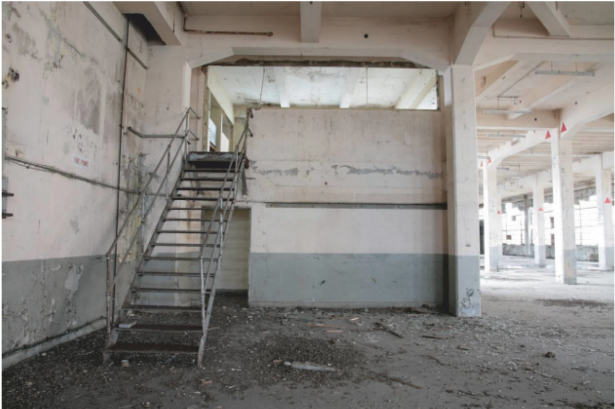
Plate 44 Office above toilets
