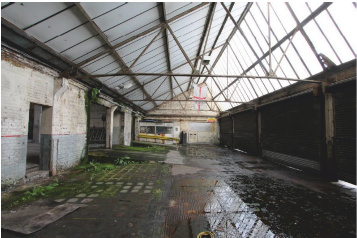
Plate 29 North-light extension looking west
