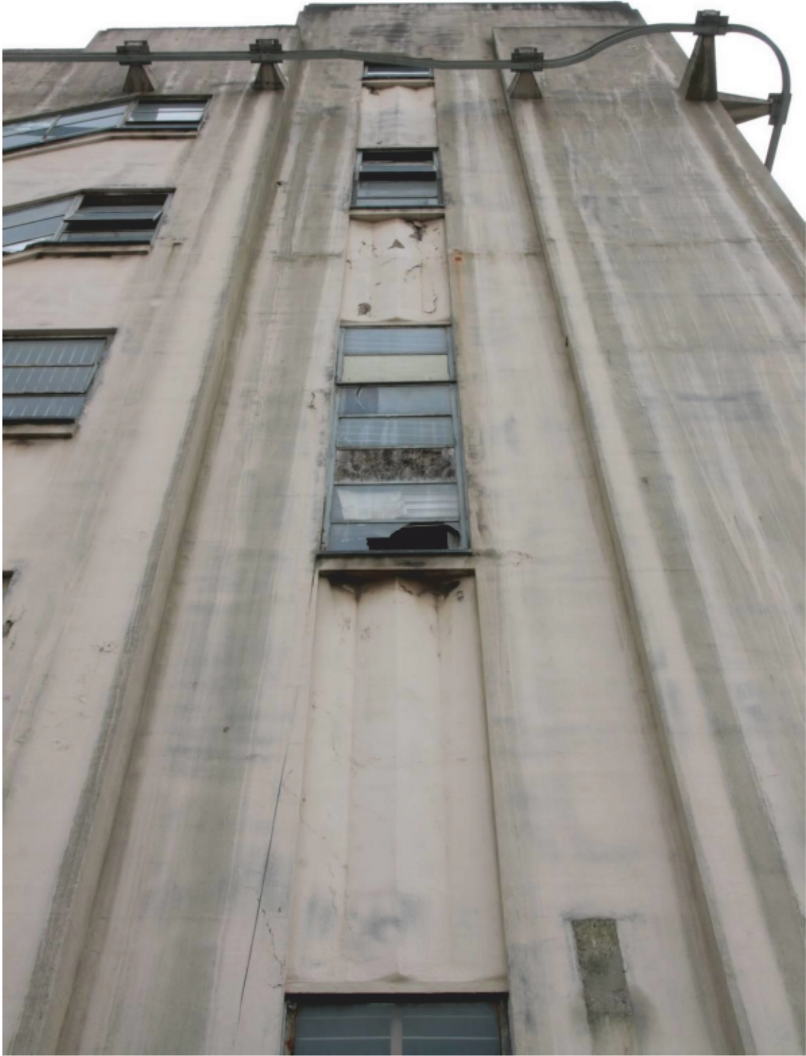
Plate 7 Recessed chevron detailing to stair-bay (south) and external track
