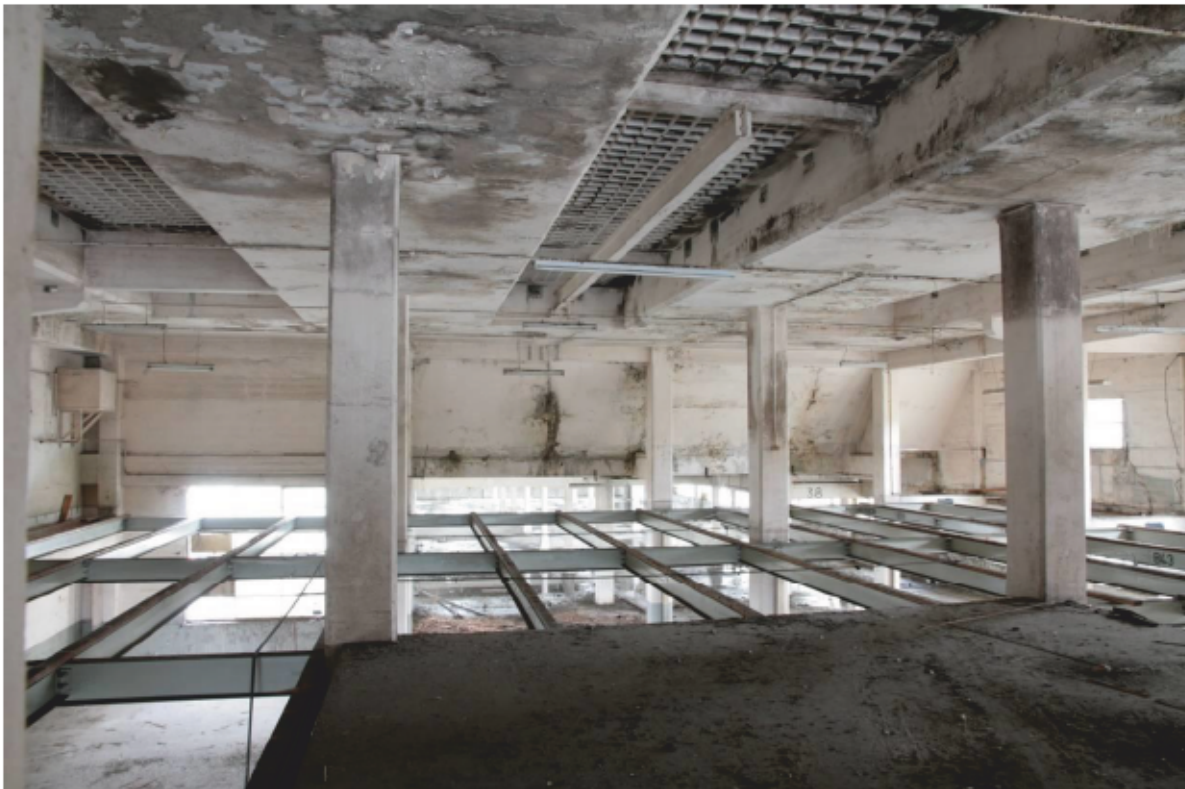
Plate 49a Second floor, northern bays, above mezzanine, looking south
