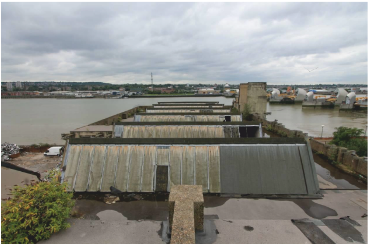
Plate 56 North-light roof looking south
