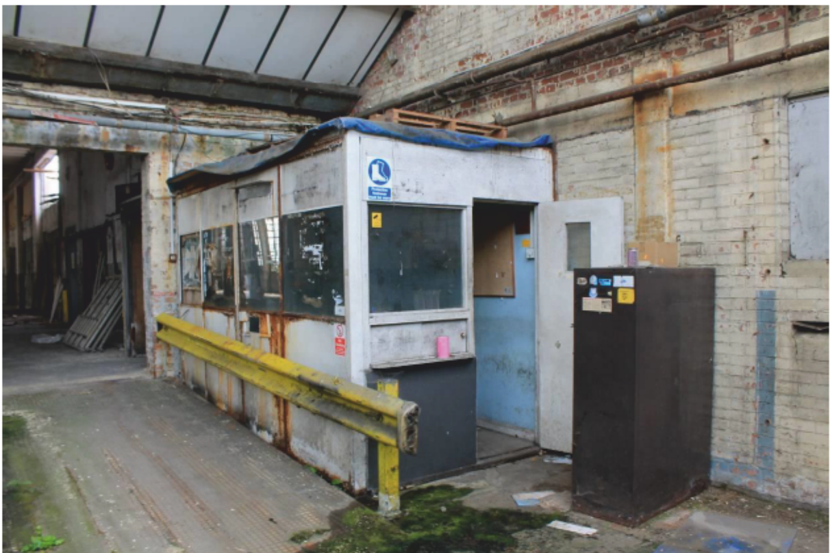
Plate 31 Small office in northern extension
