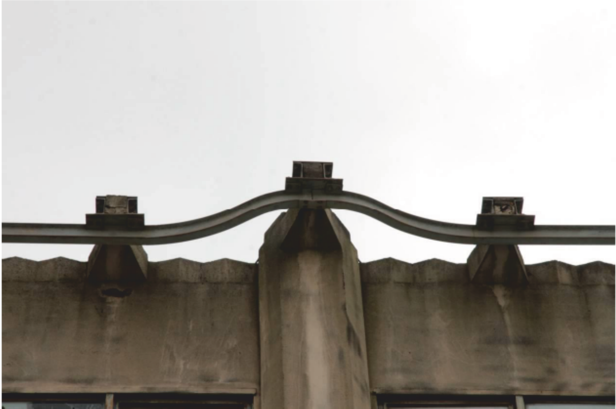
Plate 8 Chevron detail to parapet
