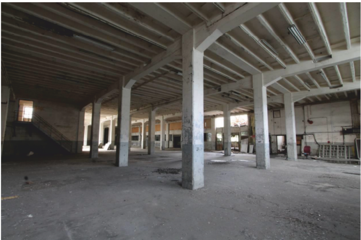
Plate 17 Ground floor, looking south-west
