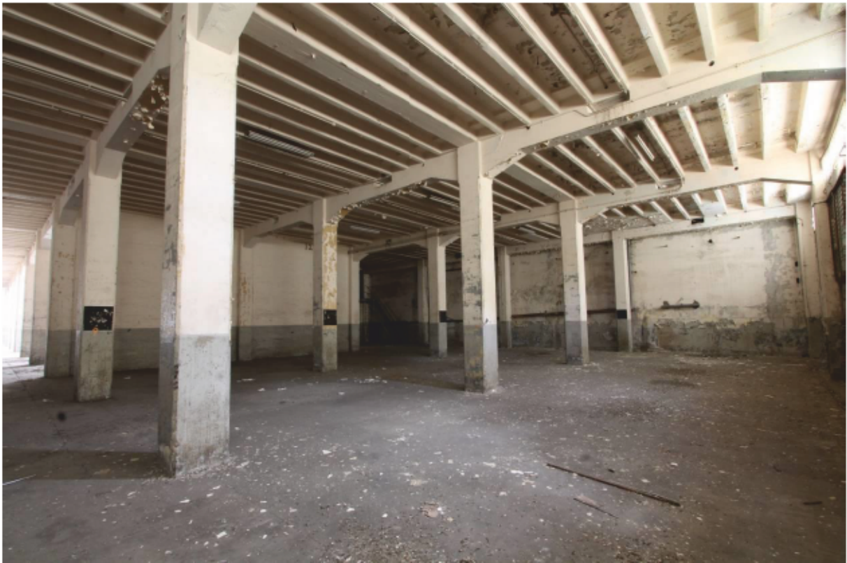
Plate 19 Ground floor, southern bays, looking north-east
