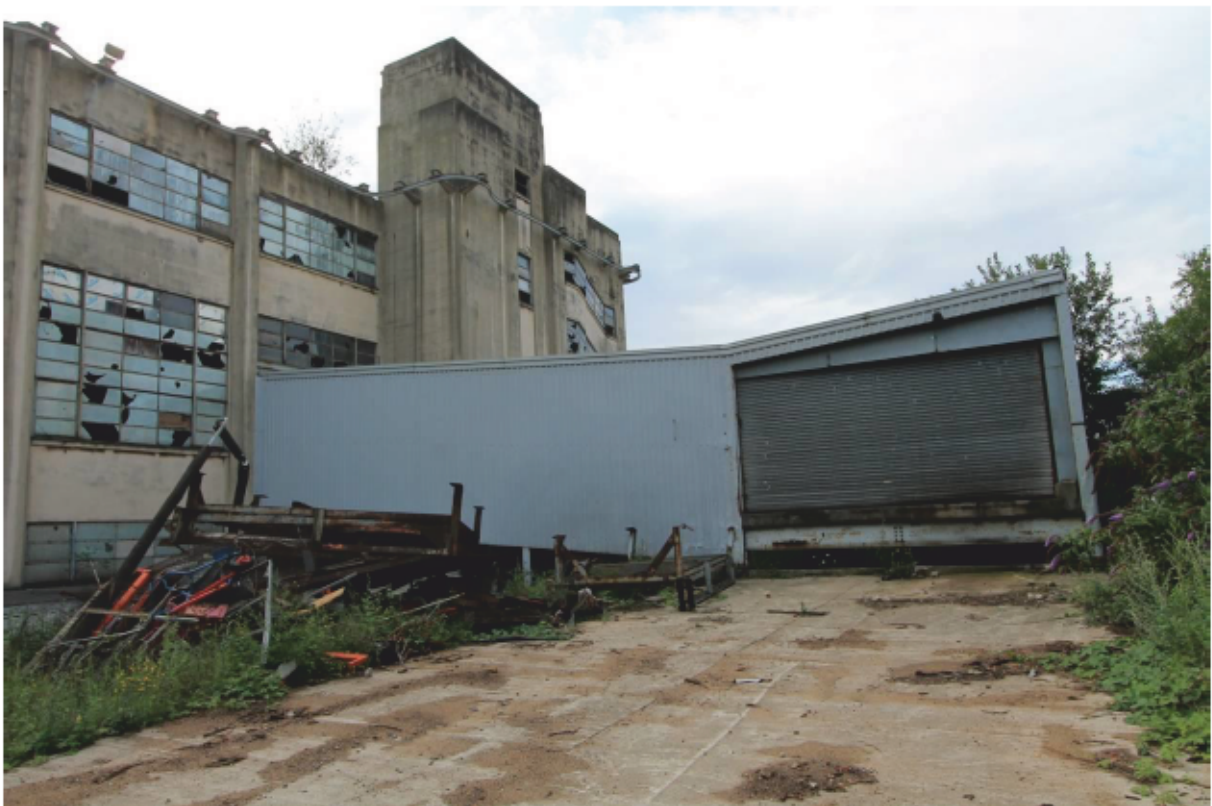
Plate 13 Modern (1972-1981) ramped loading bay on west side
