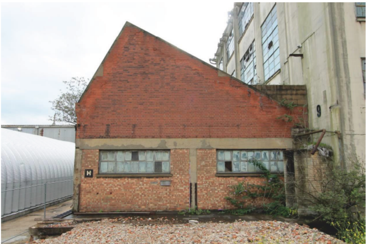
Plate 11 North-light northern extension
