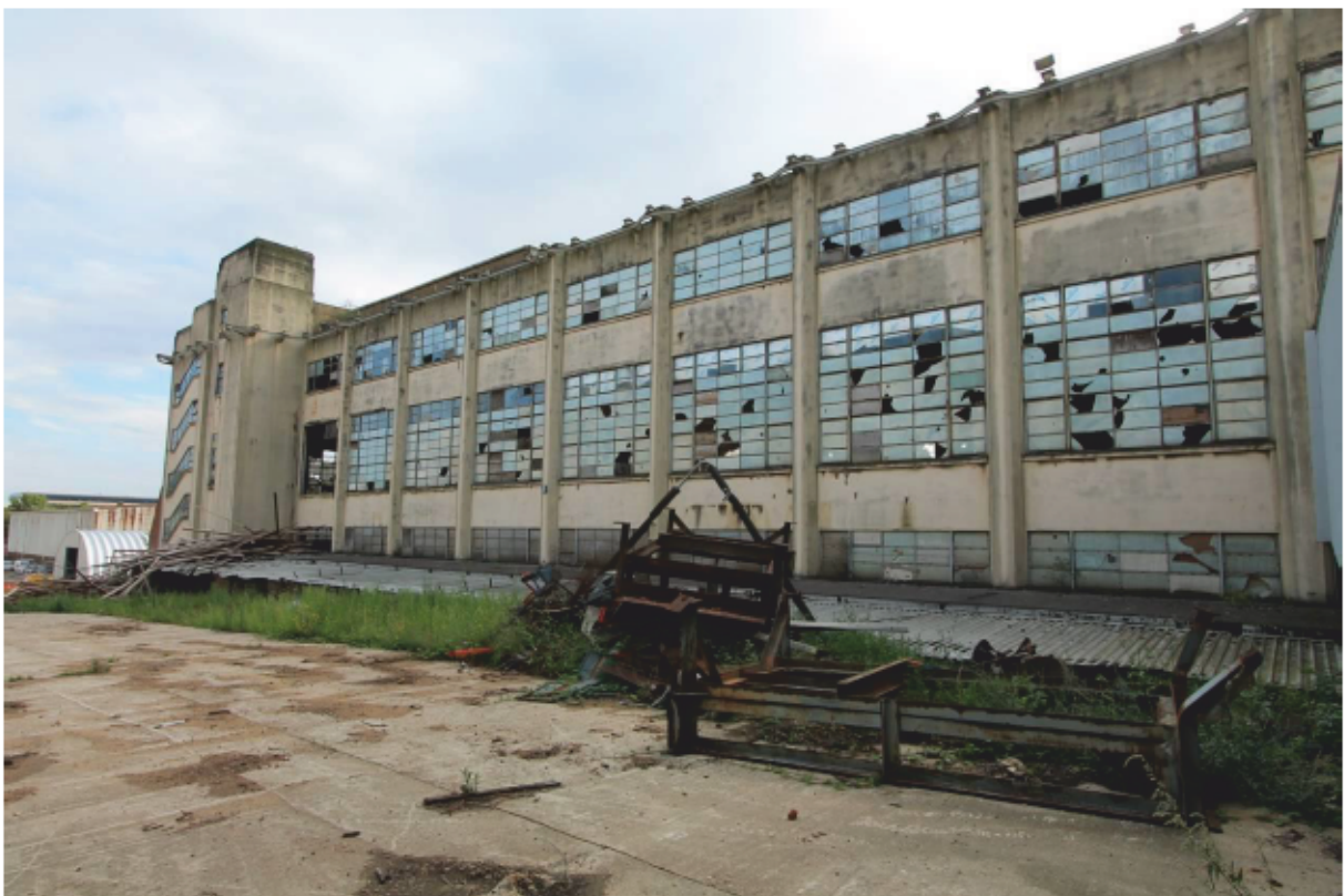
Plate 4 Unit 9 looking north-east
