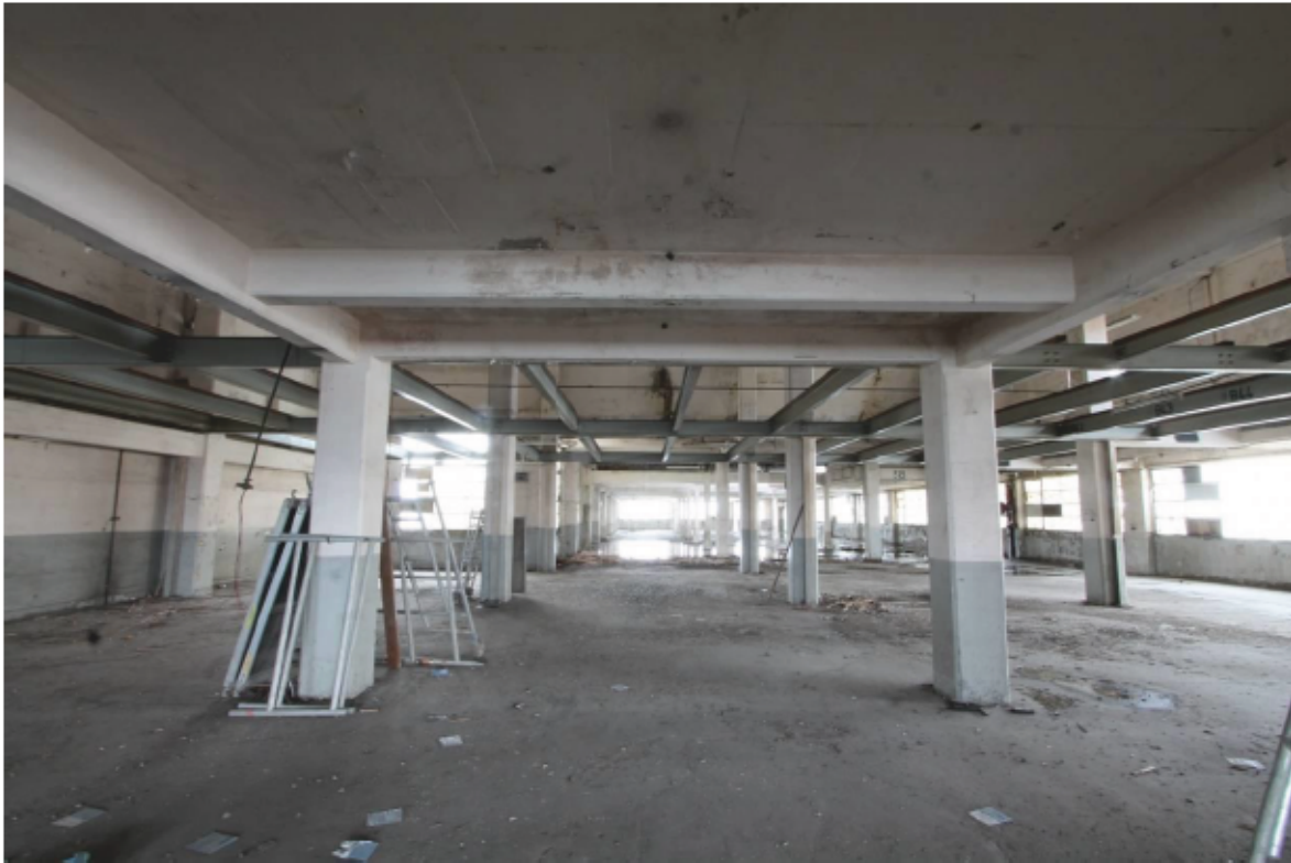
Plate 48 Second floor, northern bays, below mezzanine
