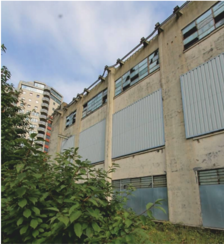
Plate 14 Southern elevation looking north-west
