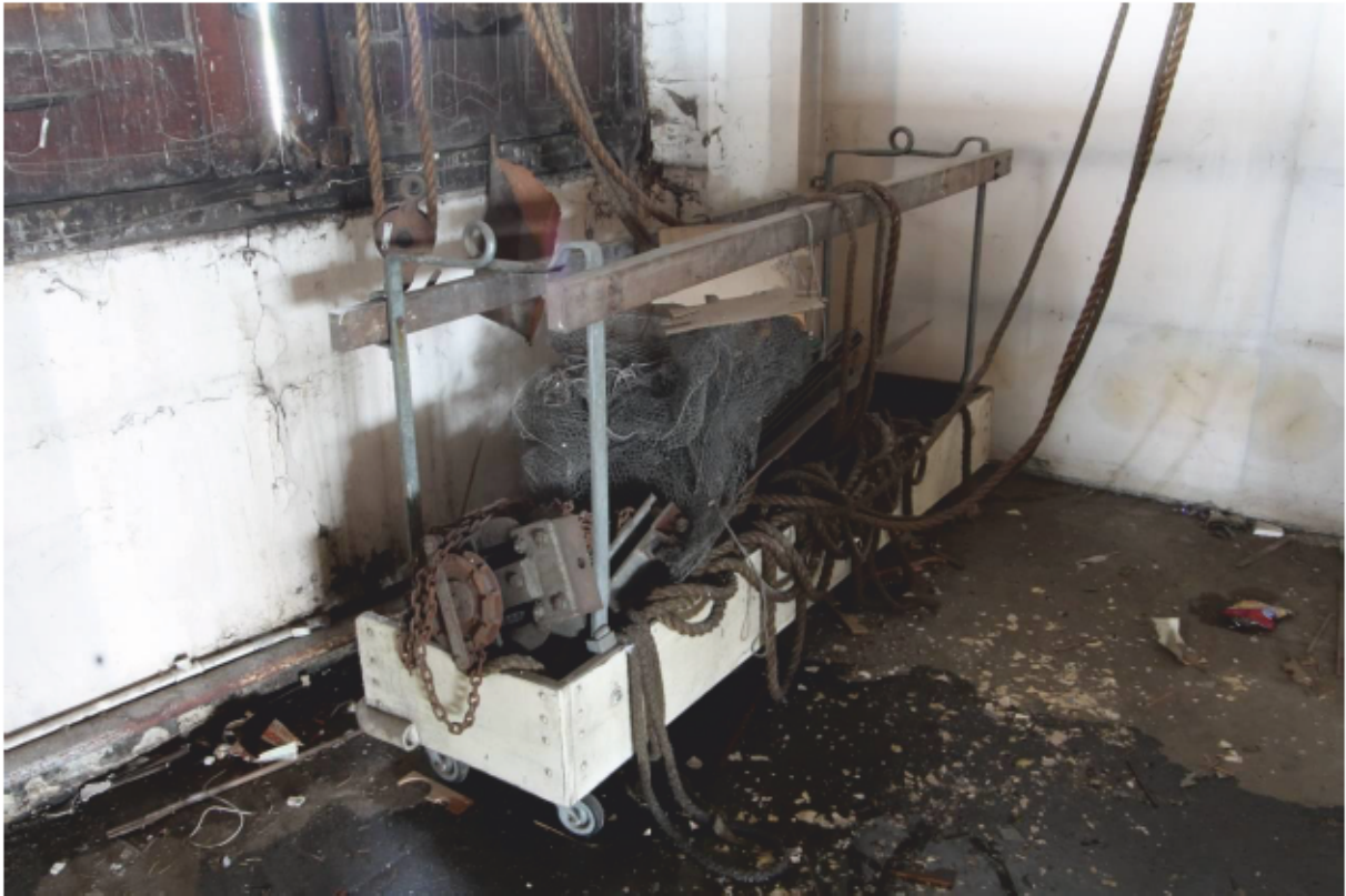
Plate 53 Cradle used for external works
