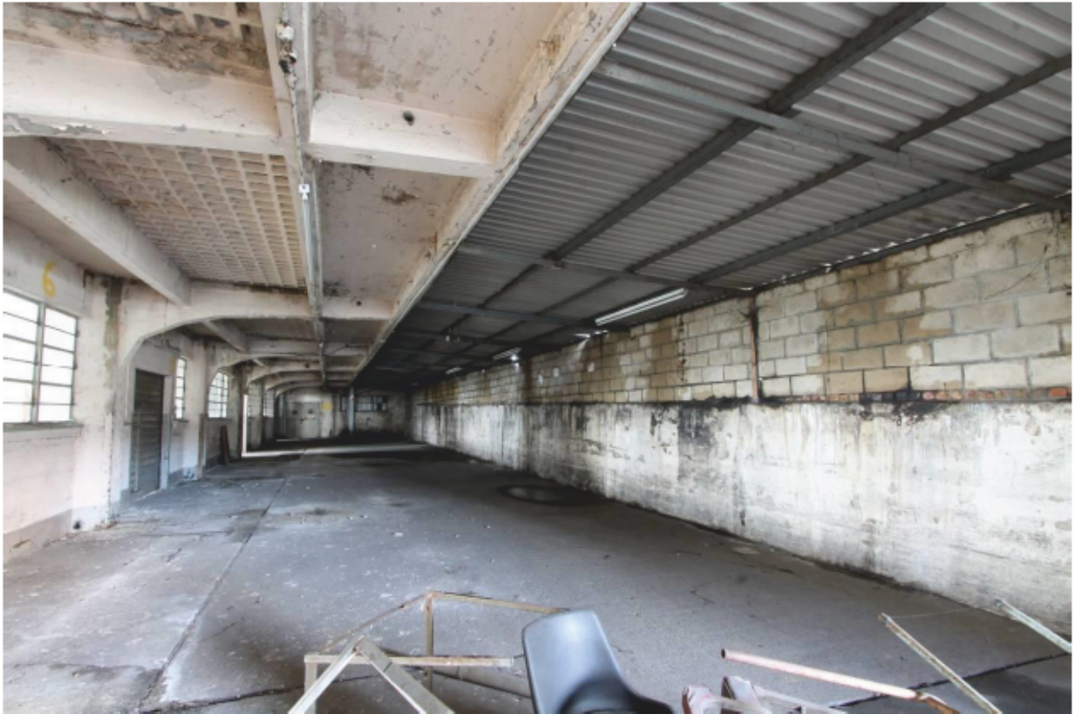
Plate 26 Western loading bay looking south
