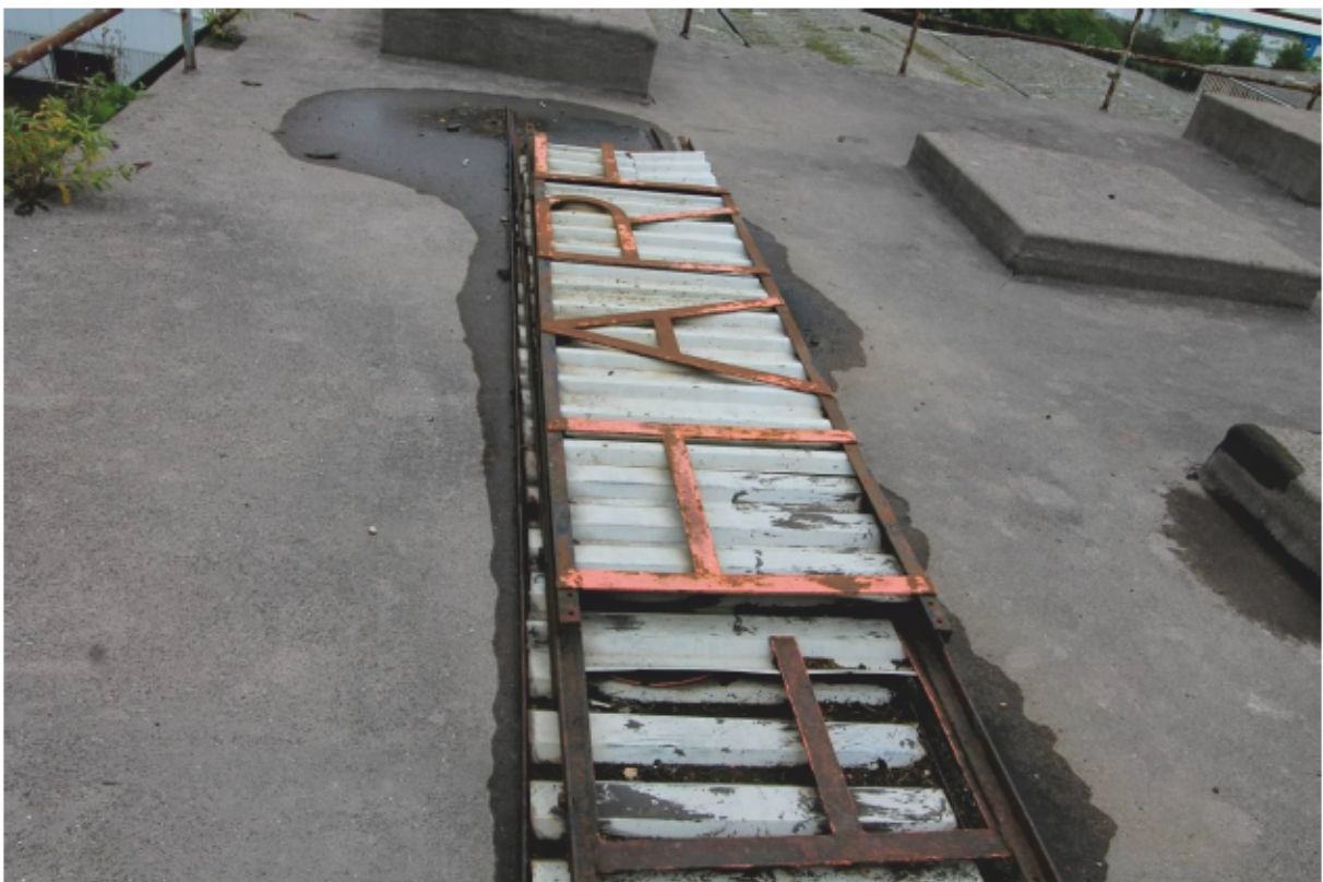
Plate 58 Former signage at roof level
