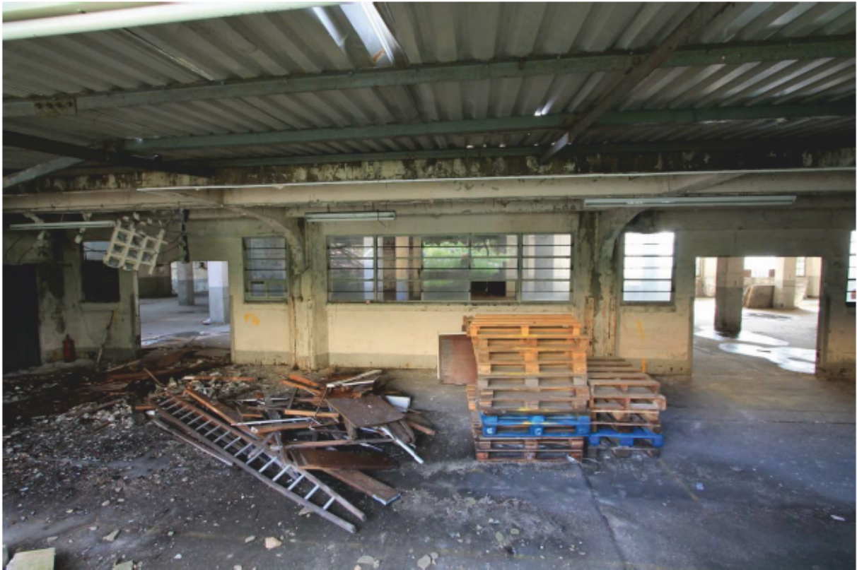
Plate 10 Western loading bay (viewed externally)
