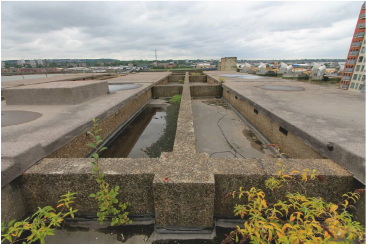
Plate 57 Flat roof over northern bays, looking south
