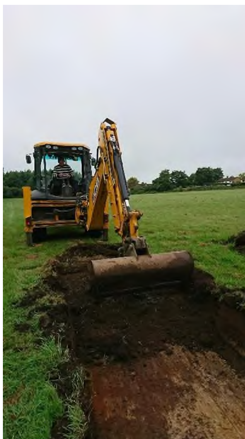
Plate 2: Trench 3 mid excavation, looking northwest
