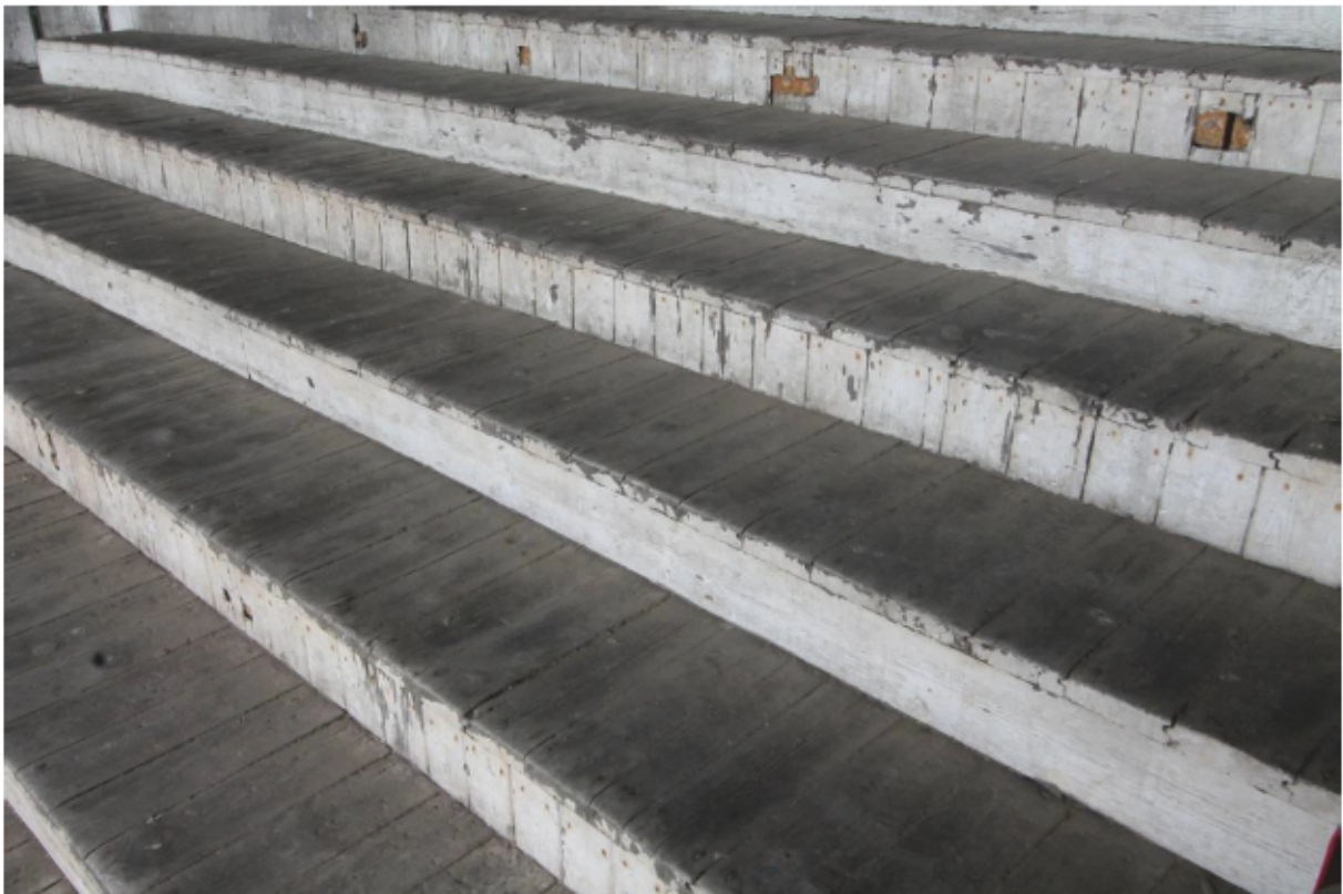
Plate 24 Original timber terraces
