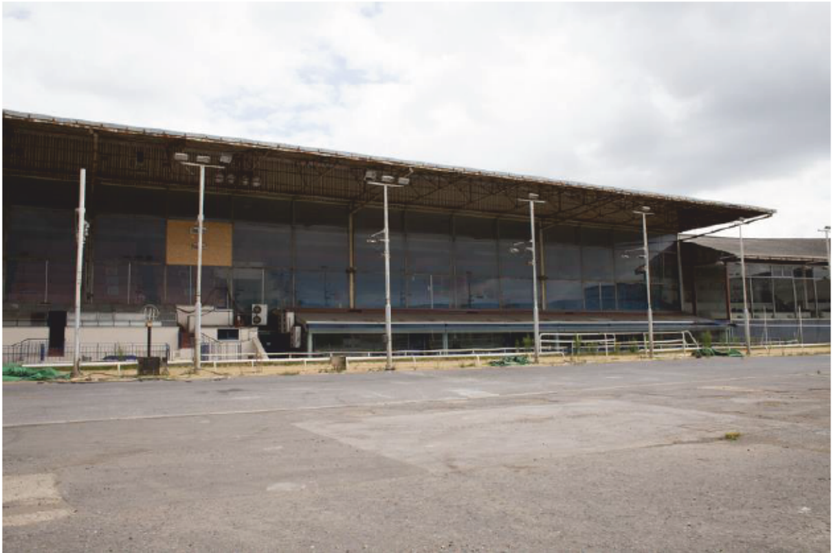
Plate 17 Main East Grandstand looking south-east
