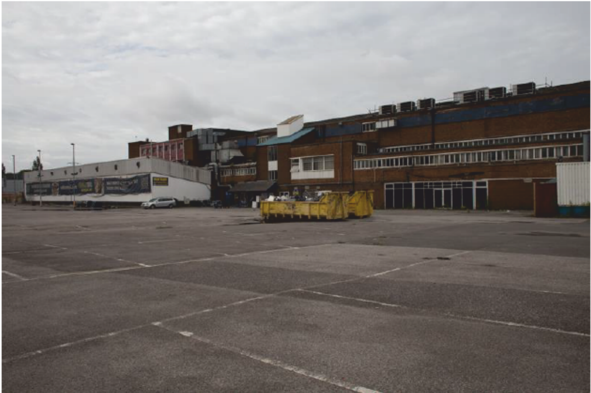
Plate 3 Main East Grandstand (right and centre) and Squash Club (left), looking south-west
