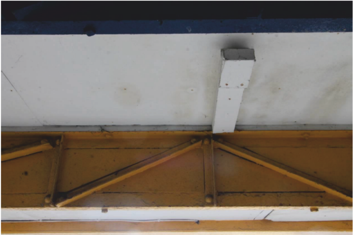
Plate 25 Detail of triangulated steel riser forming terrace
