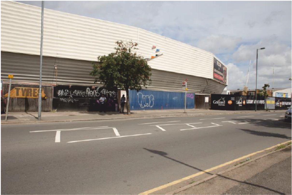
Plate 13 Rear of stands backing onto Plough Lane
