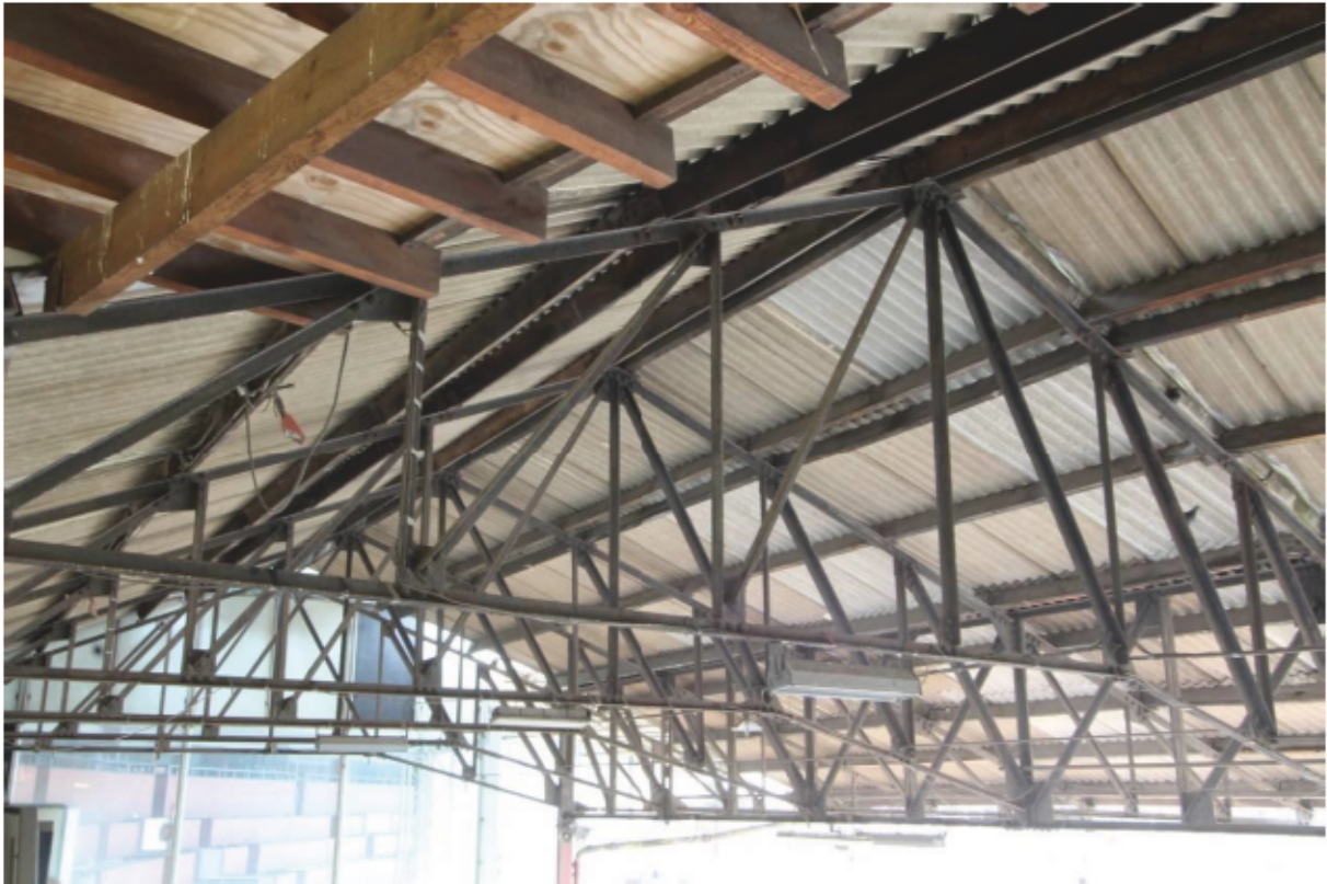
Plate 27 Original triangulating roof trusses
