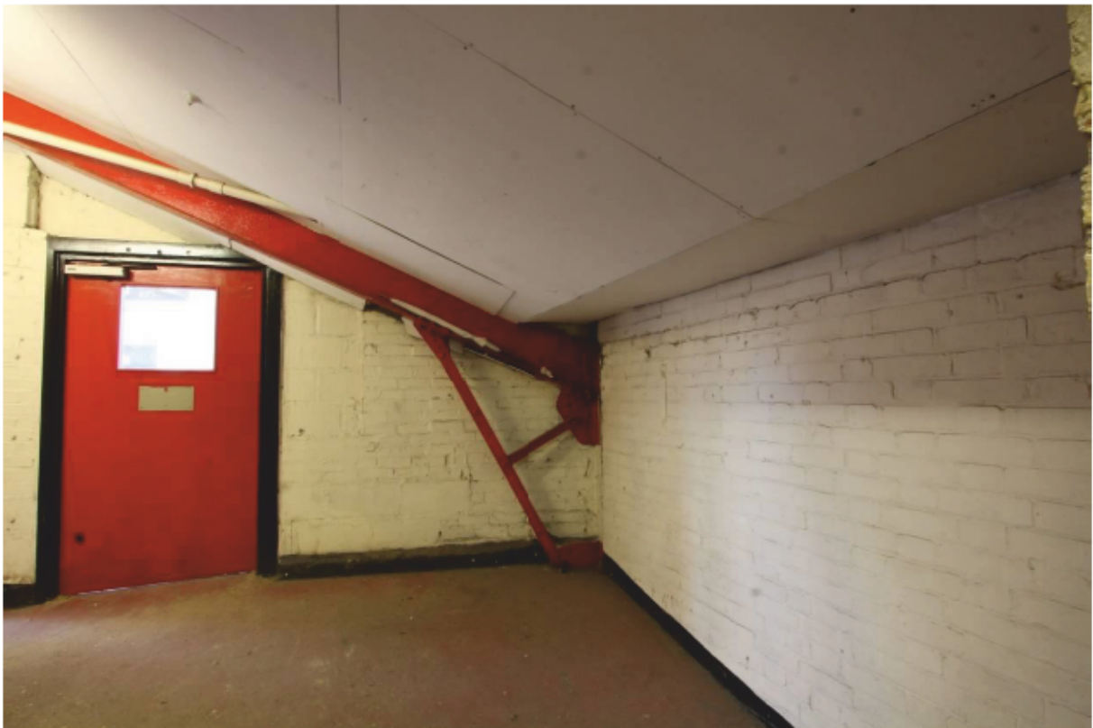
Plate 48 Steel structure supporting terracing (G12)
