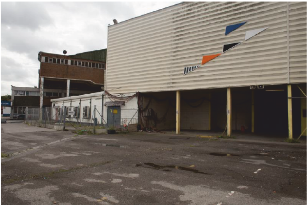
Plate 10 View to kennels (white building) and Main Grandstand
