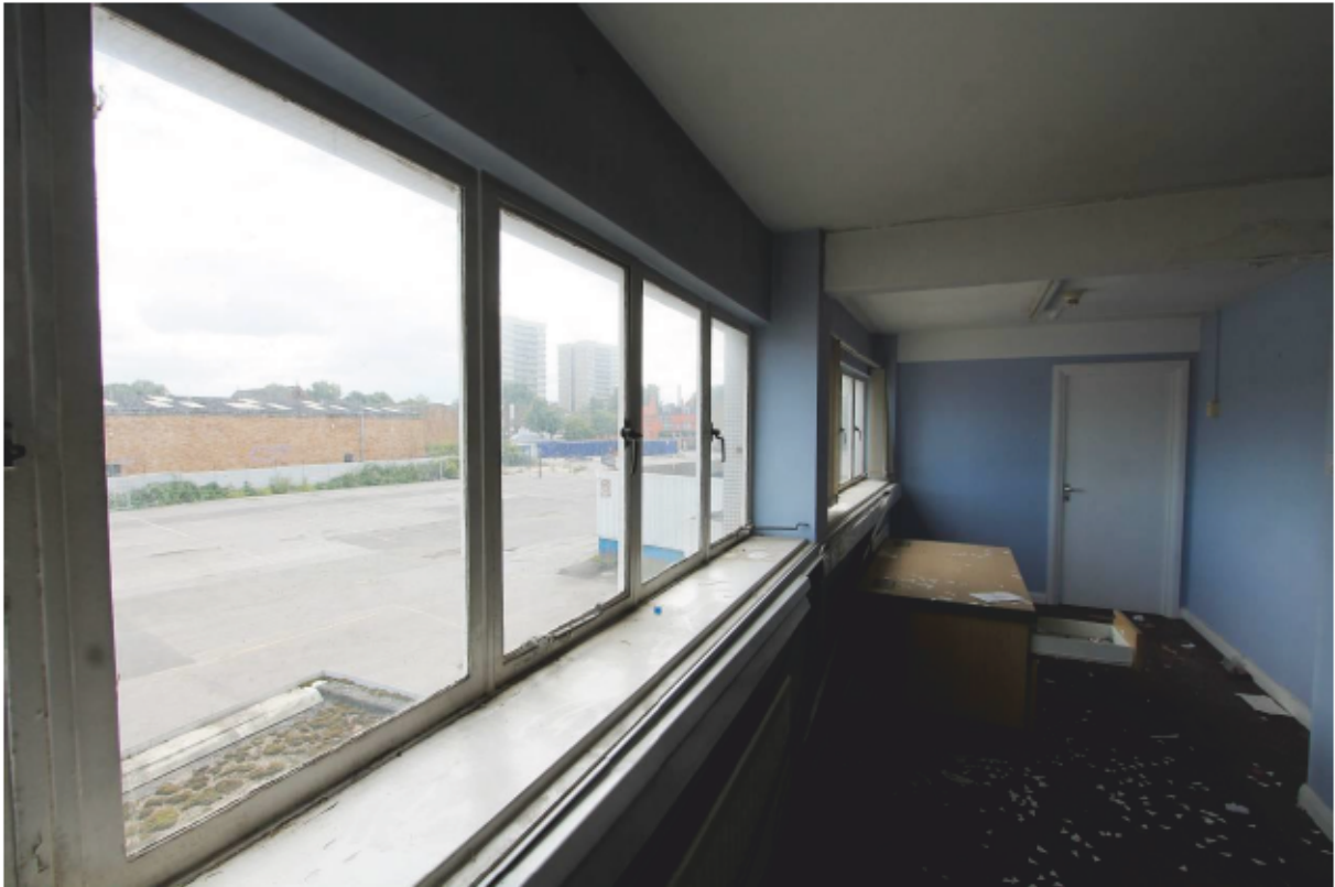
Plate 57 Typical office (F8) showing strip glazing
