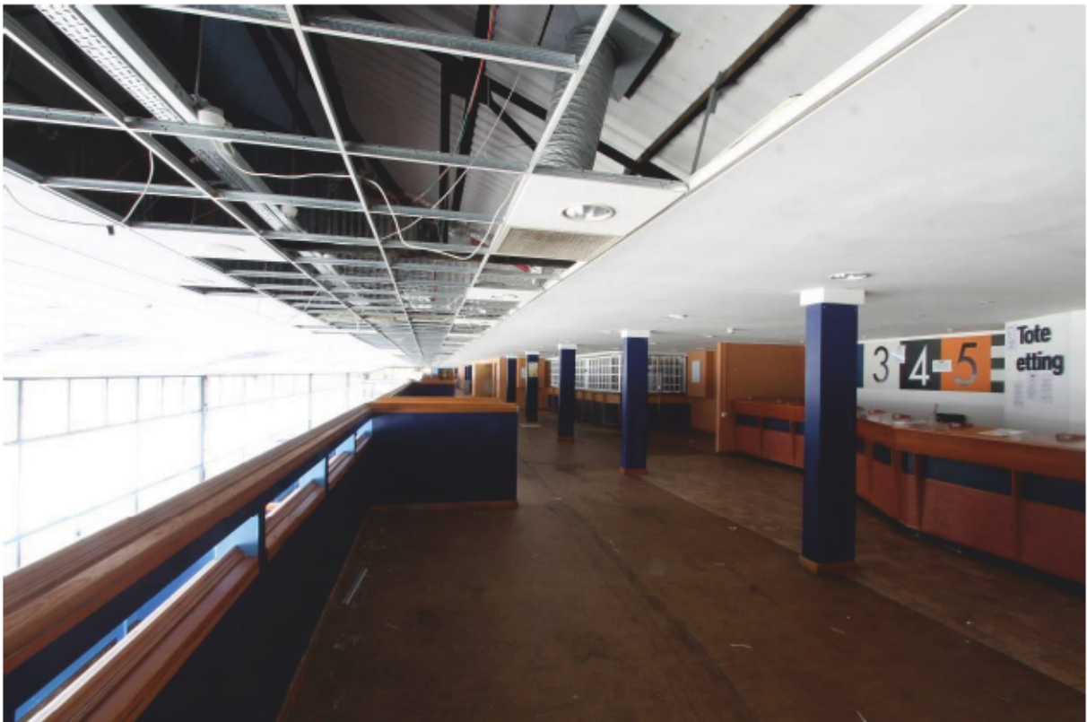
Plate 66 Bar area at first floor (F12), looking south
