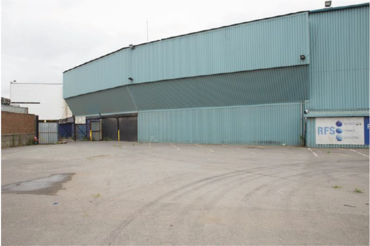
Plate 11 Rear of northern stands, looking south-east
