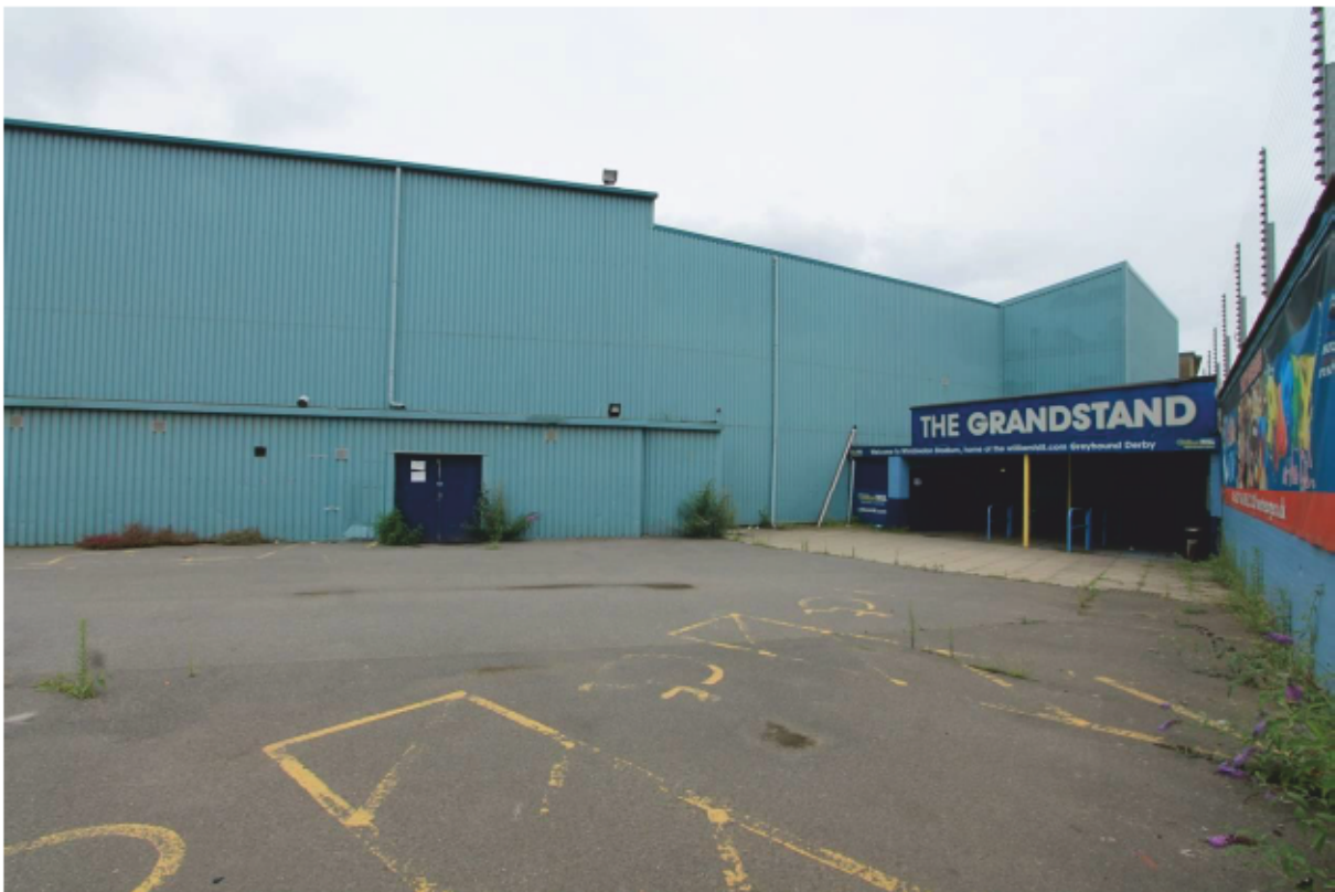
Plate 12 Rear of northern stands, looking towards turnstiles to West Grandstand
