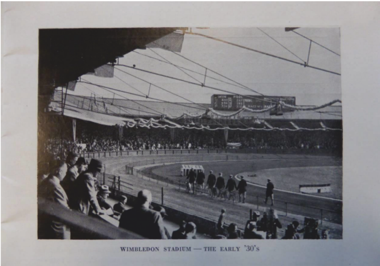
Historic Plate D: View of stadium looking south, taken in the early 1930s
