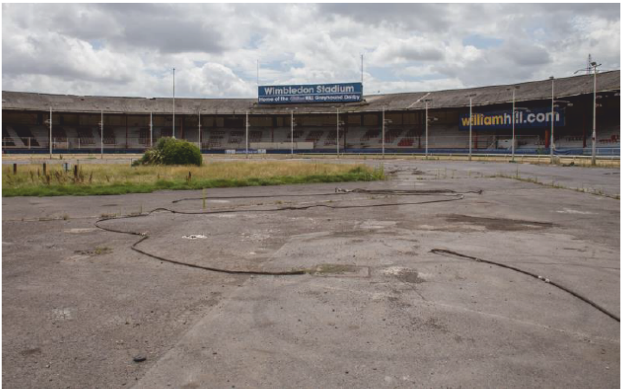
Plate 20 South stands looking south
