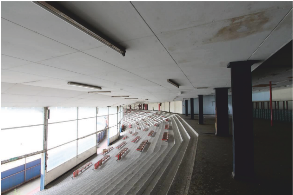
Plate 74 Terrace at rear of northern stand, showing glass partition wall (S6)
