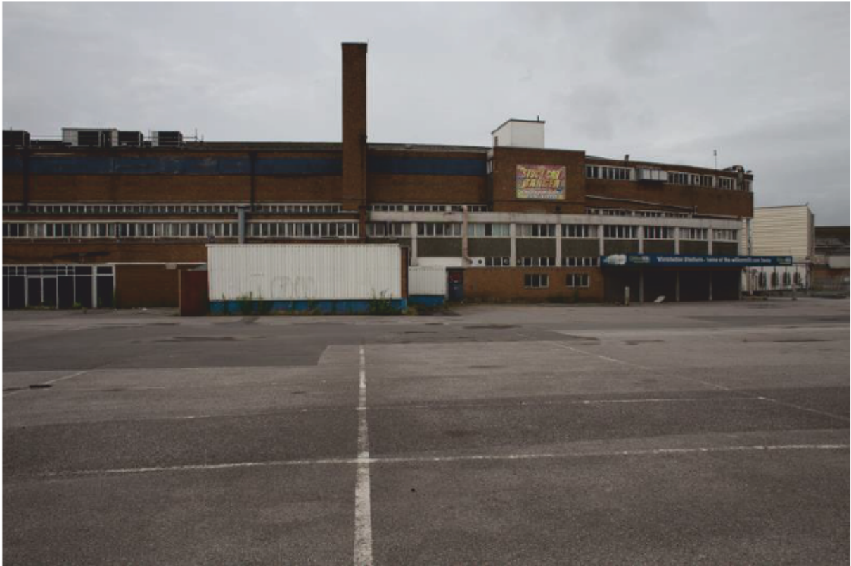
Plate 5 Main East Grandstand, northern bays, looking west
