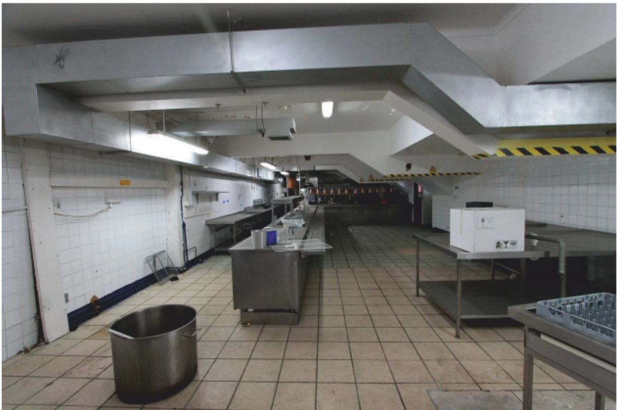
Plate 56 Kitchens (F10) on first floor of main East Ggrandstand
