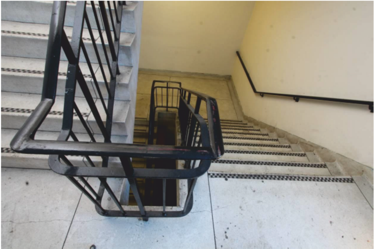
Plate 39 Open-well stair (G26) with Terrazzo treads
