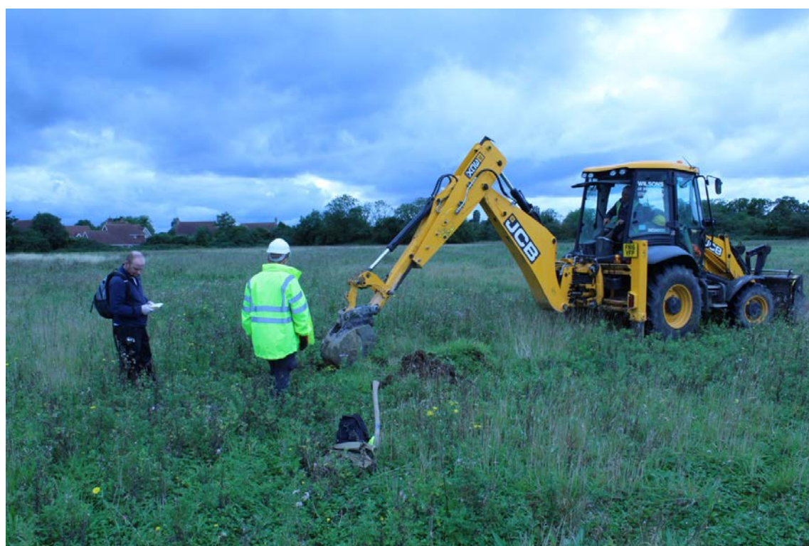
Plate 2: Machine excavation of trial trench, facing south
