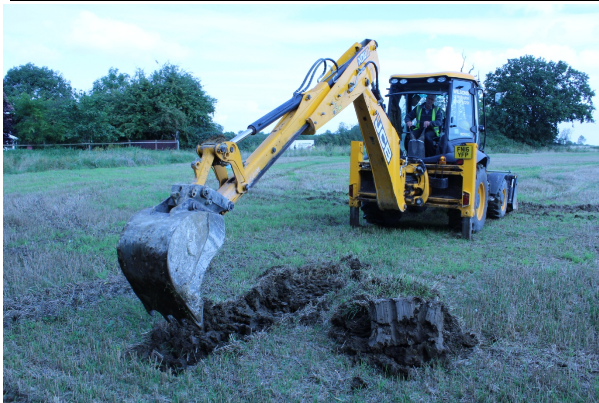
Plate 3: Machine excavation of trial trench, facing north-west
