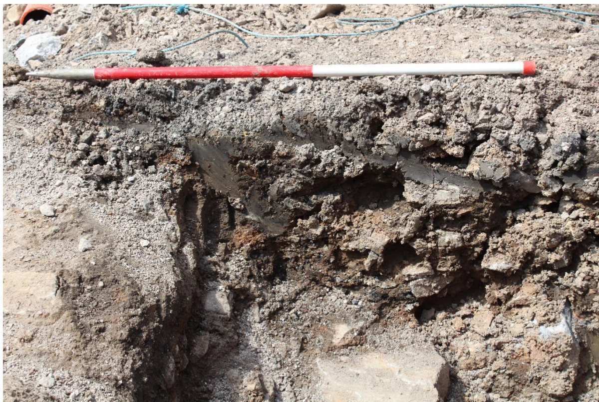
Plate 8, Photo of robber cut [1168] effecting the Portwall (1166) within the district heating main trench.
