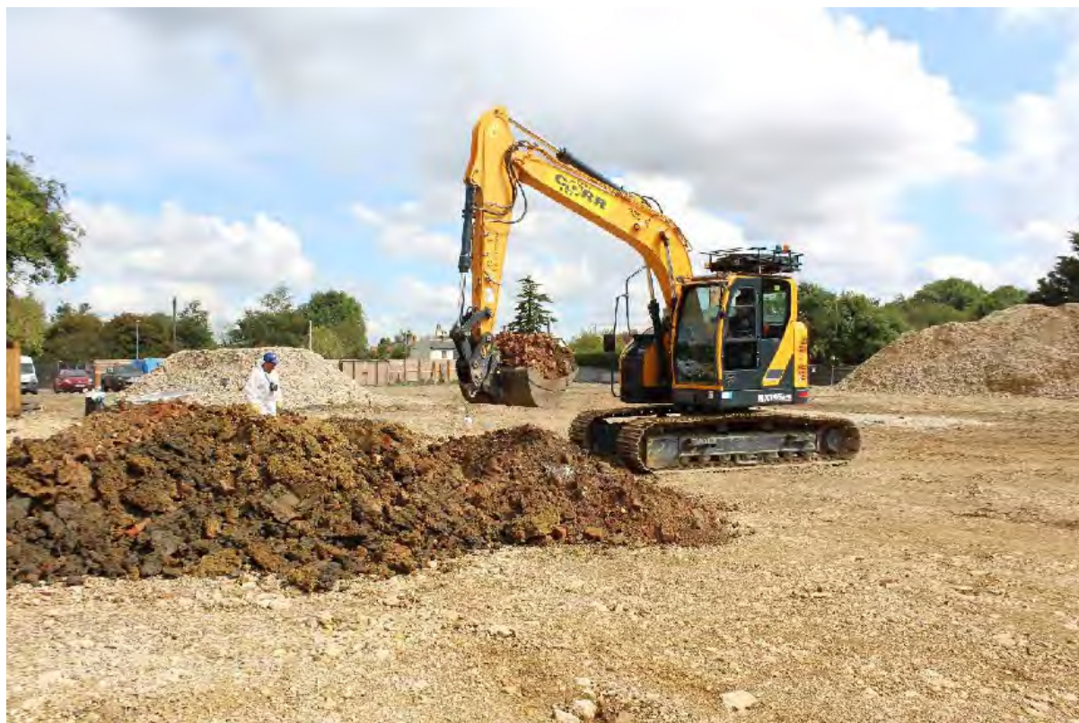
Figure 2 Machining on site looking northeast
