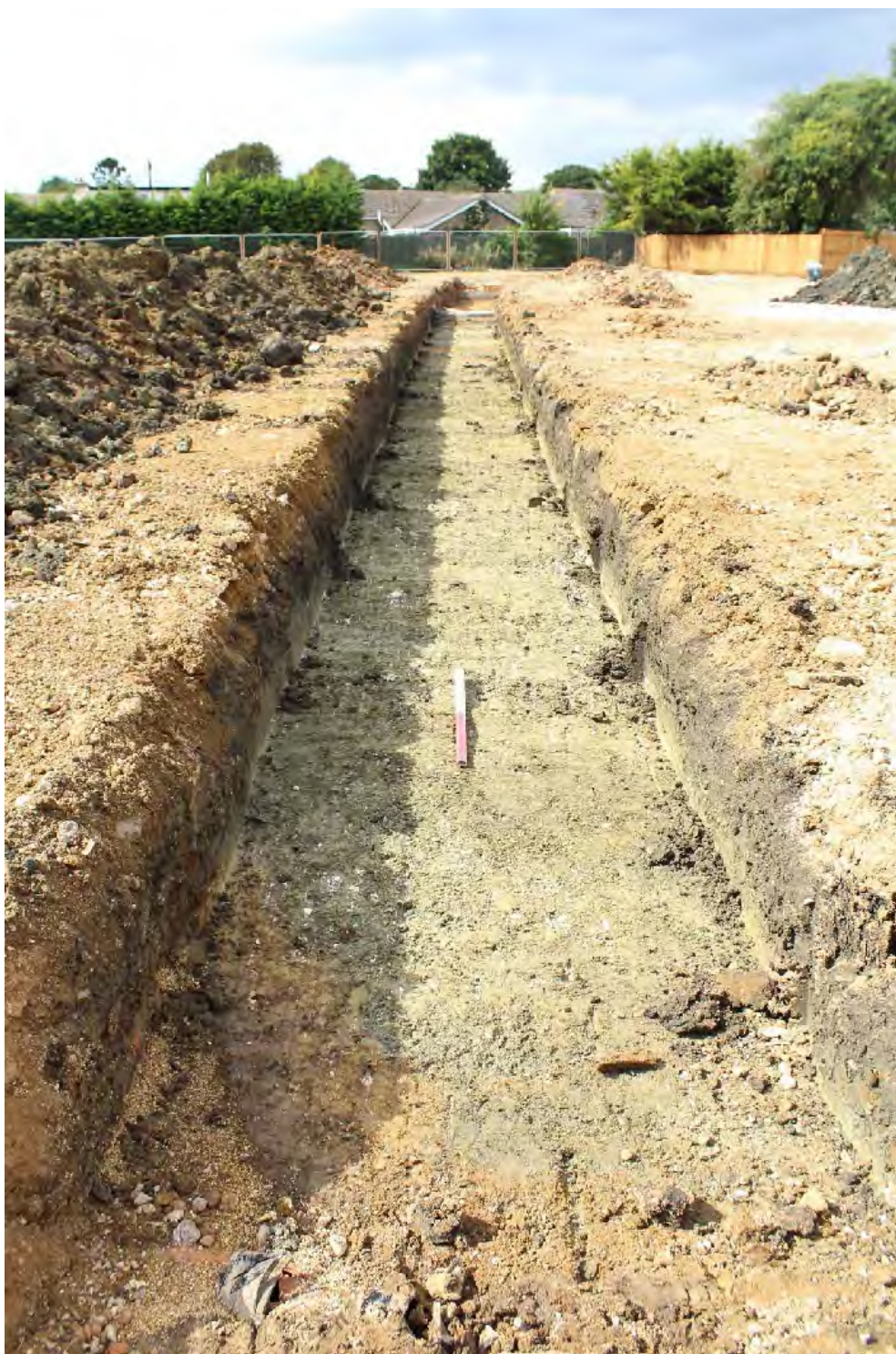
Figure 3 Trench 2, looking northwest
