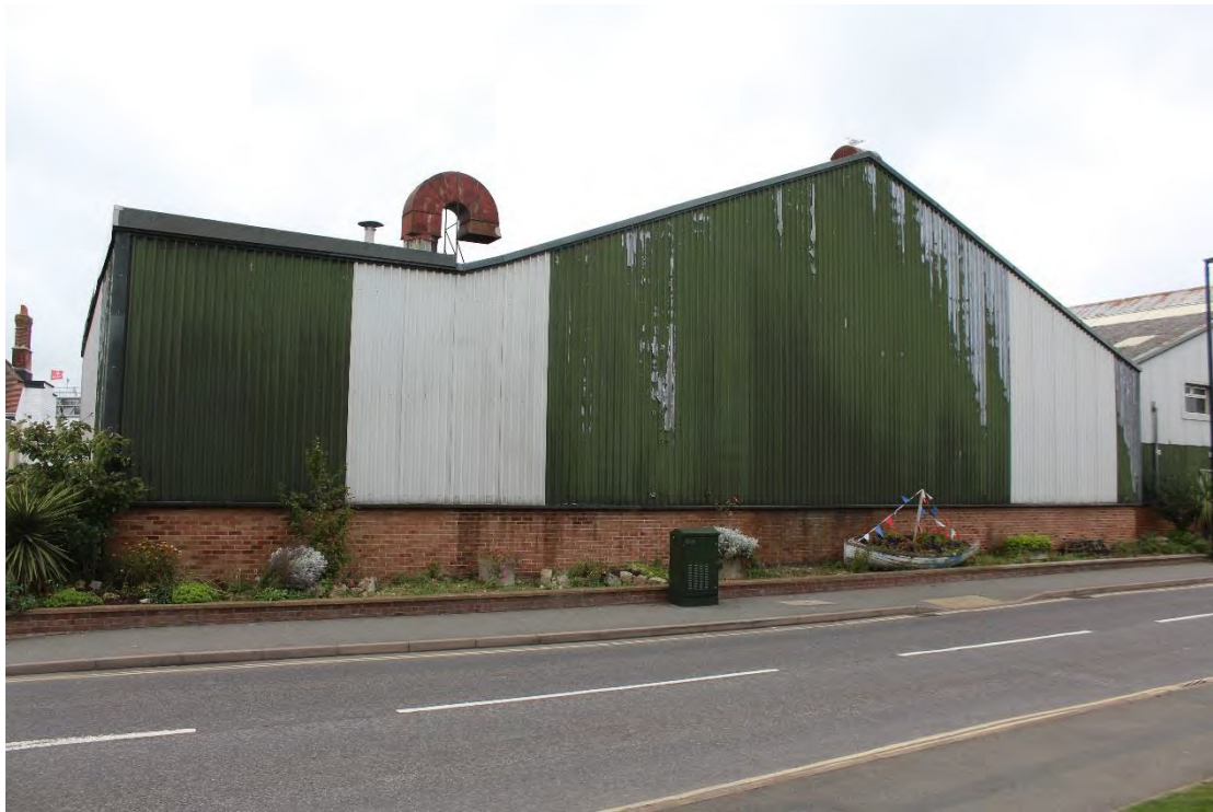
Plate 5. East elevations of Buildings 2 & 3 of the Redux Sheds.
