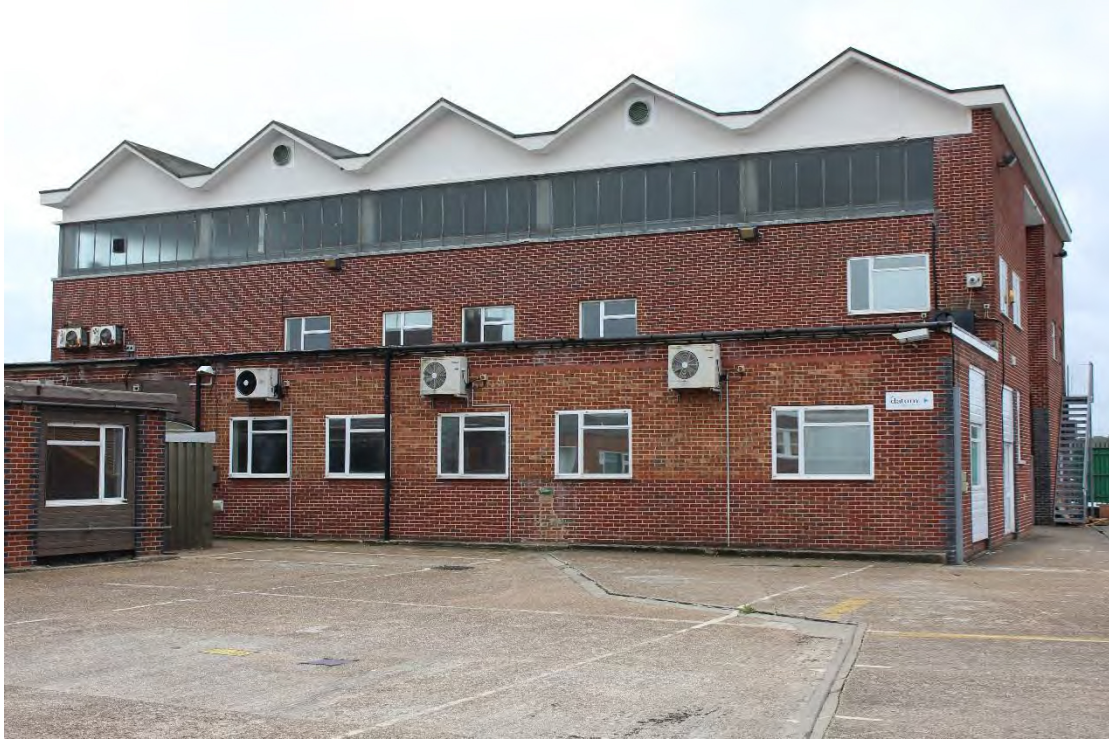
Plate 17. Northern elevation of Building 9 at Trinity House Depot.
