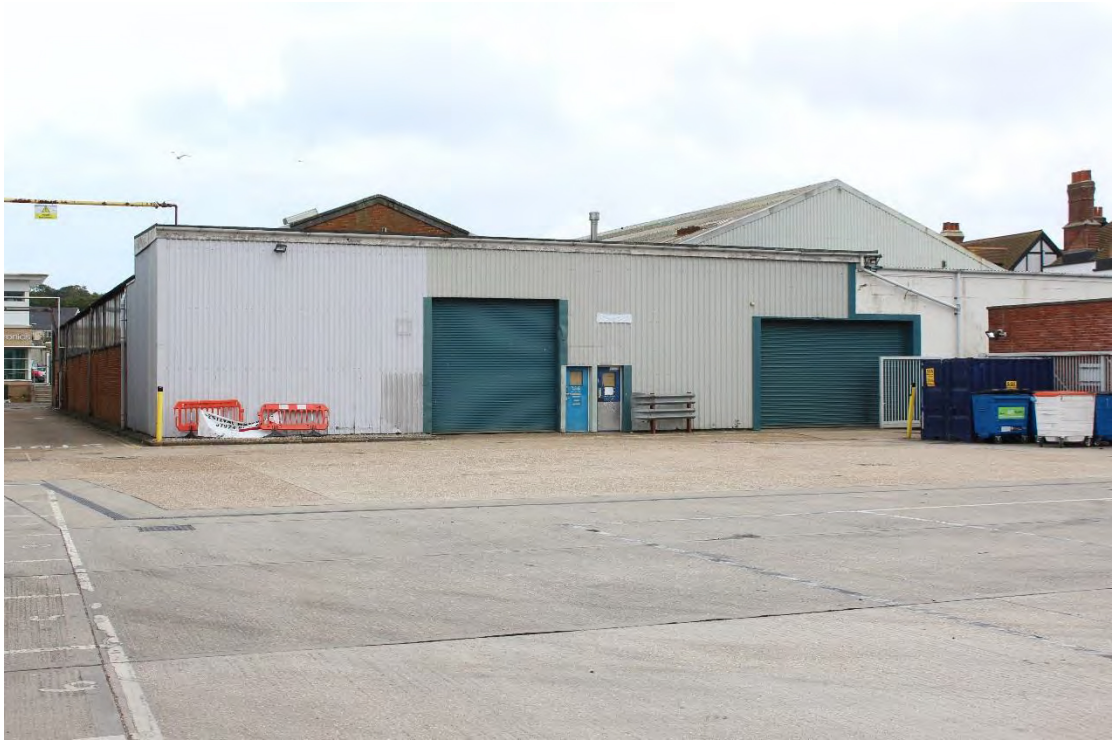
Plate 1. West elevations of Buildings 1, 2 & 5 of the Redux Sheds.
