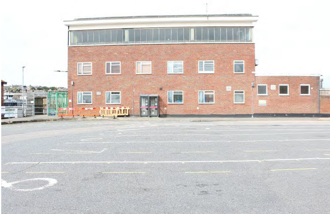
Plate 15. Eastern elevation of Building 9 at Trinity House Depot.
