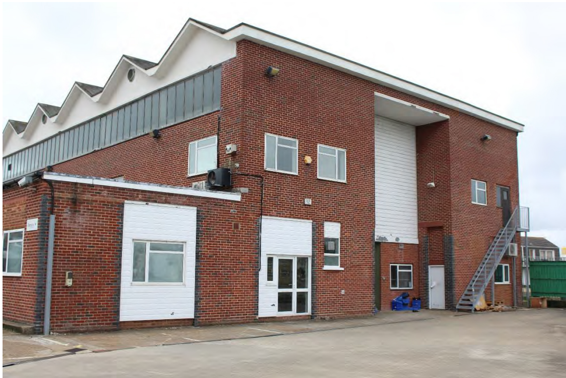
Plate 18. Western elevation of Building 9 at Trinity House Depot.
