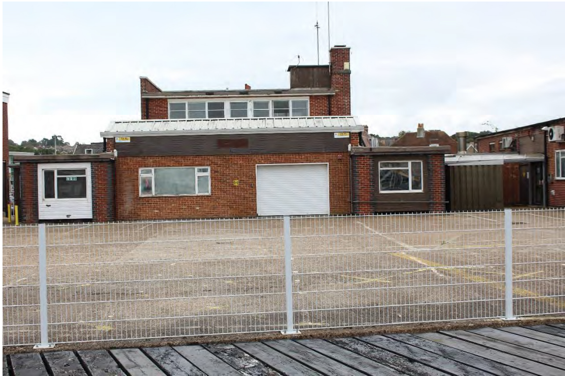
Plate 13. Western elevations of Buildings 7 and 8 at Trinity House Depot.
