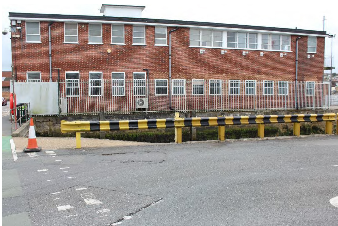
Plate 10. Northern elevation of Building 6 (St Catherines Building) at Trinity House Depot.
