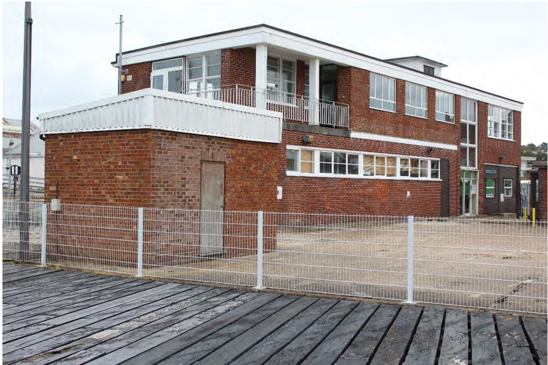
Plate 7. Oblique view of south elevations of Buildings 6 (right) and 10 (left) at Trinity House Depot
