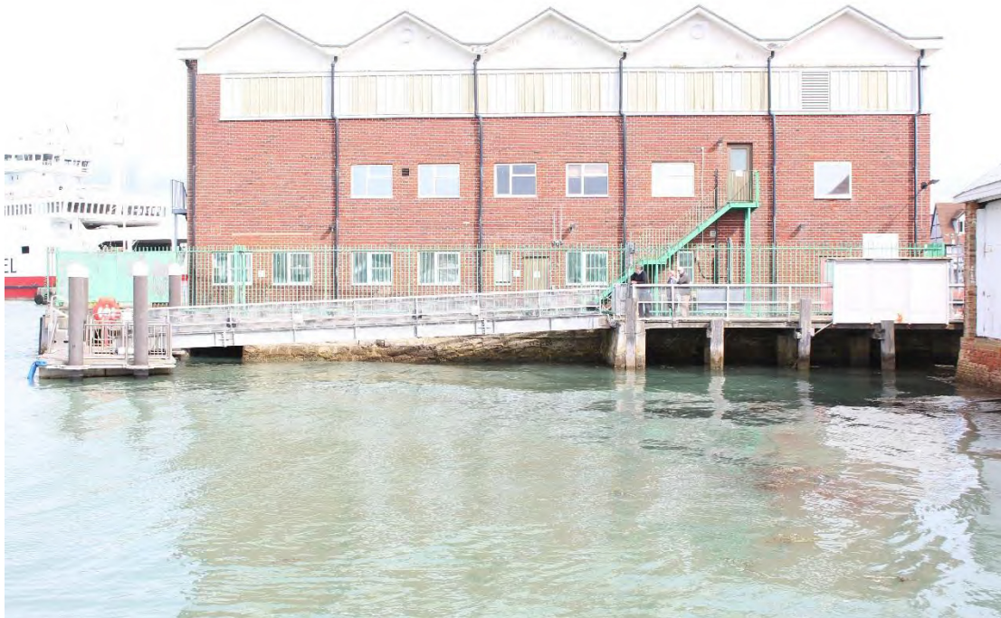
Plate 16. Southern elevation of Building 9 at Trinity House Depot.
