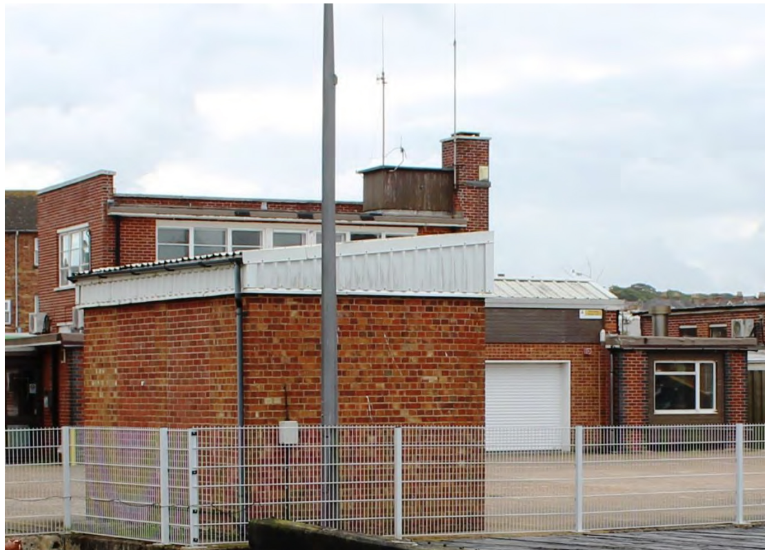
Plate 12. Western elevations of Building 7, 8 (background) and 10 (foreground) at Trinity House Depot.
