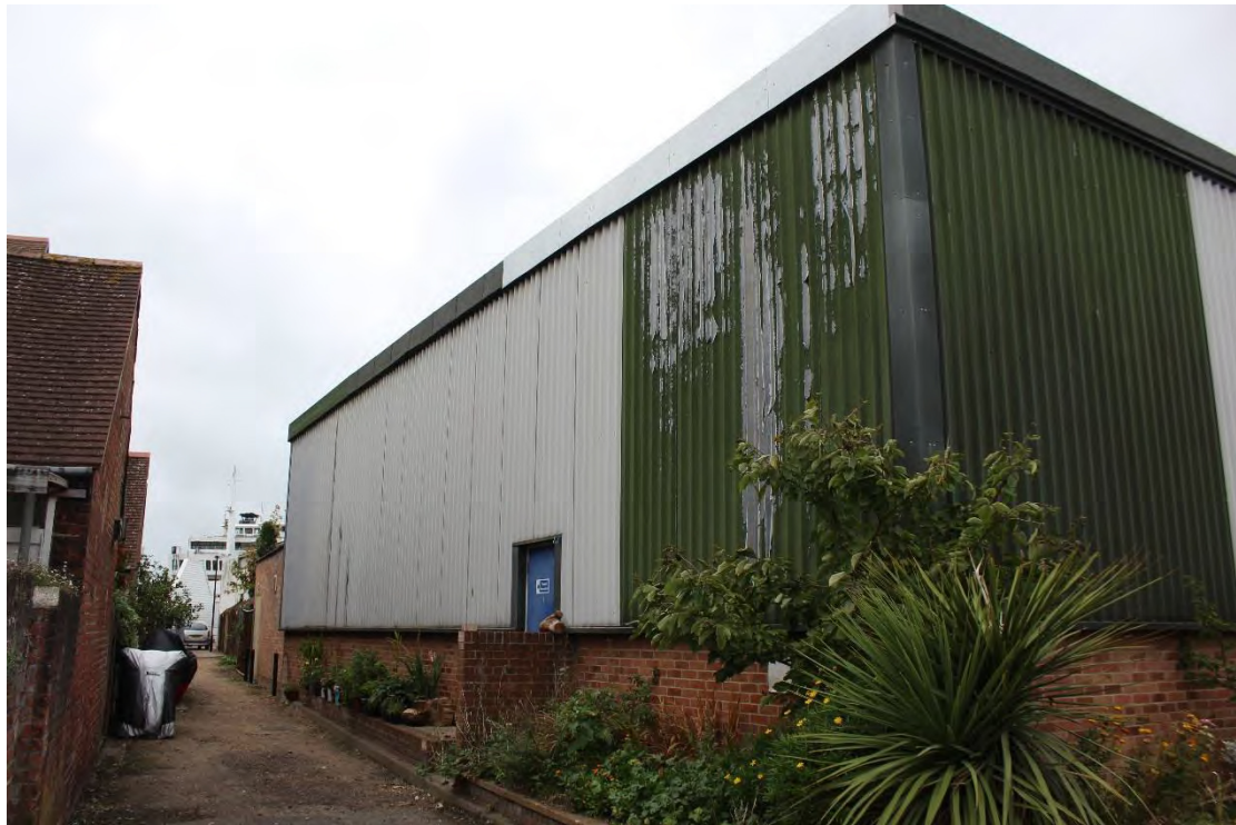
Plate 6. Oblique view of south elevations of Buildings 3 & 4 of the Redux Sheds.
