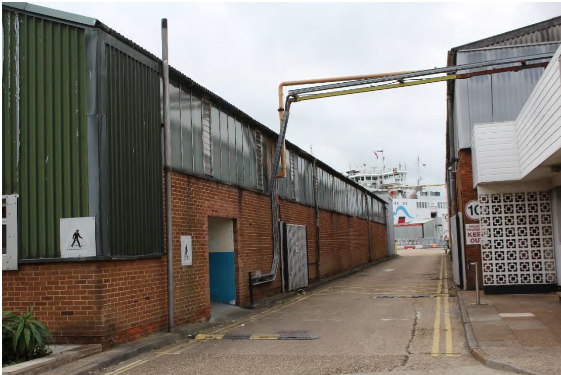
Plate 3. Oblique view of north elevation of Building 1 of Redux Sheds looking west.
