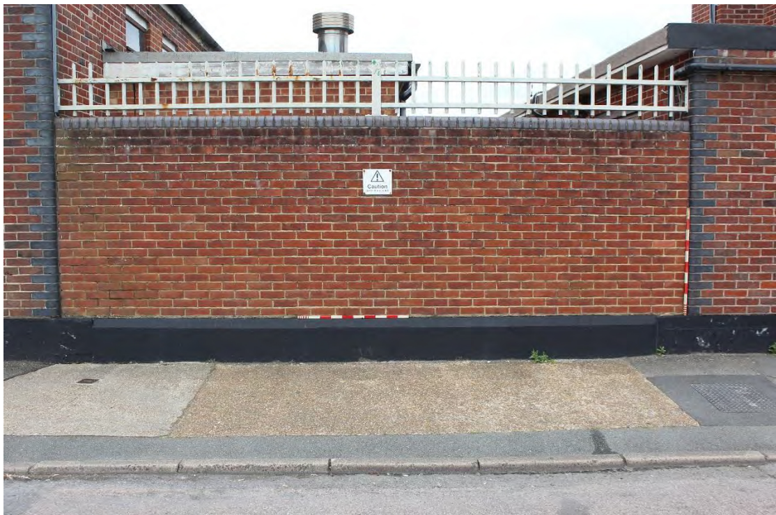
Plate 14. East-facing brick infill wall between Buildings 7 and 9 at Trinity House Depot.
