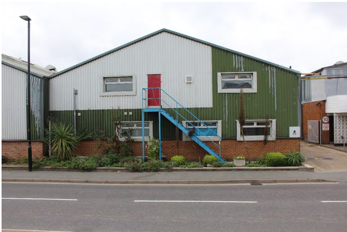
Plate 4. East elevation of Building 1 of the Redux Sheds.
