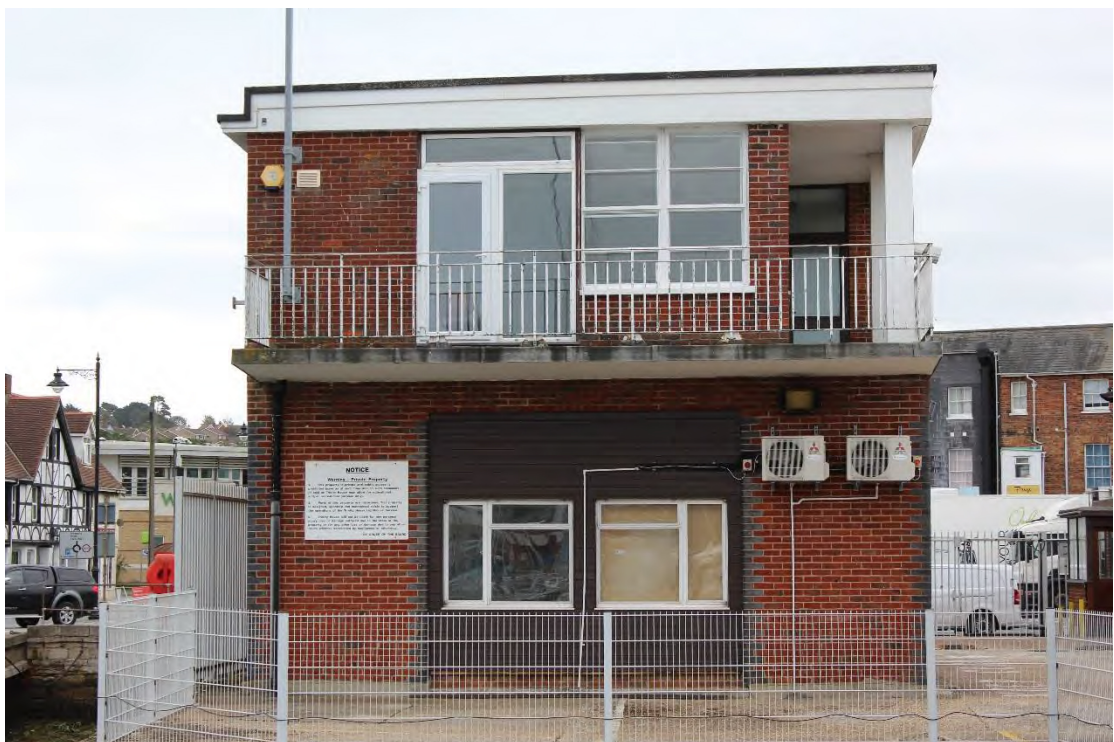
Plate 8. Western elevation of Building 6 (St Catherines Building) at Trinity House Depot.
