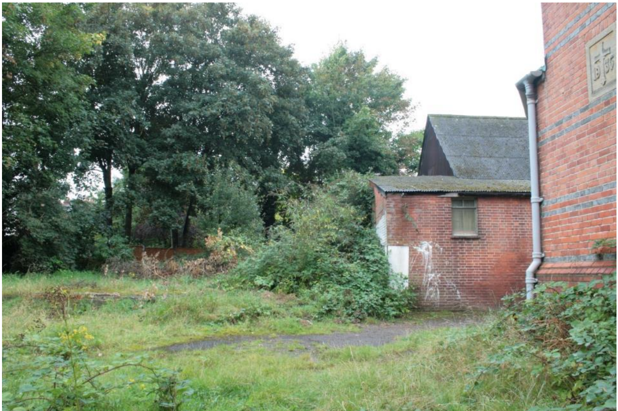
Plate 4: Concrete platform (left) and brick extension to the hall, looking south
