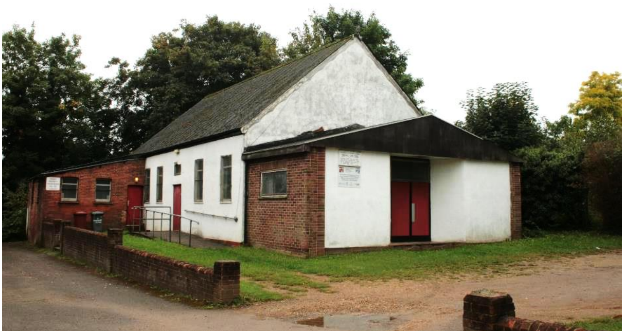
Plate 2: St George's Hall, looking south-east
