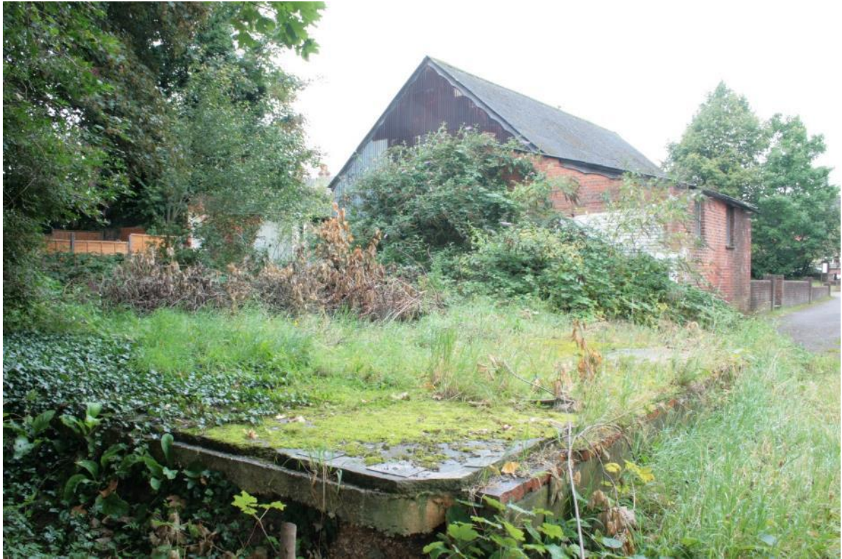
Plate 3: Concrete platform at rear (east) of hall, looking west
