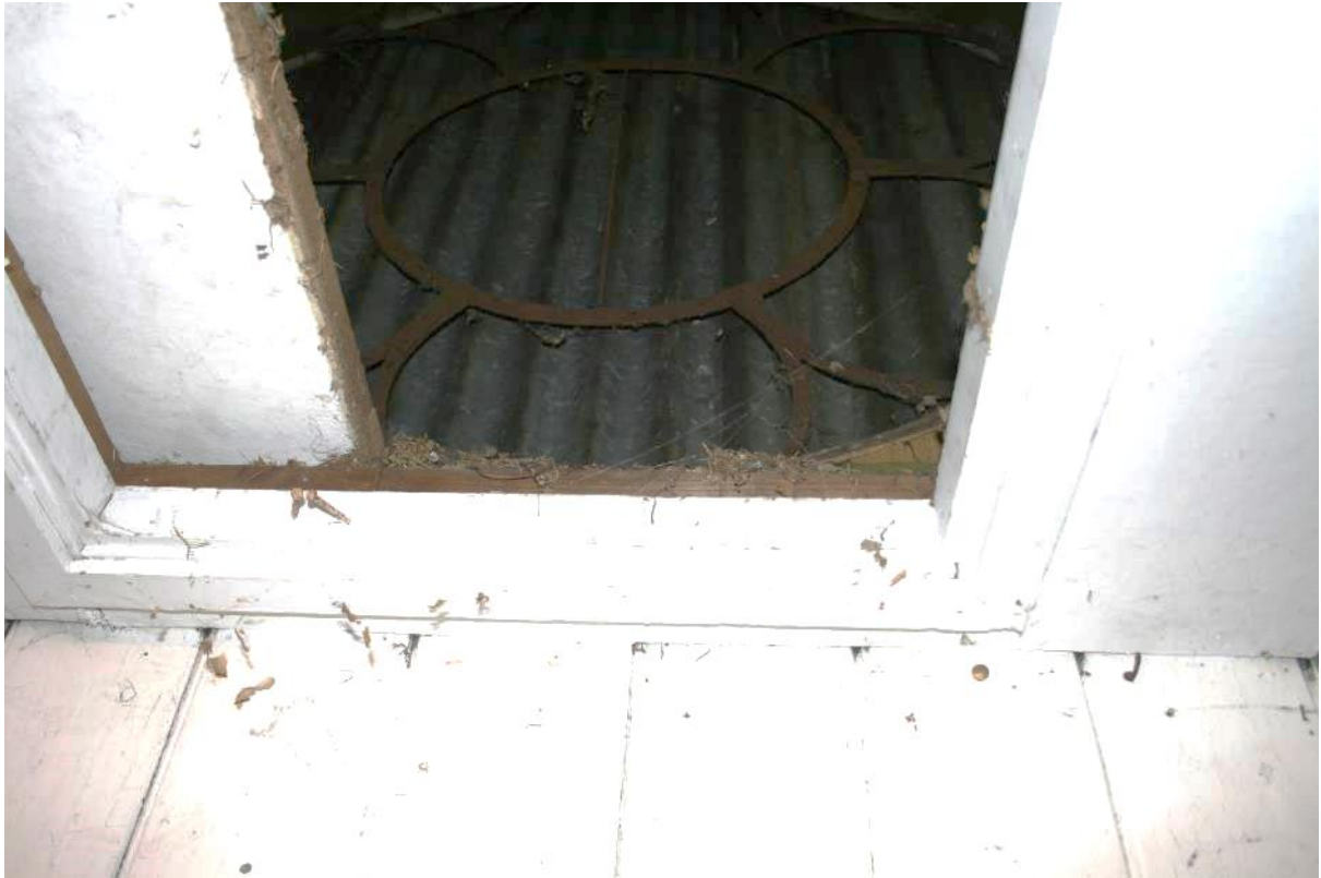
Plate 42: Access hatch to roof space above stage, looking east
