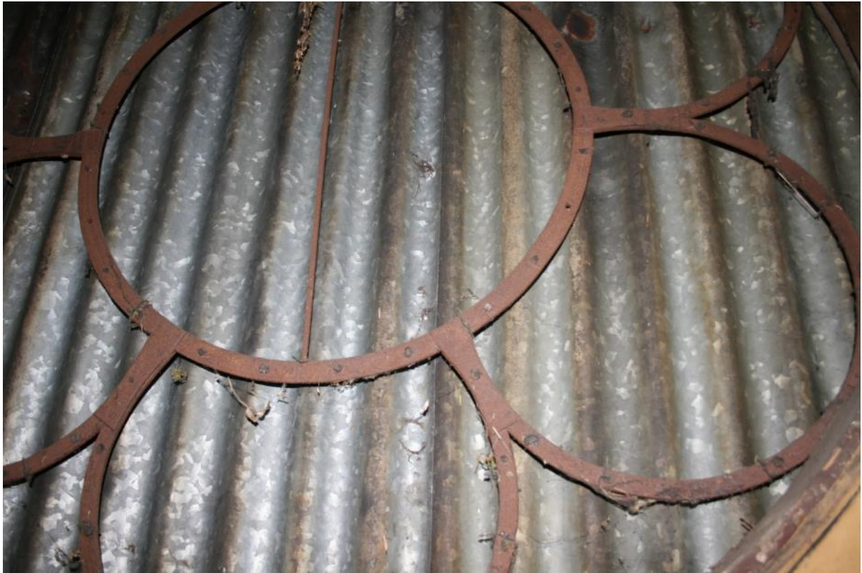
Plate 44: Original rose window in the east gable of the Iron Church, looking east
