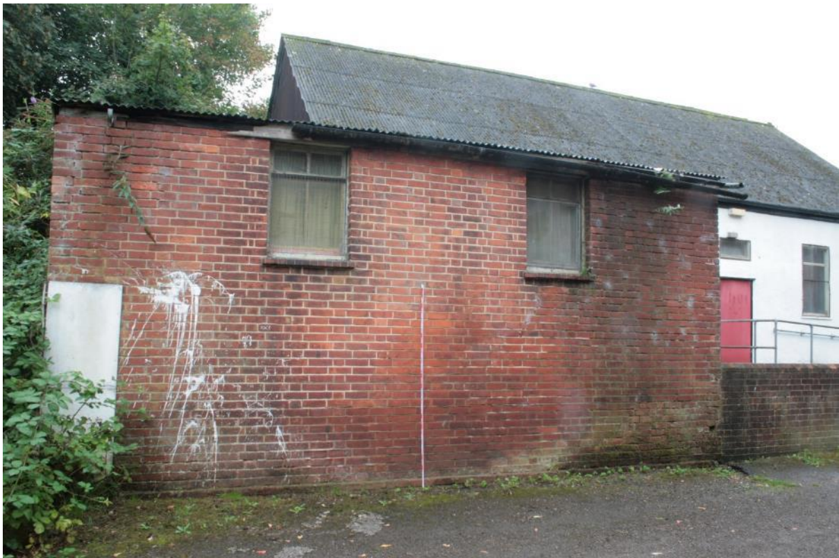
Plate 18: Brick extension at north-east corner of St George's Hall, looking south
