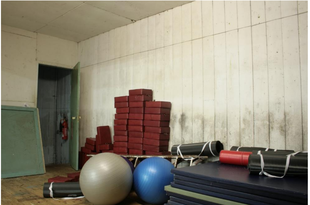
Plate 33: Back of stage area of St George's Hall, looking east
