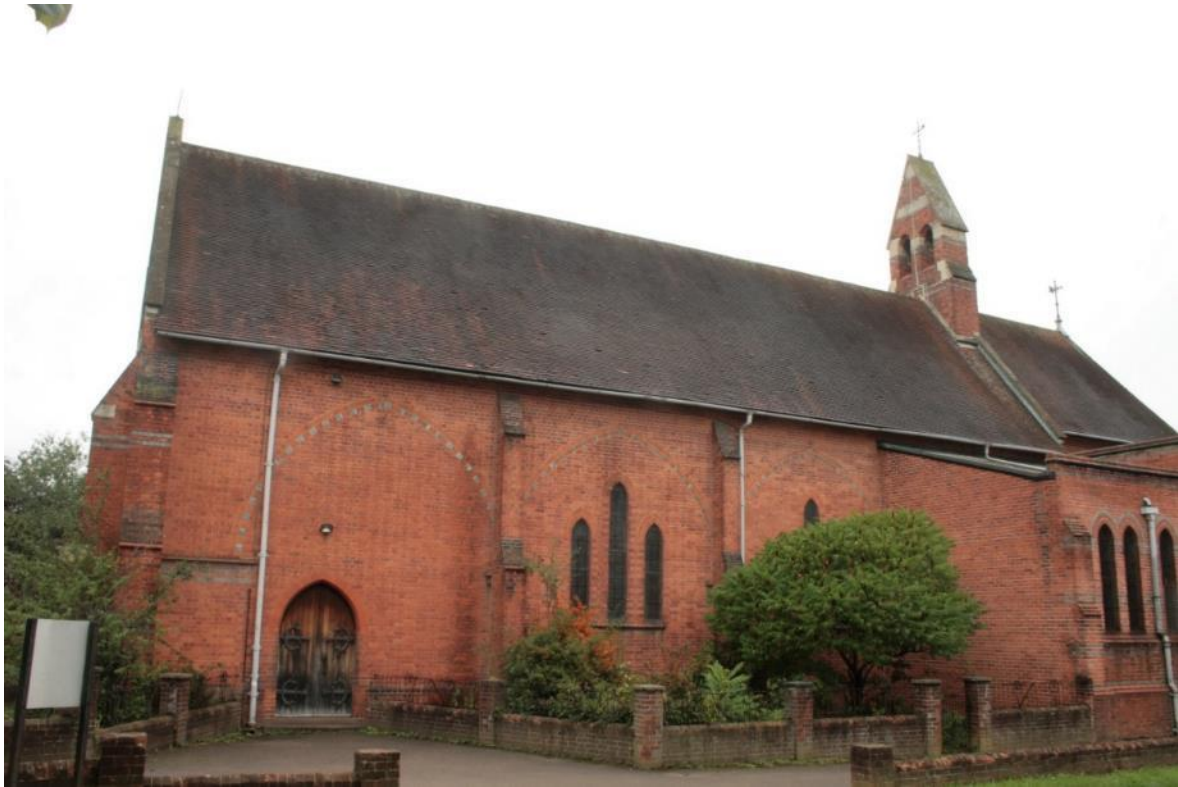
Plate 48: West end of the south elevation of St George's Church, looking north
