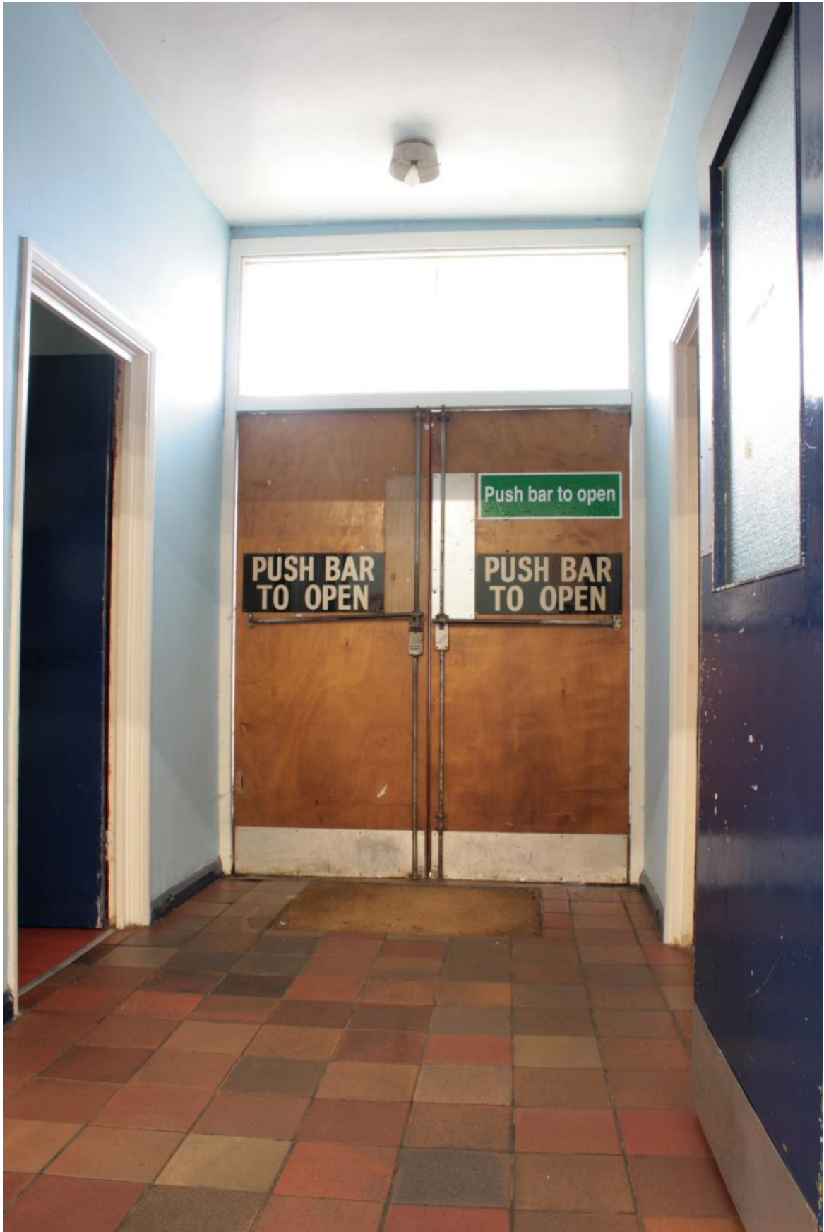
Plate 40: Front entrance hallway, looking west
