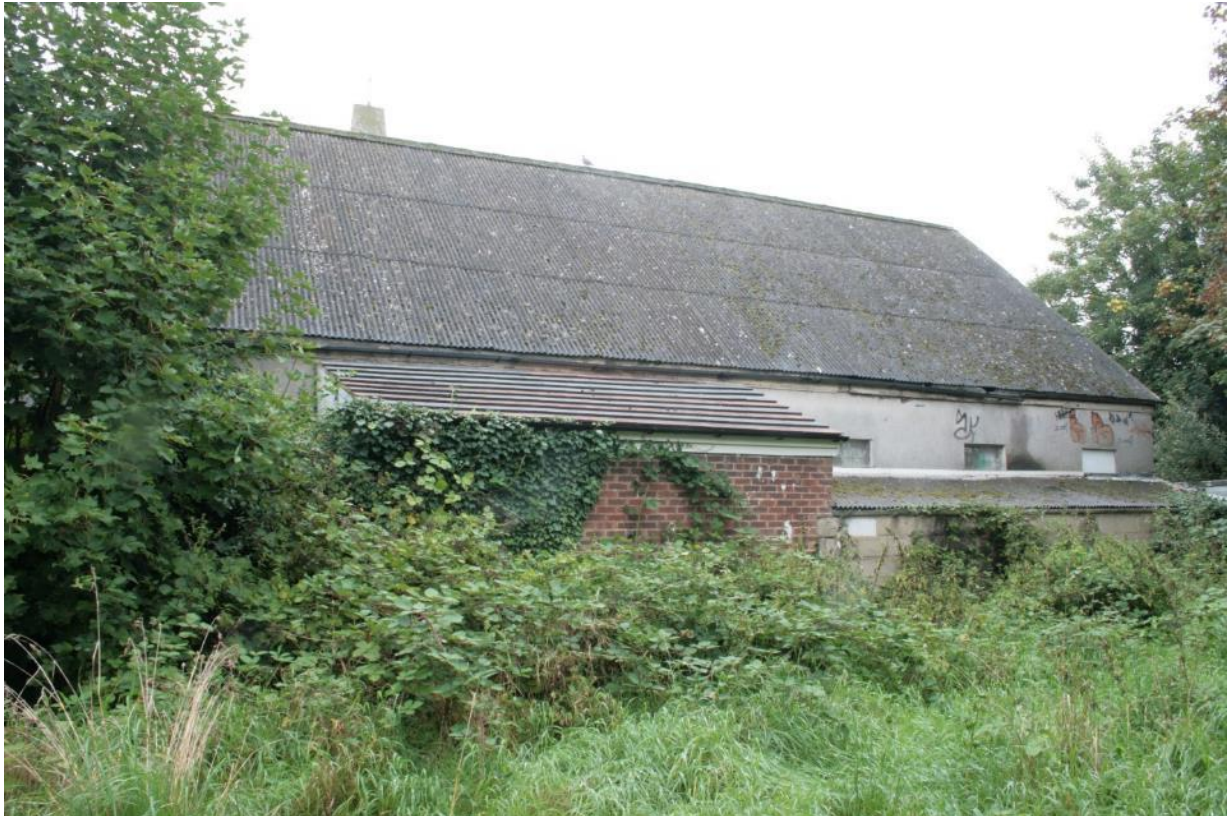
Plate 9: South (rear side) elevation and brick extension of St George's Hall, looking north
