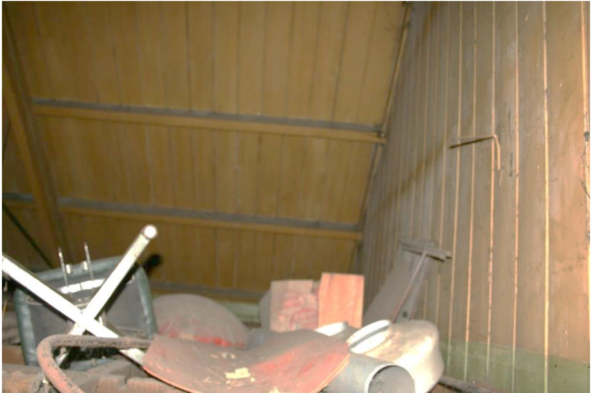
Plate 46: Roof space over main building showing purlins and rafters, looking north
