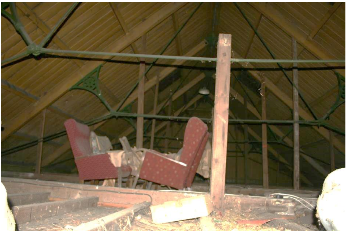
Plate 45: Roof space of showing roof trusses, looking west
