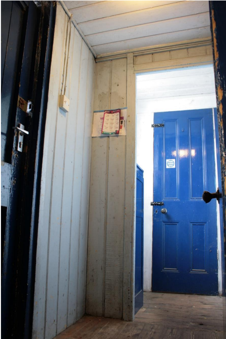
Plate 21: Side entrance into St George's Hall, looking north
