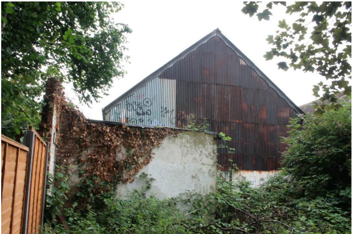
Plate 12: East (rear gable end) elevation of St George's Hall, looking west
