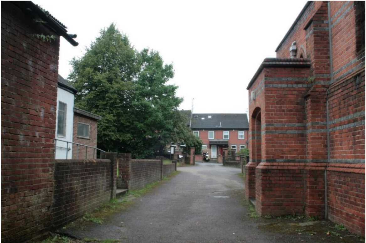
Plate 5: Access road between St George's Hall (left) and St George's Church (right), looking west
