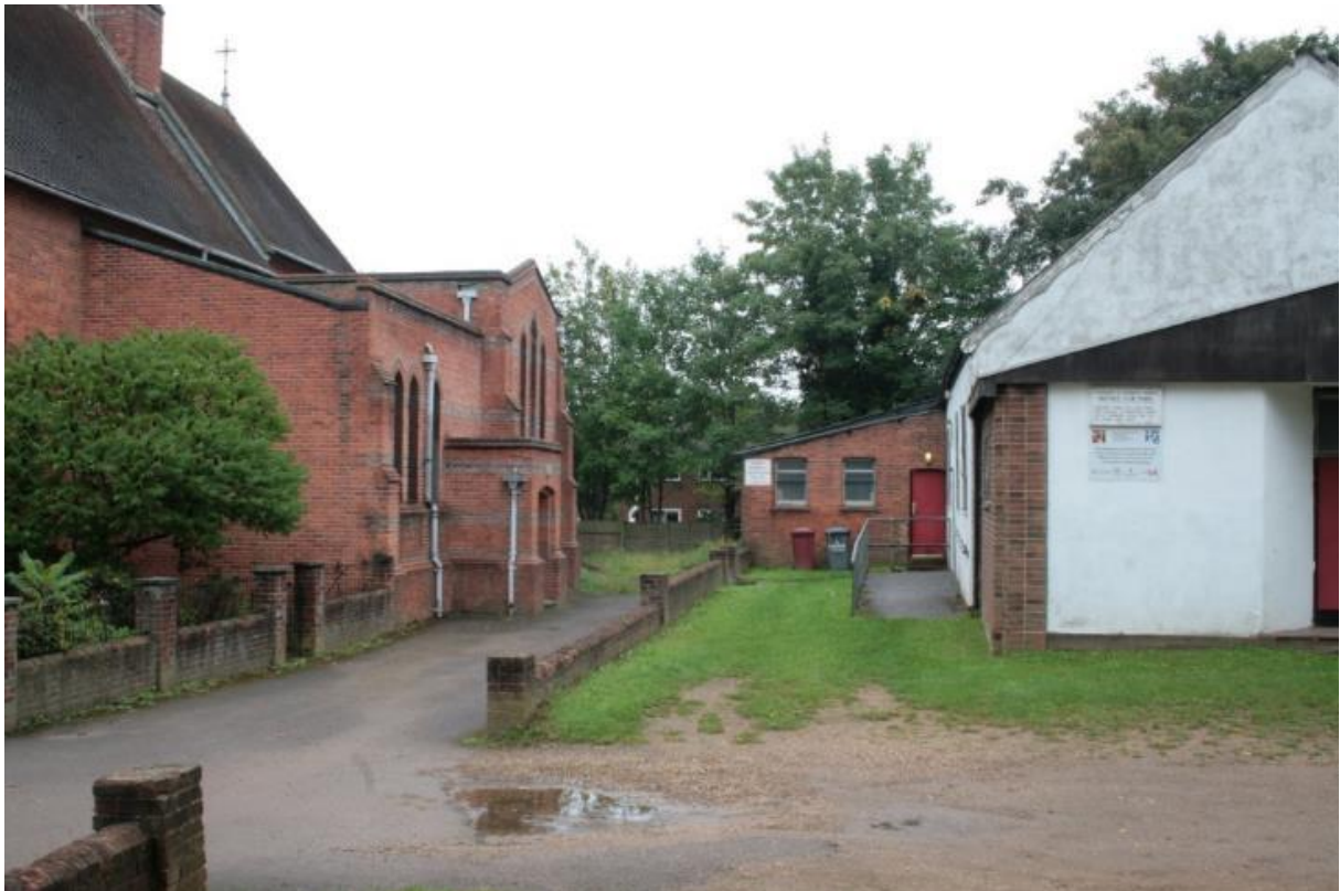
Plate 6: Access road between St George's Hall (right) and St George's Church (left), looking east
