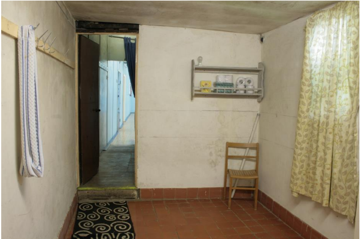
Plate 37: Entrance to male toilets at rear of St George's Hall, looking west
