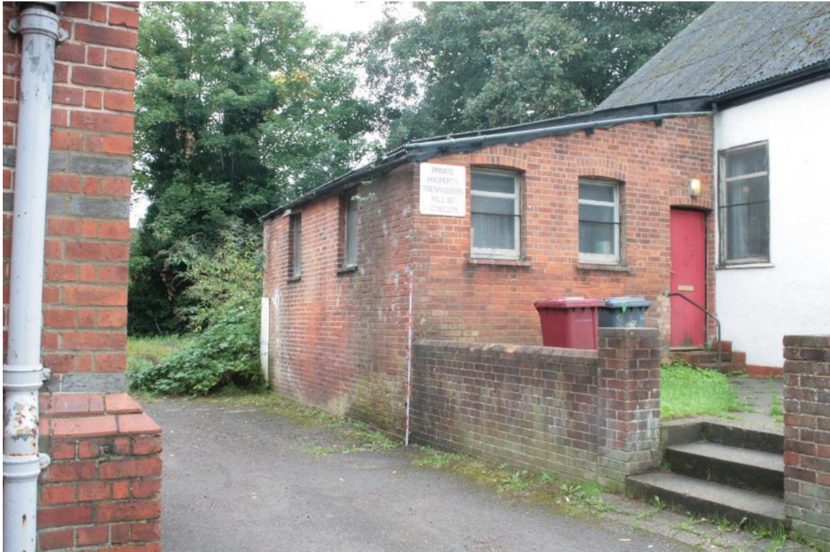
Plate 17: Brick extension at north-east corner of St George's Hall, looking east
