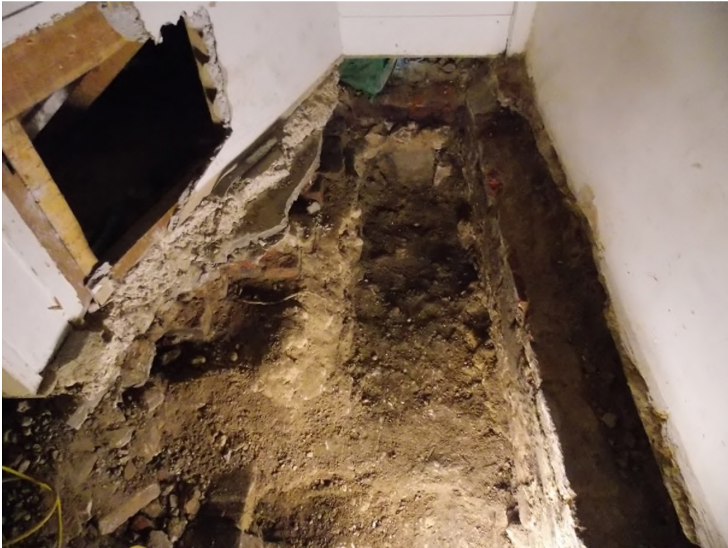
Plate 10: Ground reduction within the Receiver General's house
