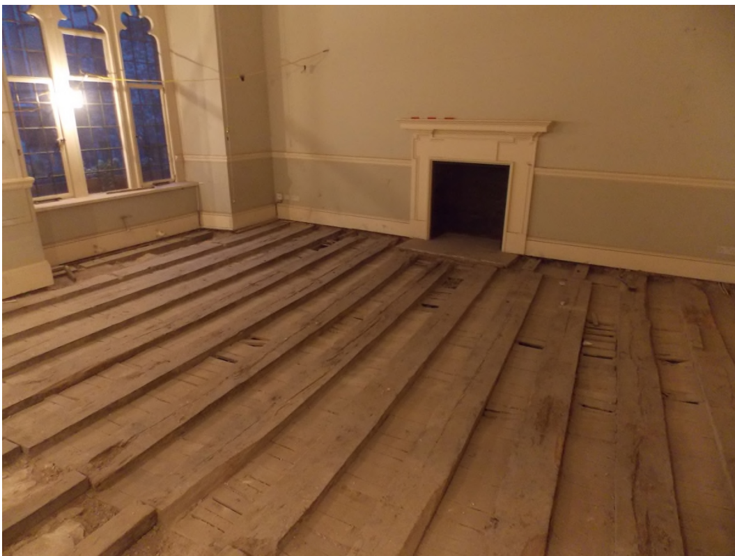
Plate 11: Floorboard removal in Room F6
