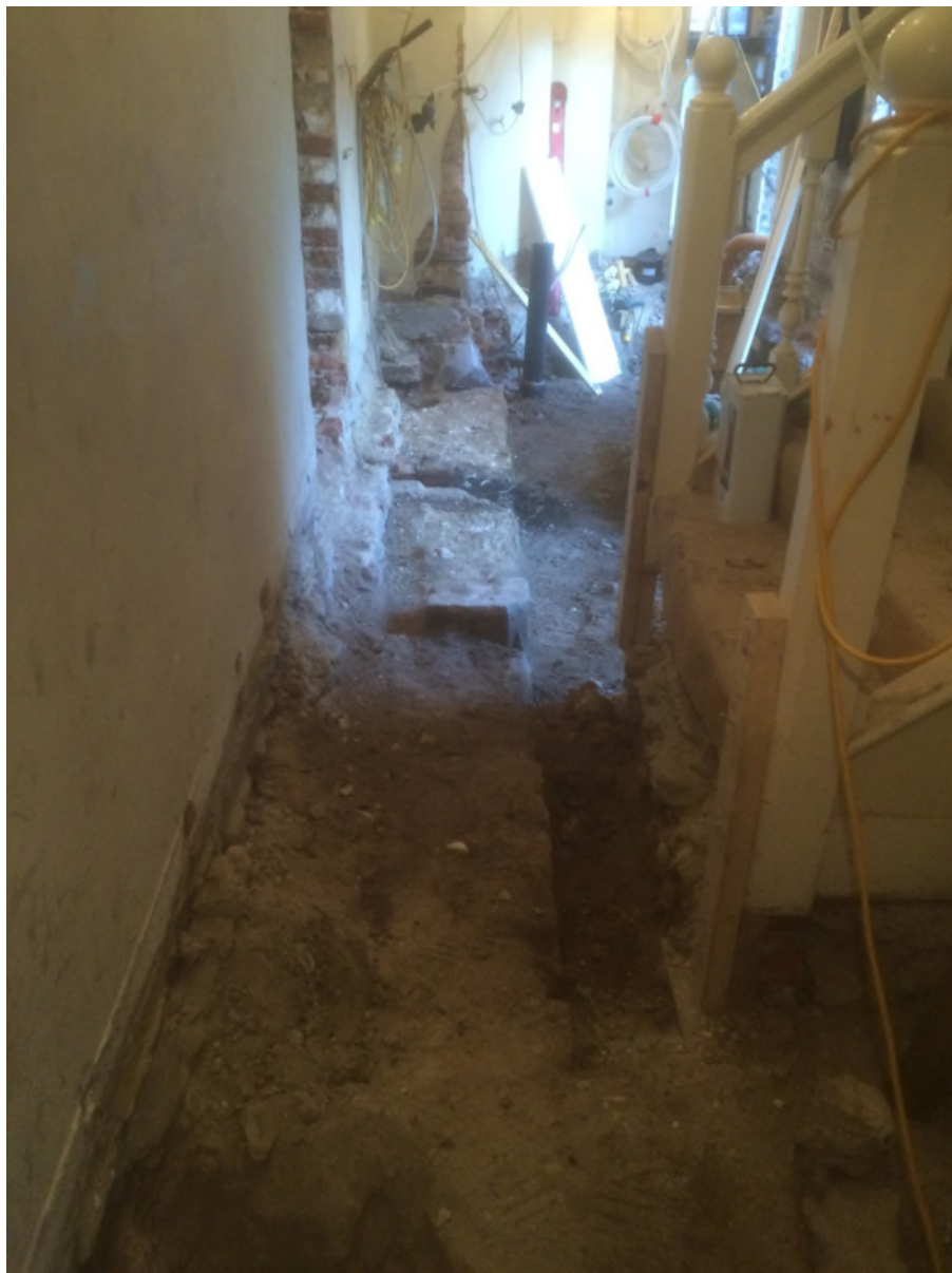
Plate 9: North facing excavation of Trench 3
