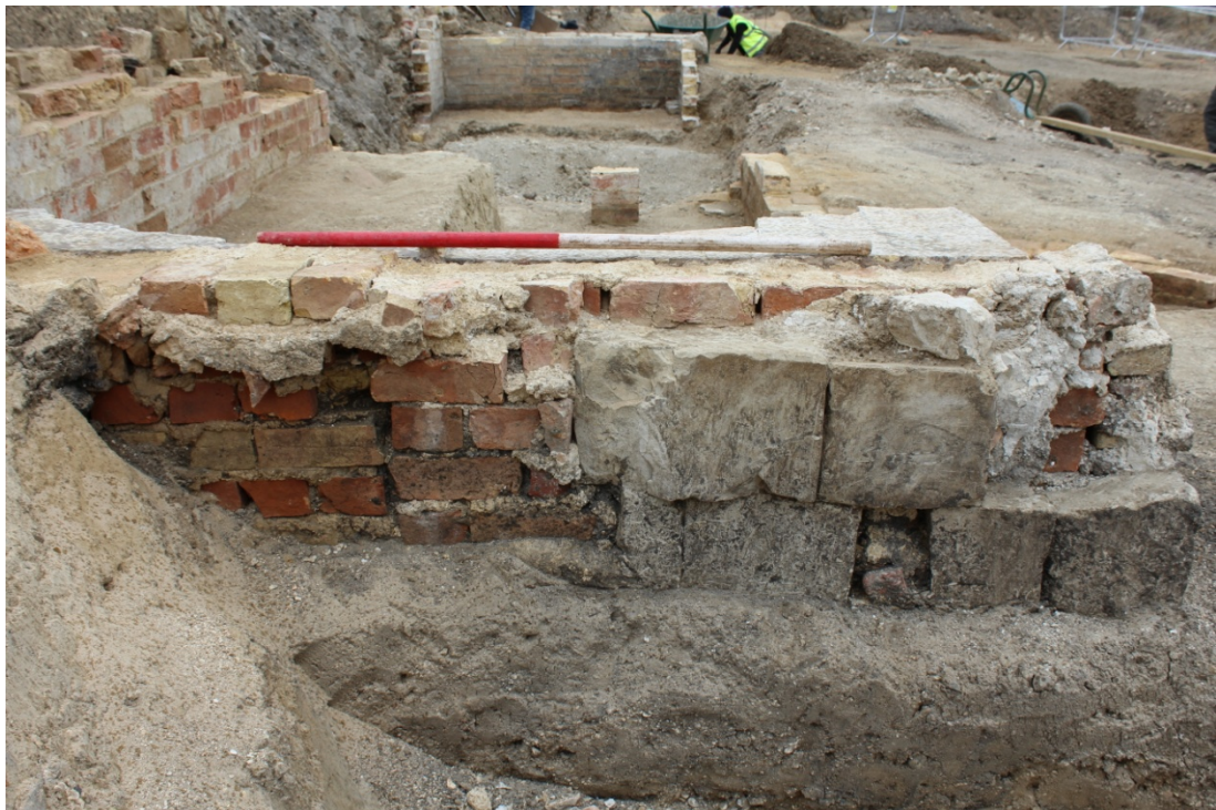
Plate 16: Wall [XXXX], taken from the east, typical wall construction of brick and clunch.
