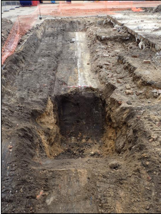
Plate 12 Trench 6 facing southeast, with 2.4m sondage in foreground.
