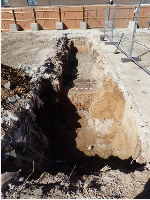
Plate 1 Trench 1 facing north-west, with sondage in foreground.
