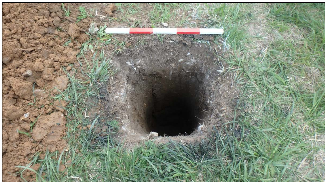
Plate 4, BH01 – Starter pit.
