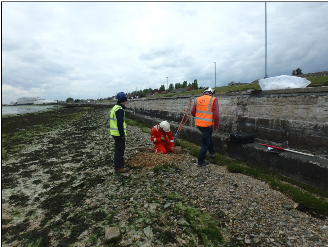
Plate 1, TP13 – Area 1, looking north west.
