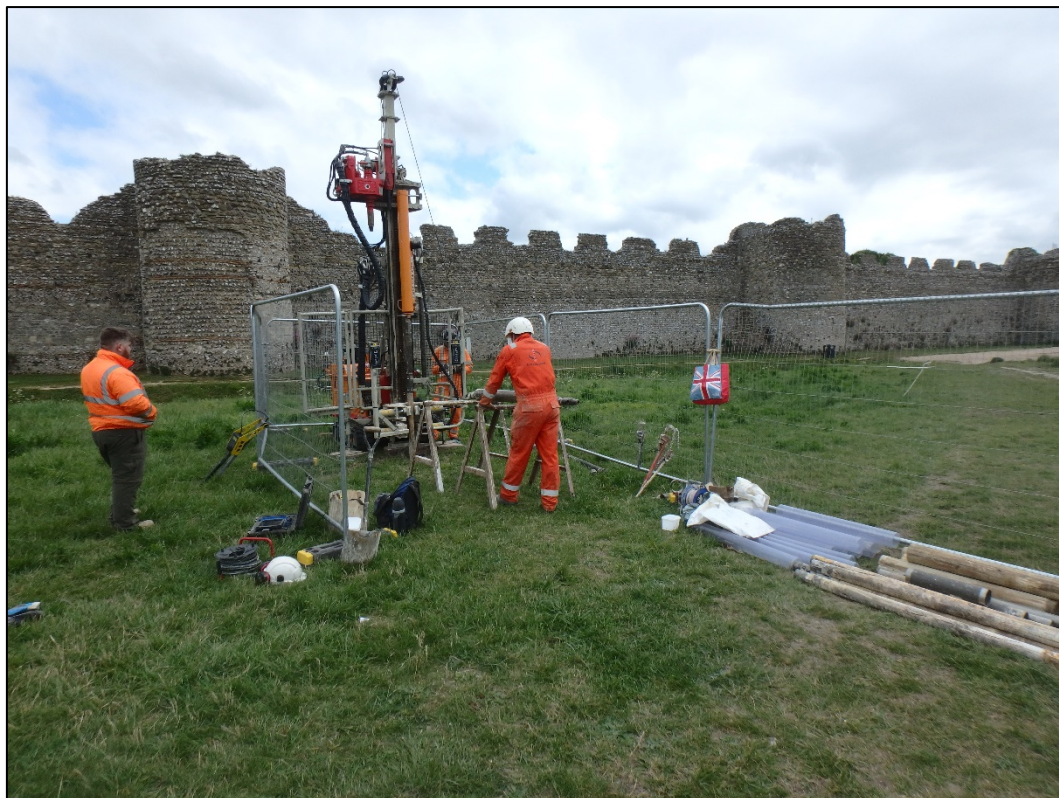
Plate 3, BH01 – Area 2, looking north.
