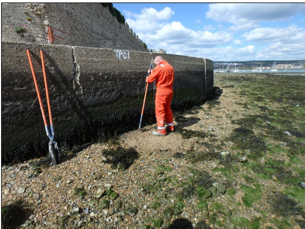
Plate 2, TP01 – Area 2, looking north west.
