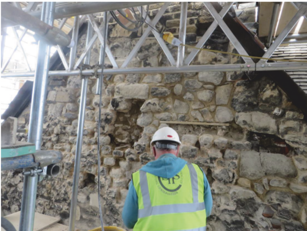
Plate 14: East gable wall of the Queen's House, looking south-west
