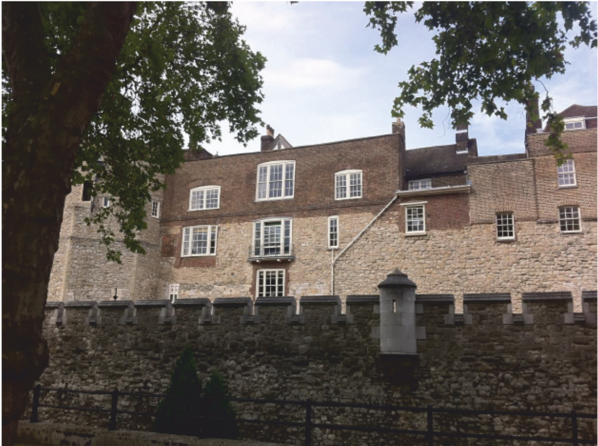
Plate 2: South elevation of the Inner Curtain Wall and Queen's House with the gable roof of the Queen's House Kitchen shown recessed back (centre right), looking north (photograph provided by HRP)
