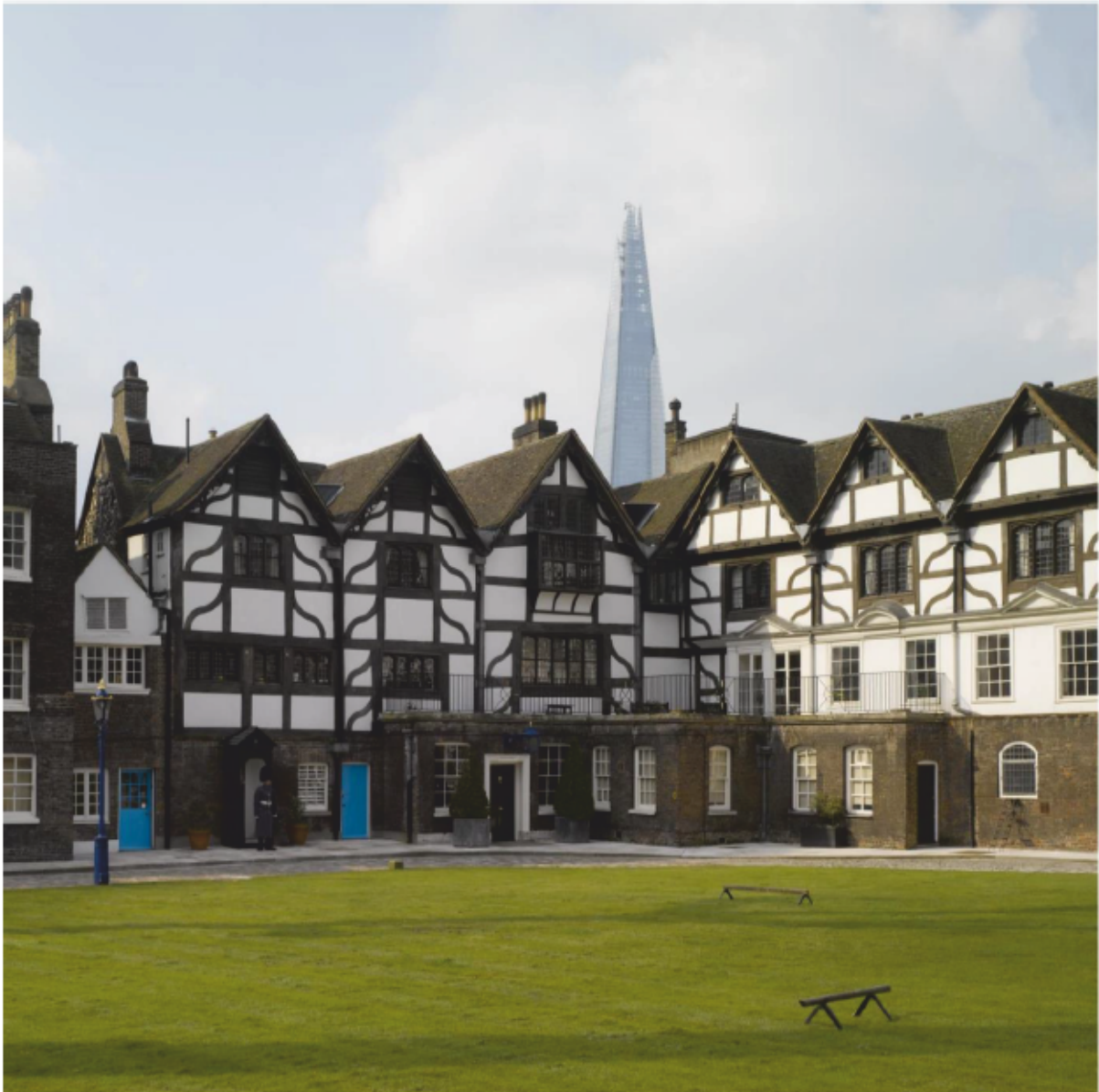
Plate 1: The Queen's House with the east gable end wall of the Queen's House Kitchen (left), looking south (photograph provided by HRP)
