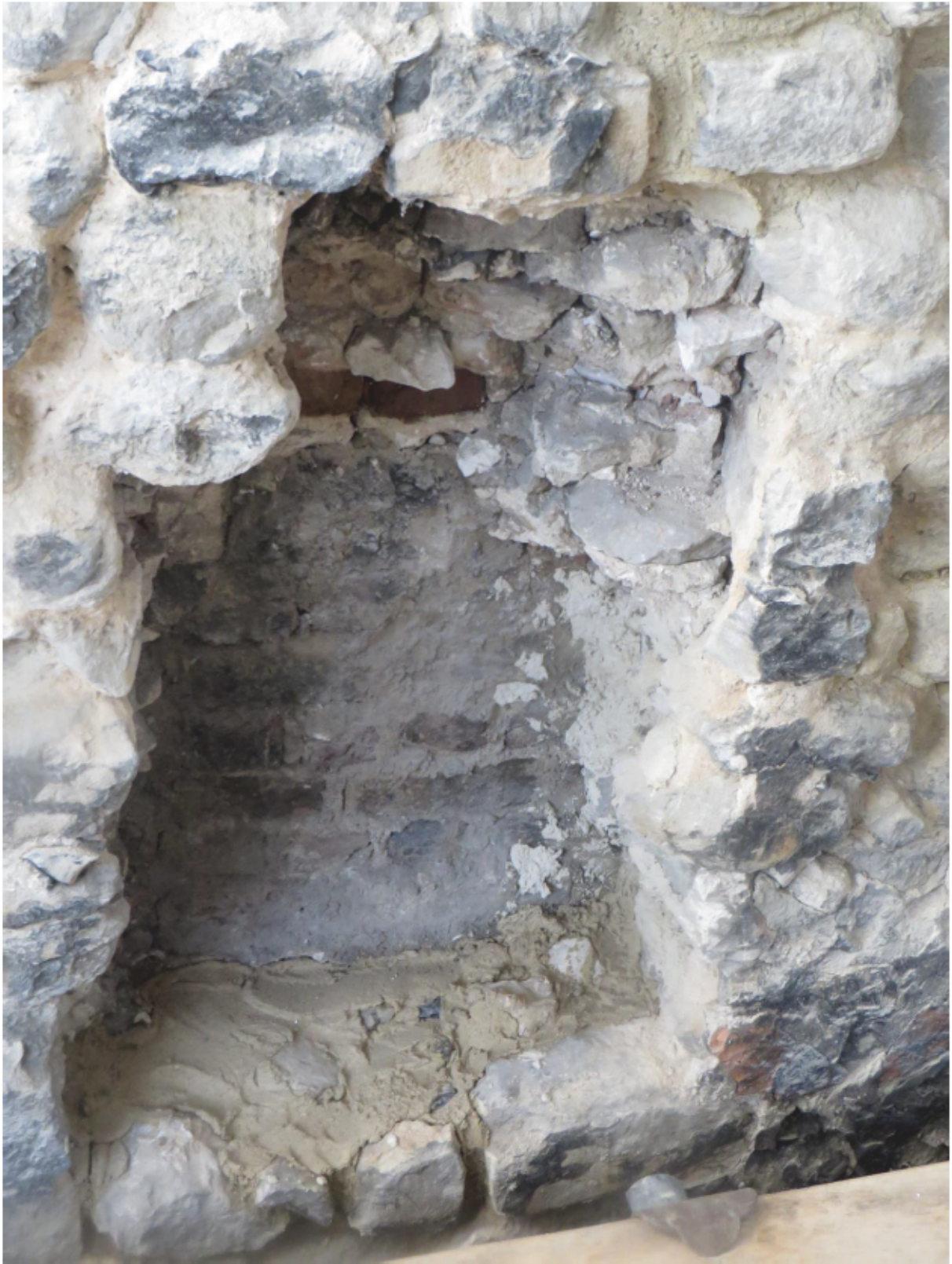
Plate 18: Infilled window in the east gable wall of the Queen's House, looking west
