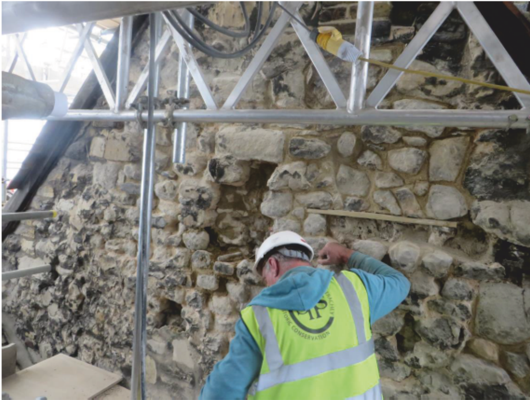
Plate 15: East gable wall of the Queen's House, looking south-west
