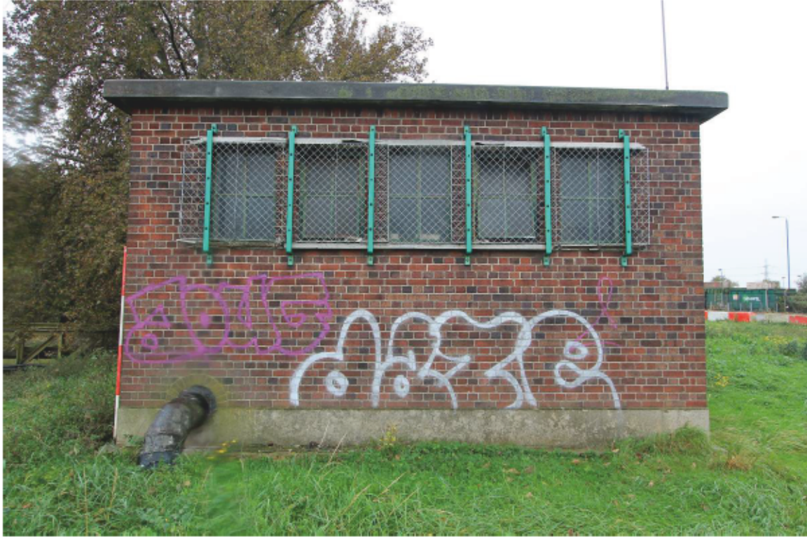
Plate 1 Building 1: looking south
