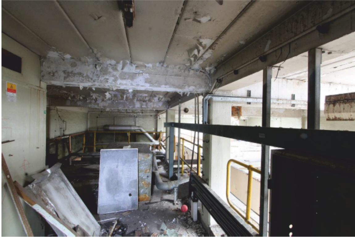
Plate 36 Building 13: Floor above central offices looking north
