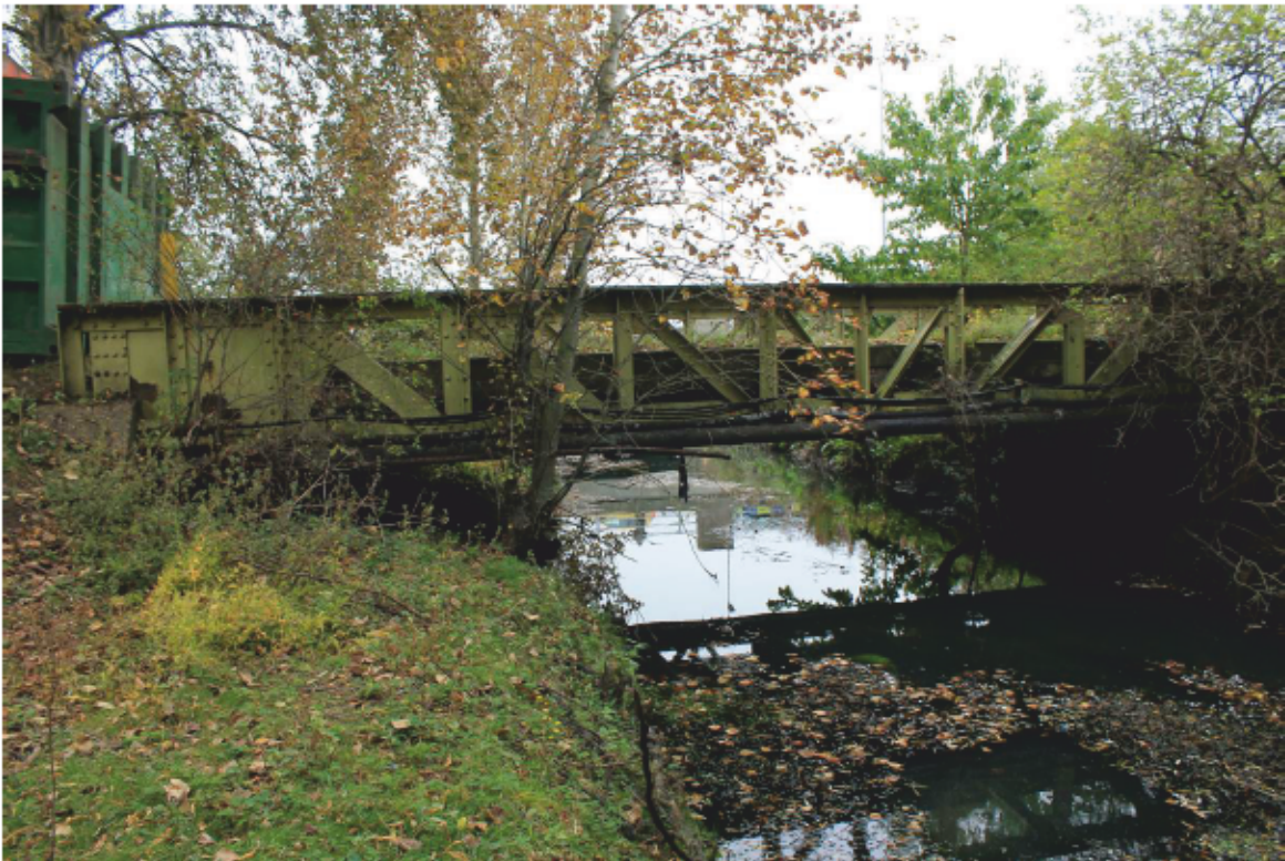
Plate 6 Bridge 3: looking north
