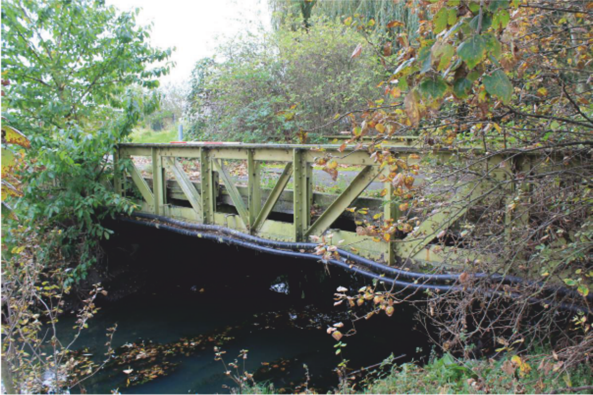
Plate 5 Bridge 3: looking north-west
