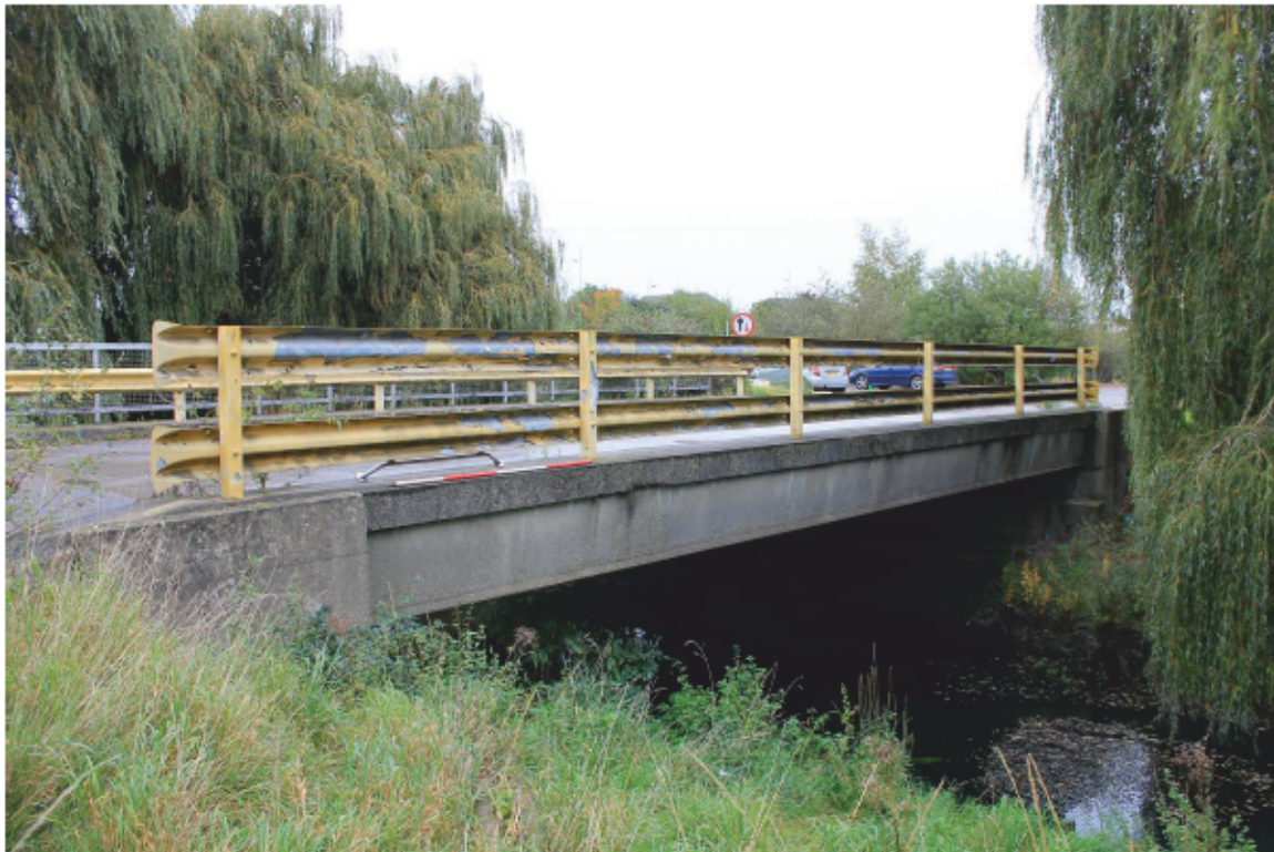
Plate 8 Bridge 4: looking north-east
