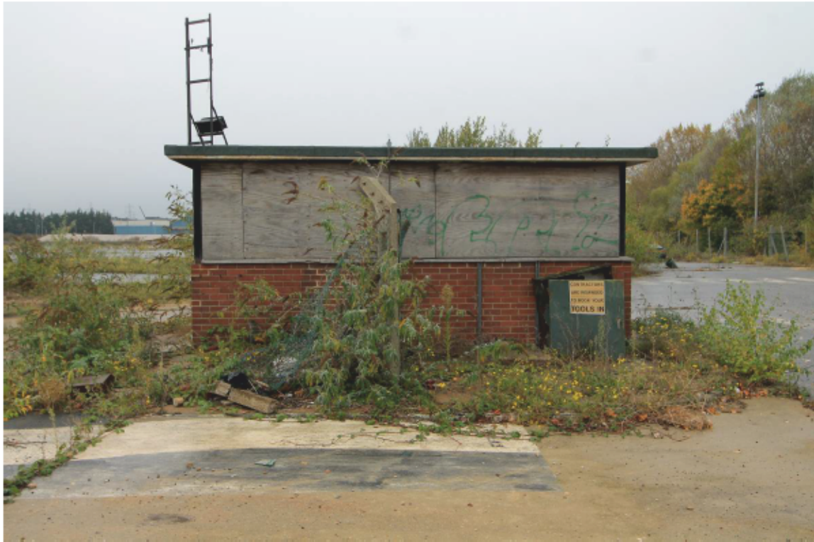
Plate 22 Building 11: Gatehouse No. 1, looking west
