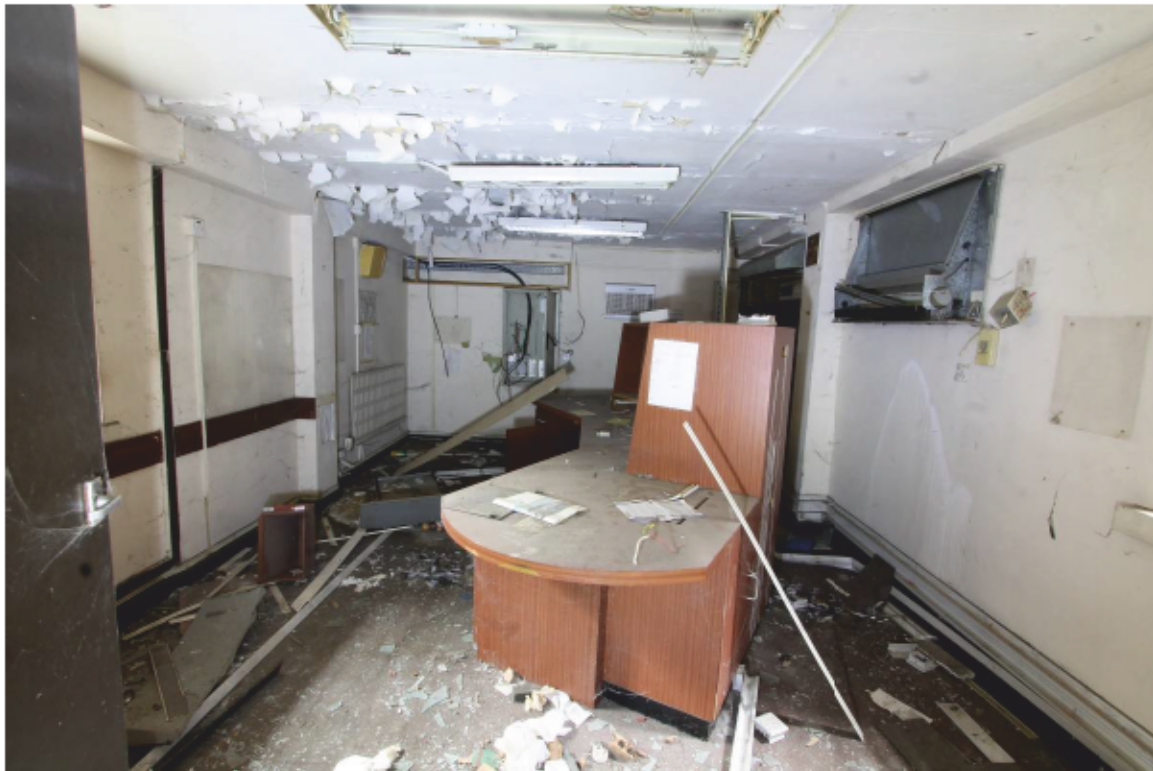
Plate 37 Building 13: Office (room 4)
