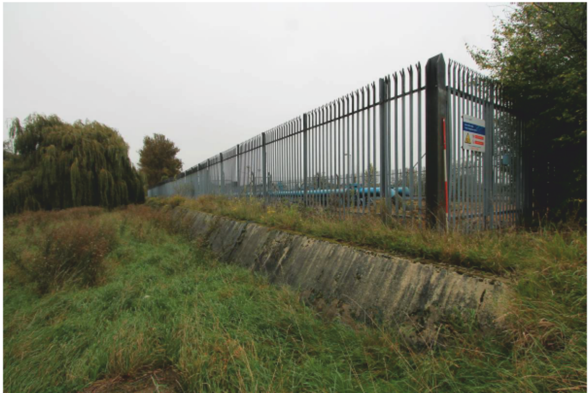
Plate 12 Building 6: Compound looking north-east
