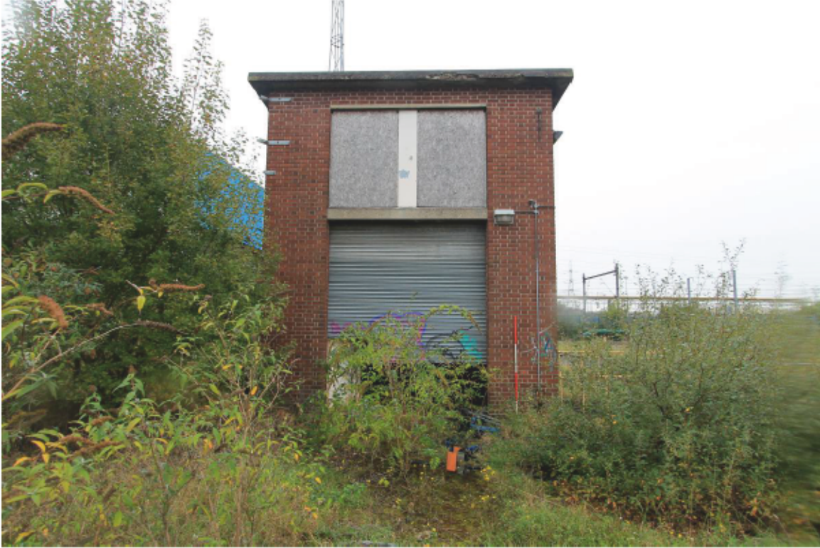
Plate 17 Building 8: Storm Water Pump House, looking south
