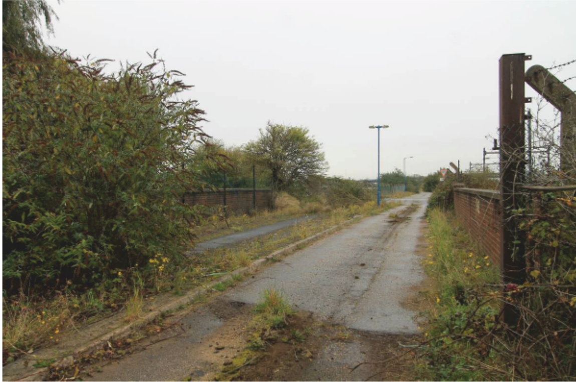
Plate 15 Bridge 7: Bridge deck, looking east
