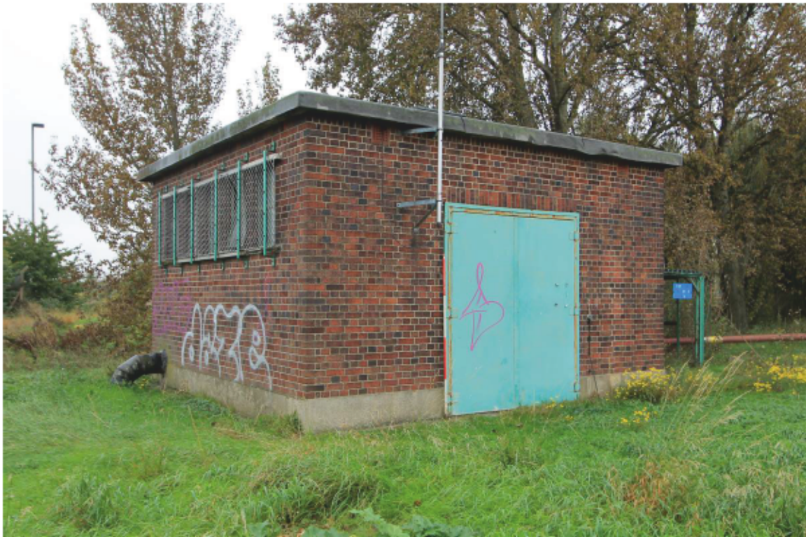
Plate 2 Building 1: looking south-east
