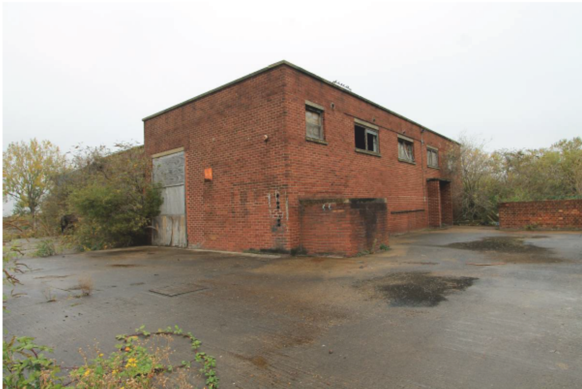
Plate 28 Building 13: Oil Storage, looking north-west
