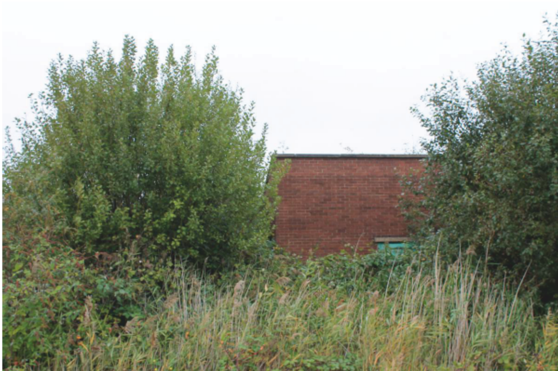
Plate 20 Building 10: Gas Meter House, looking north
