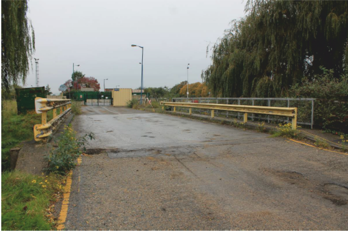
Plate 9 Bridge 4: Bridge deck, looking west
