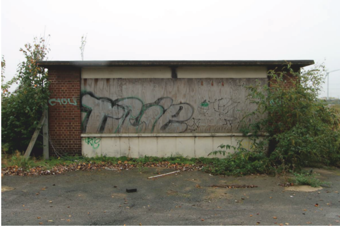
Plate 23 Building 12: Sewage Pump House, looking south
