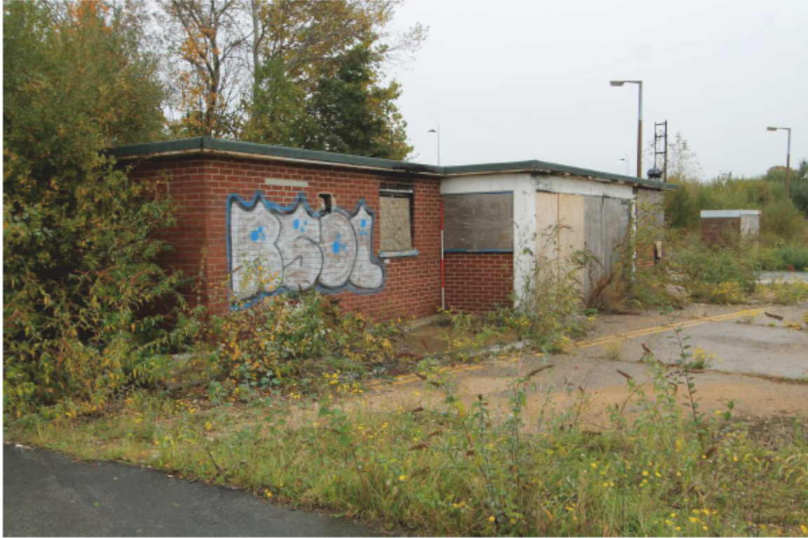
Plate 21 Building 11: Gate House No. 1 and Search Lodge, looking north-east
