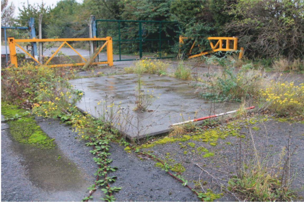
Plate 19 Building 9: Foundation of Barrier Gatehouse, looking north-west
