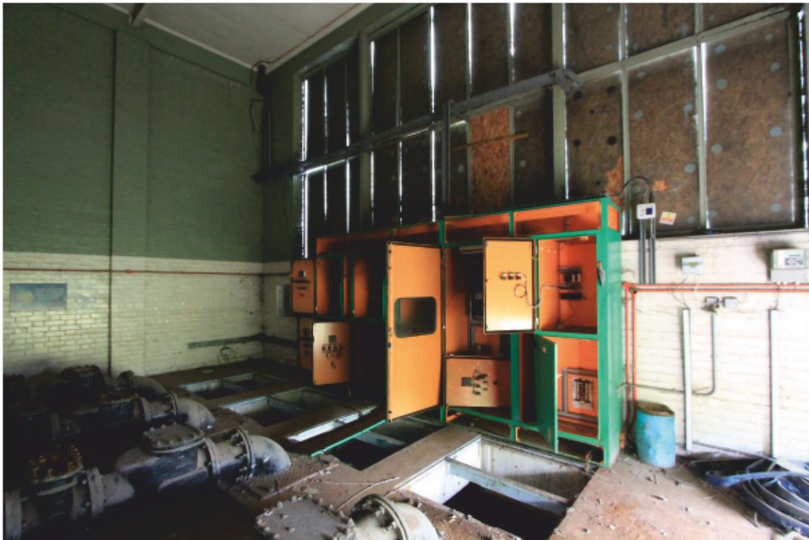
Plate 18 Building 8: Storm Water Pump House, Internal
