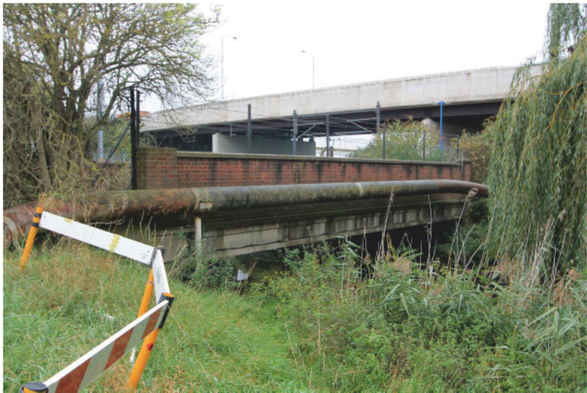
Plate 14 Bridge 7: looking south-west
