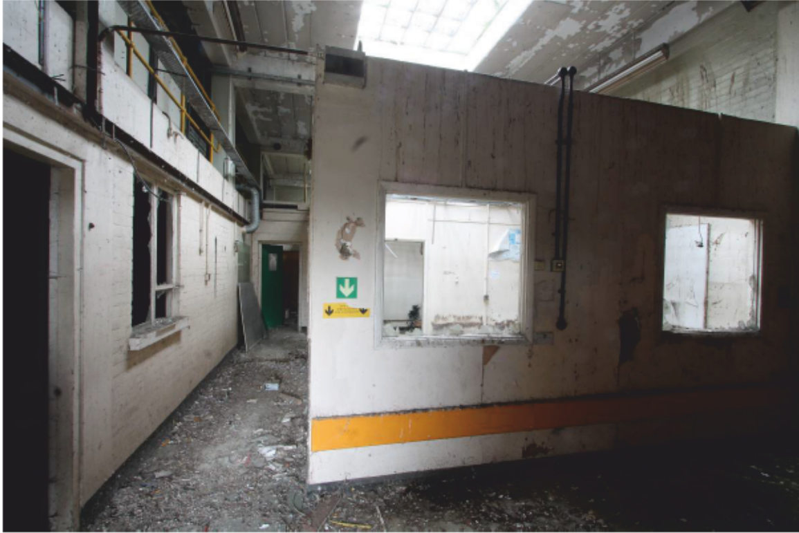
Plate 31 Building 13: Modern offices (right) inserted into eastern bays (formerly for appliance)
