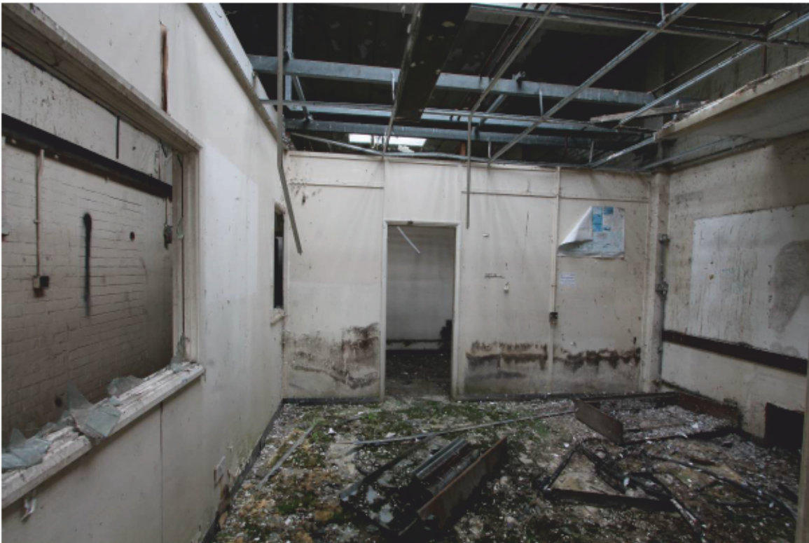
Plate 32 Building 13: Modern Office (room 14) looking north
