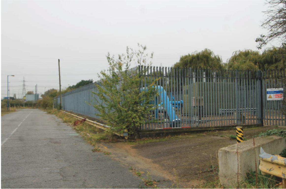
Plate 11 Building 6: Compound looking south-west
