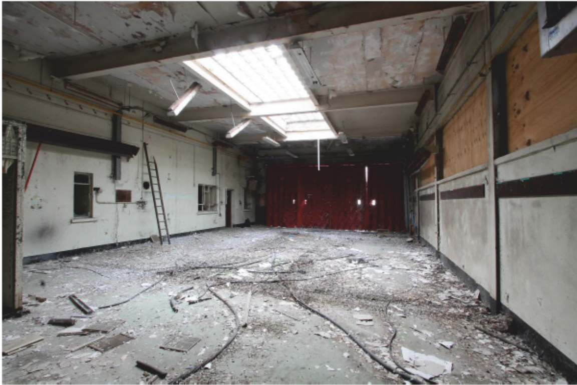
Plate 30 Building 13: Appliance Shed (room 10) looking south-east
