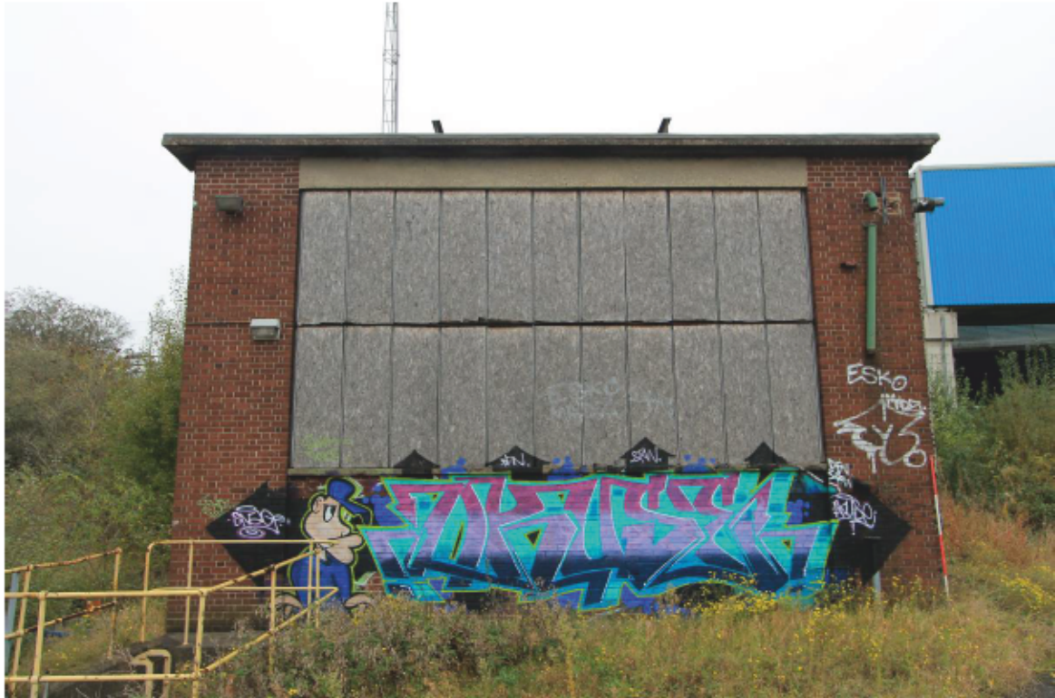
Plate 16 Building 8: Storm Water Pump House, looking east
