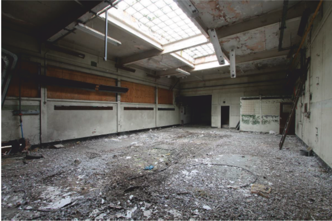
Plate 29 Building 13: Appliance Shed (room 10) looking north-west
