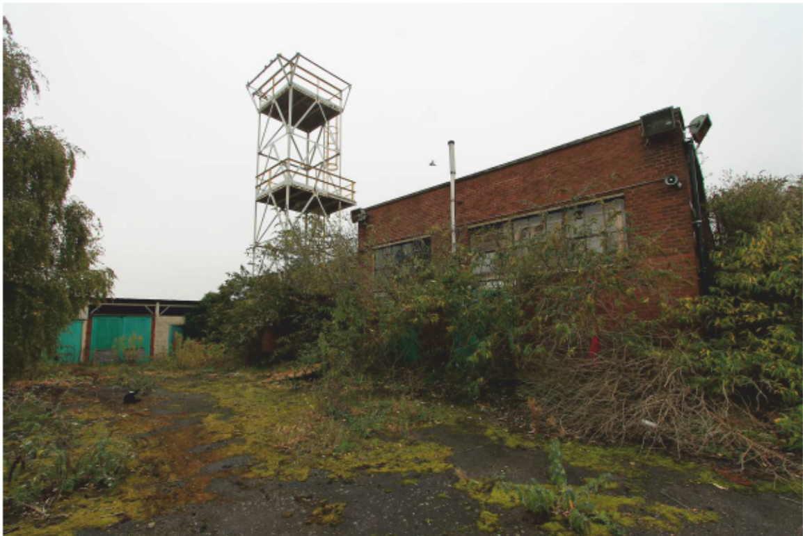
Plate 26 Building 13: Appliance house and Drill Tower, looking south-east
