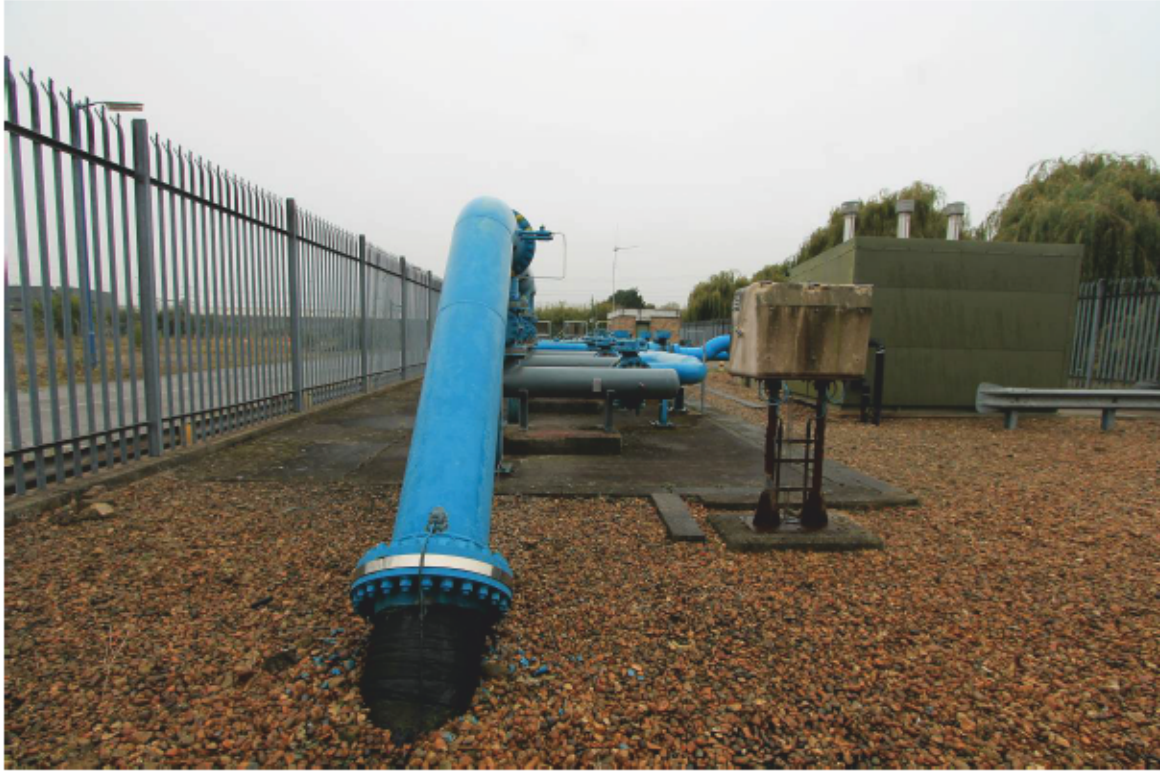
Plate 13 Building 6: View south inside compound
