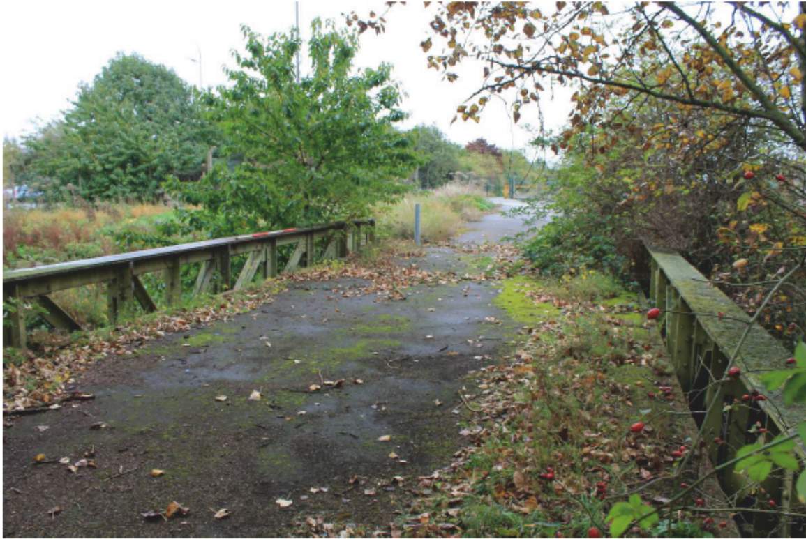
Plate 7 Bridge 3: Bridge deck, looking east
