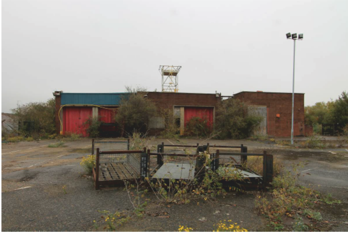
Plate 27 Building 13: Appliance House looking north
