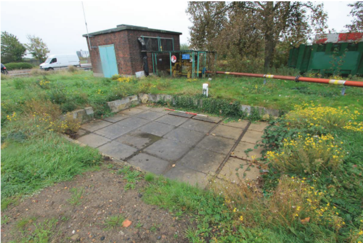
Plate 4 Building 2: looking north-east
