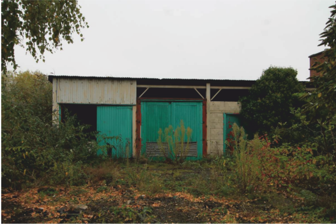
Plate 25 Building 13: Garage/store looking east
