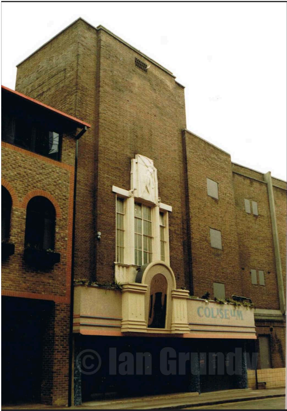
Historic Plate 16: The former Union Cinema, Gordon Street as the Coliseum Nightclub in 1988 (© Ian Grundy: Internet Source 2)
