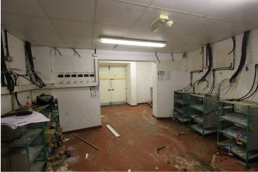
Plate 17 Cold storage area on ground floor
