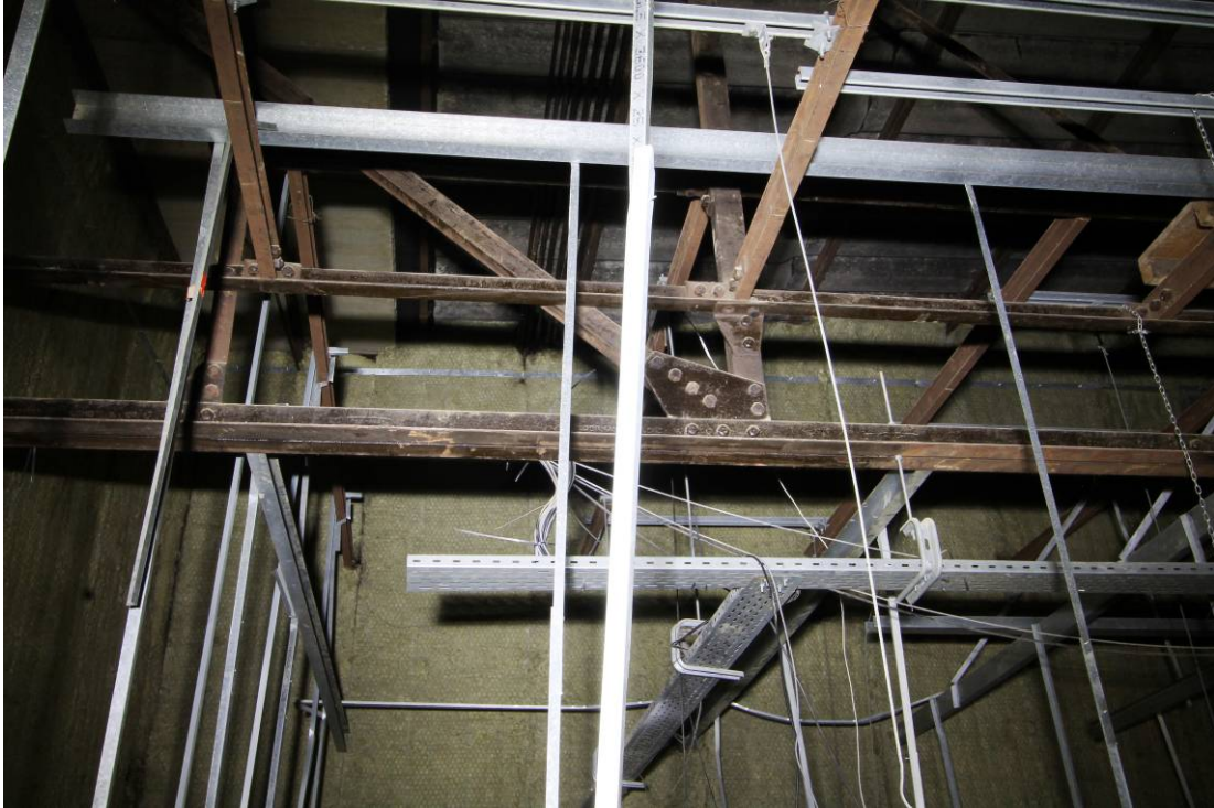
Plate 32 Remains of original steel superstructure
