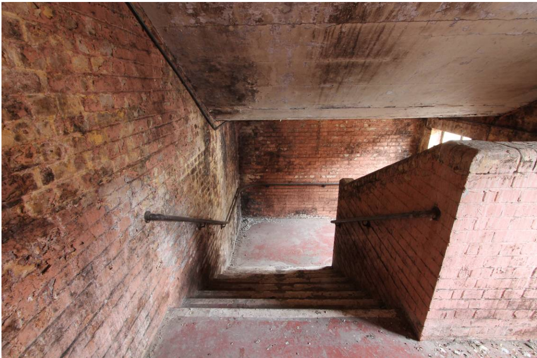
Plate 18 Original brick and concrete fire stair at second floor level
