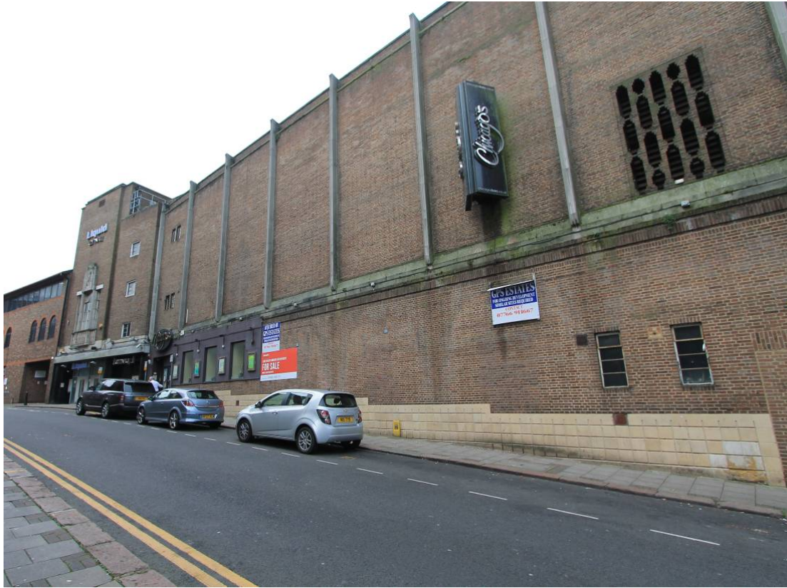
Plate 1 Front (east) elevation of the Former Union Cinema looking south-west
