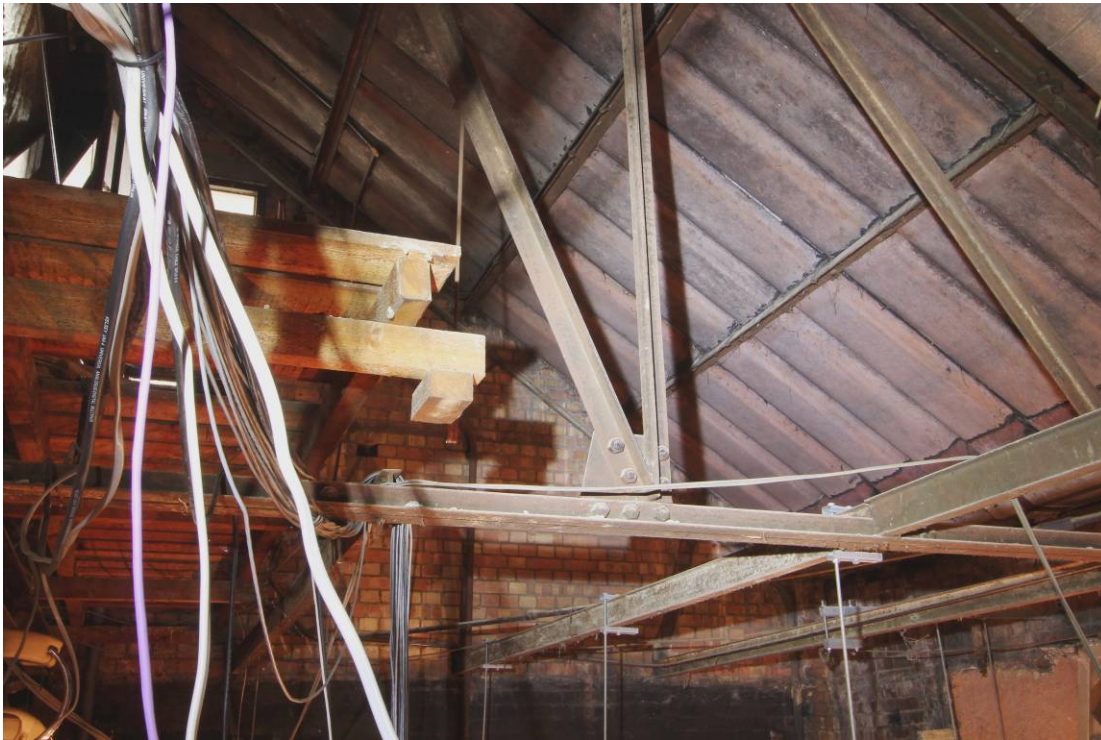
Plate 33 Section of roof truss
