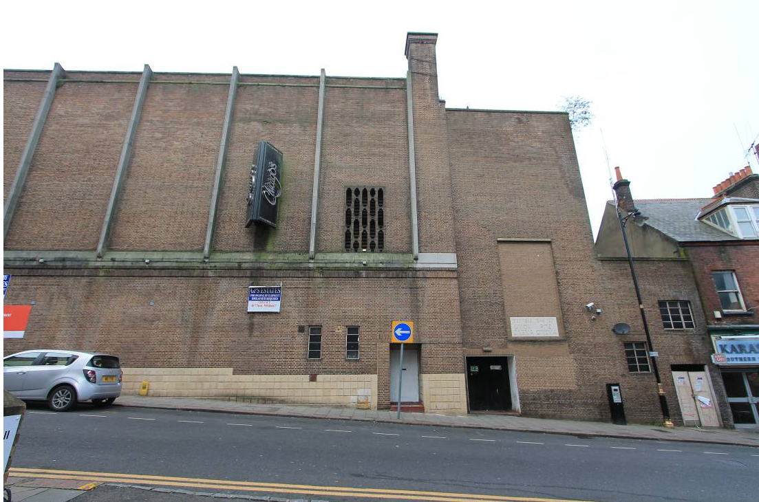
Plate 2 Northern end of the front (east) elevation of the Former Union Cinema looking west
