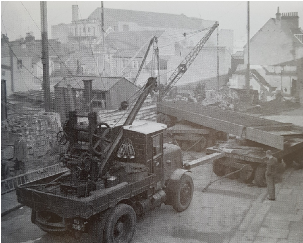
Historic Plate 4: Photograph taken c.1937 looking north-west from Gordon Street showing demolition of properties along Gordon Street, prior to the construction of the Union Cinema (© Grabham, 2007)
