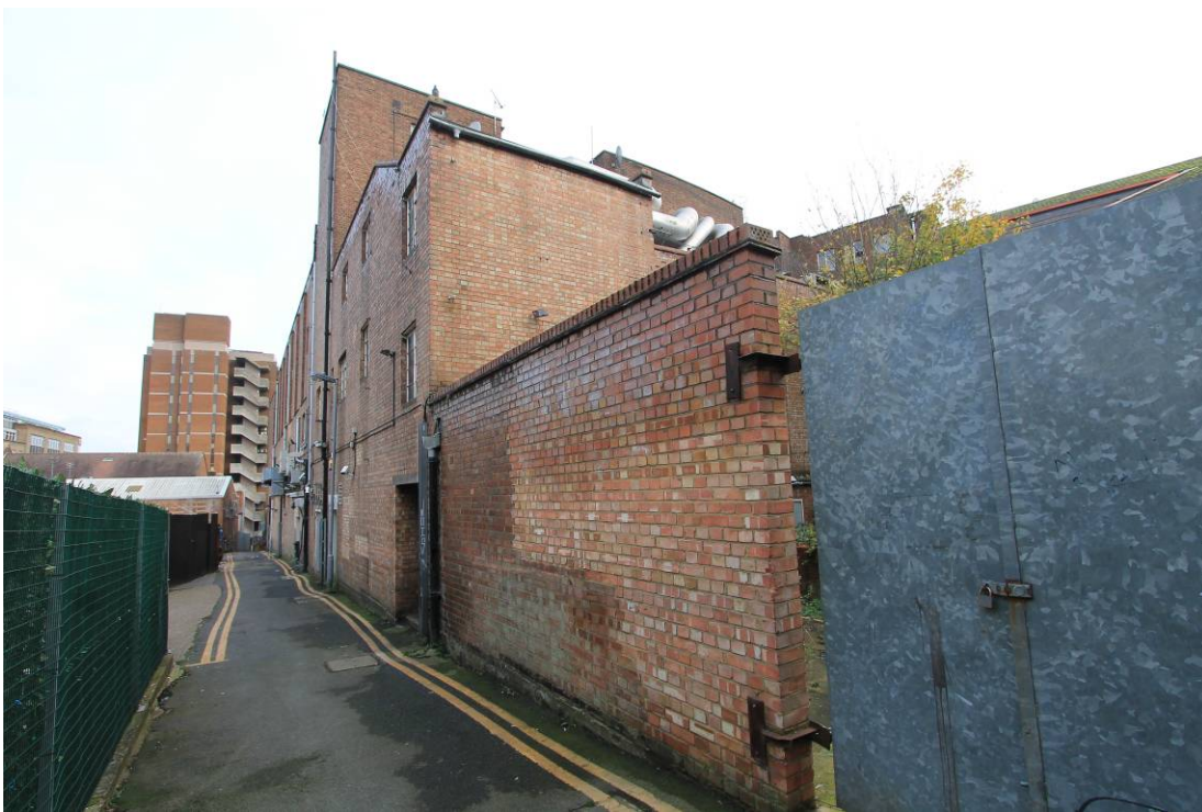
Plate 13 Rear elevation viewed from Lancrets Path, looking north
