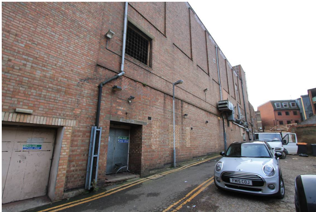
Plate 12 Rear elevation viewed from Lancrets Path, looking south
