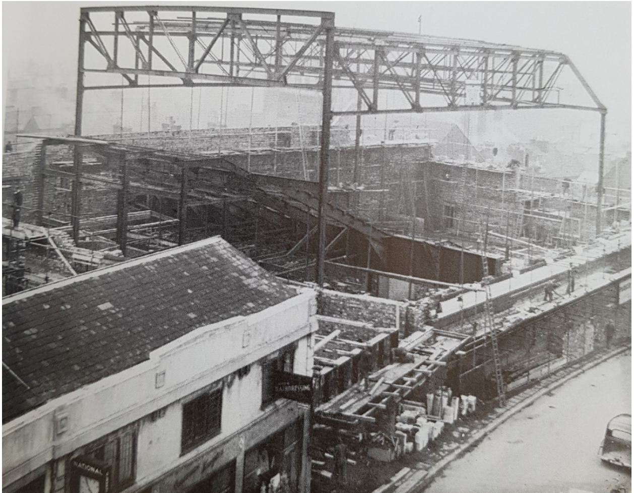
Historic Plate 5: Photograph taken c.1937 showing the steel frame for the roof and seats of the Union Cinema during construction (© Grabham, 2007)
