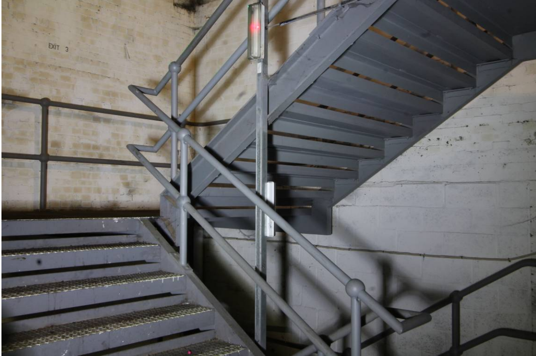
Plate 23 Modern steel fire escape stair
