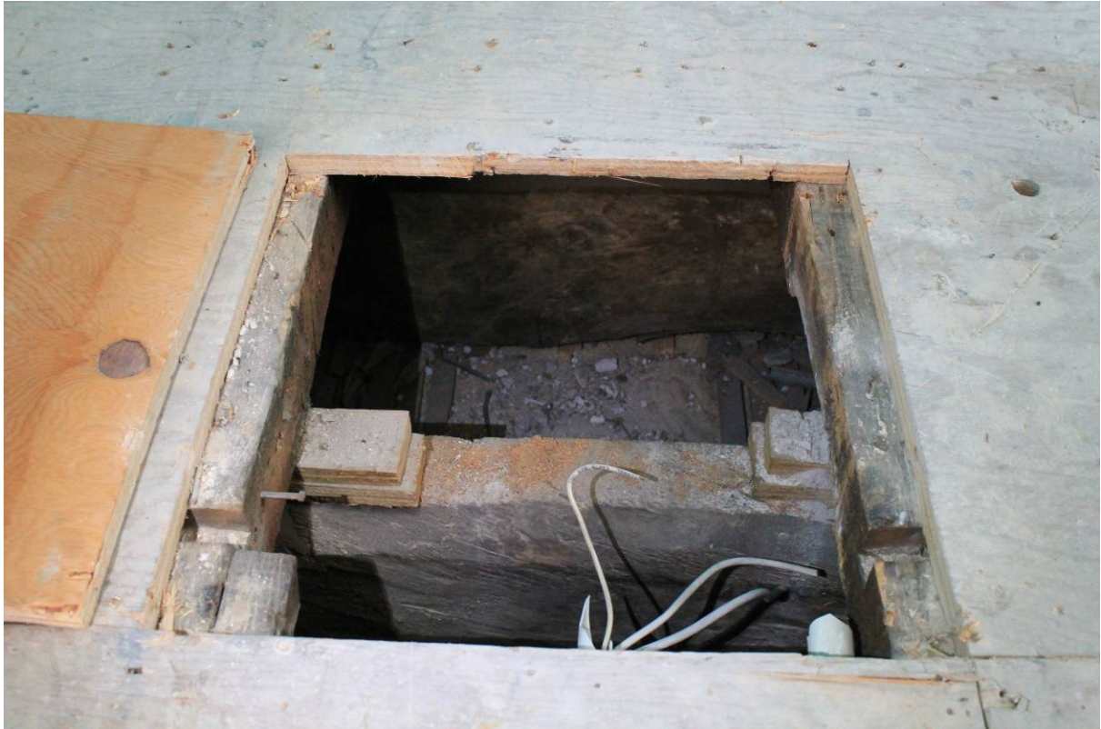
Plate 11 Floor joists seen in opening S8 (SF02), looking north
