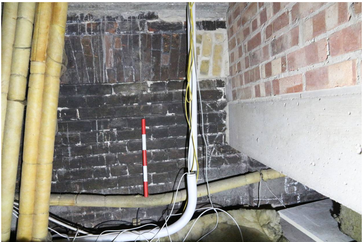
Plate 4 Blocked 17 th century window in former 17 th century former south wall (over FF09) seen through hatch (F3), looking north-east
