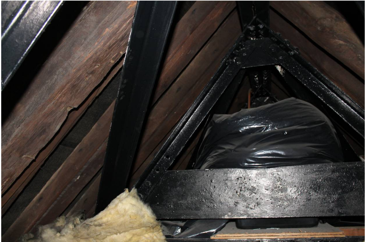
Plate 9 East roof and sub-structure, looking south from (S6)
