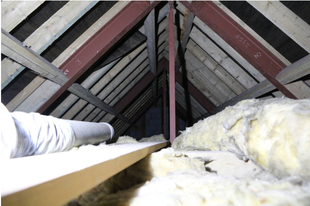
Plate 13 Roof over (SF11-SF13) looking west from (S12)
