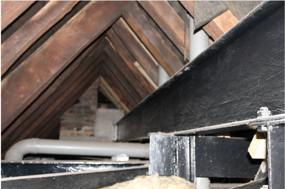
Plate 5 North roof and RSJ (from S2), looking east
