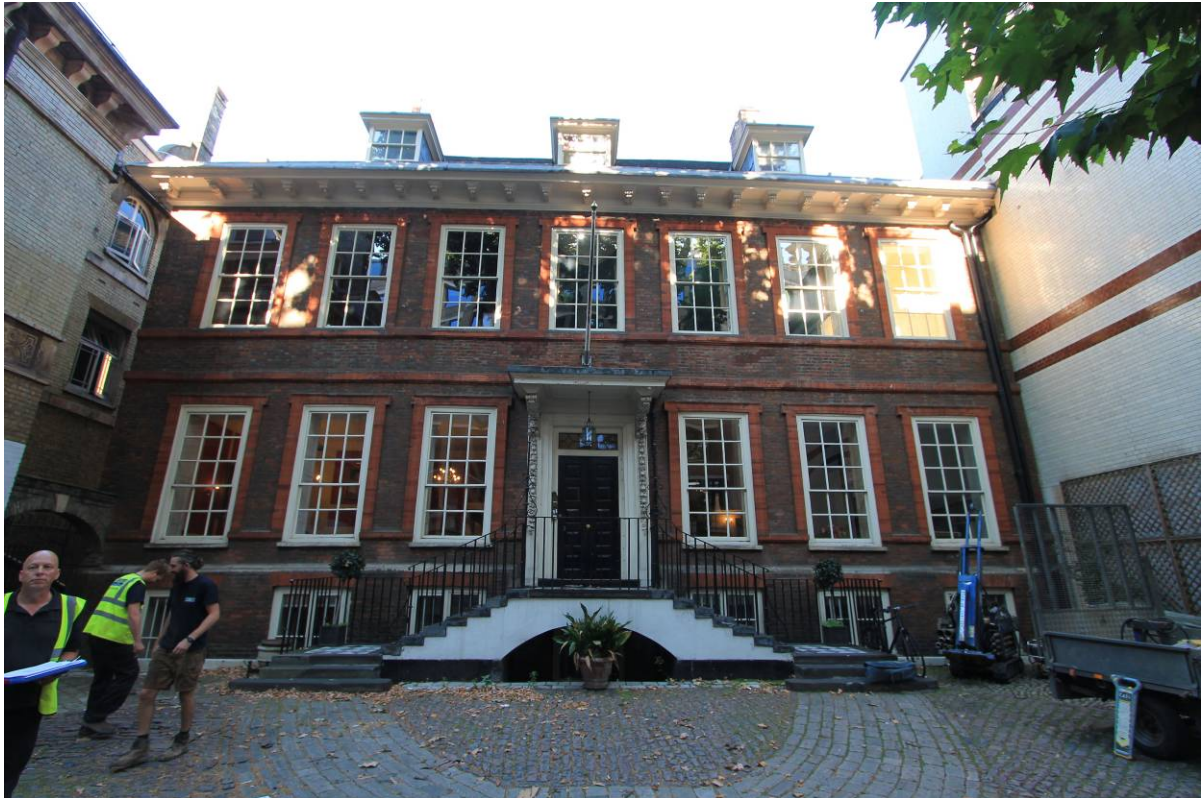
Plate 1a Principal Elevation, looking west
