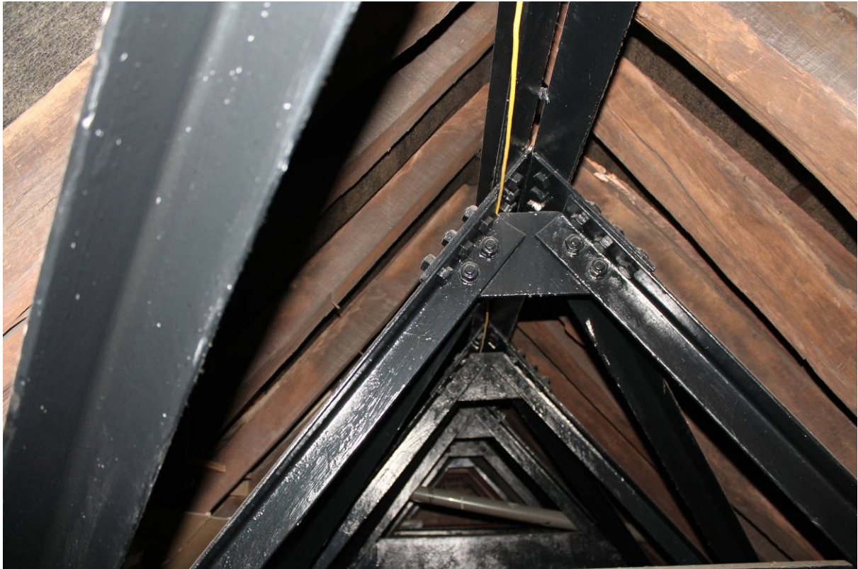
Plate 7 West roof and steel sub-structure, looking south
