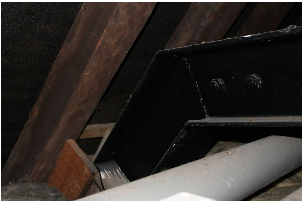
Plate 6 North roof and steel 'principal' bracing (from S2), looking north-east
