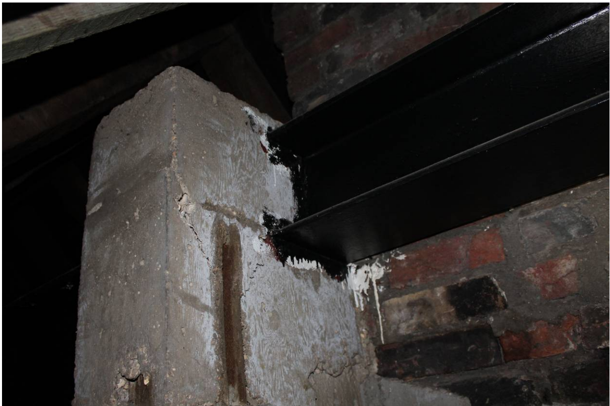
Plate 10 Supporting concrete structure tied into chimneystack looking north-west from (S6)
