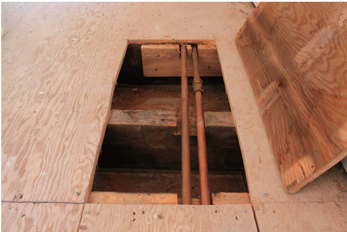
Plate 14 Floor joists in (SF13) within SF13
