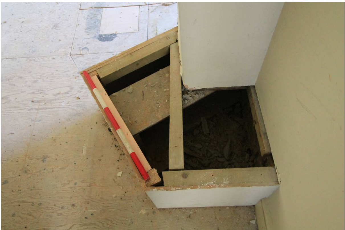
Plate 8 Steelwork carrying post, seen in (S5), looking south-west
