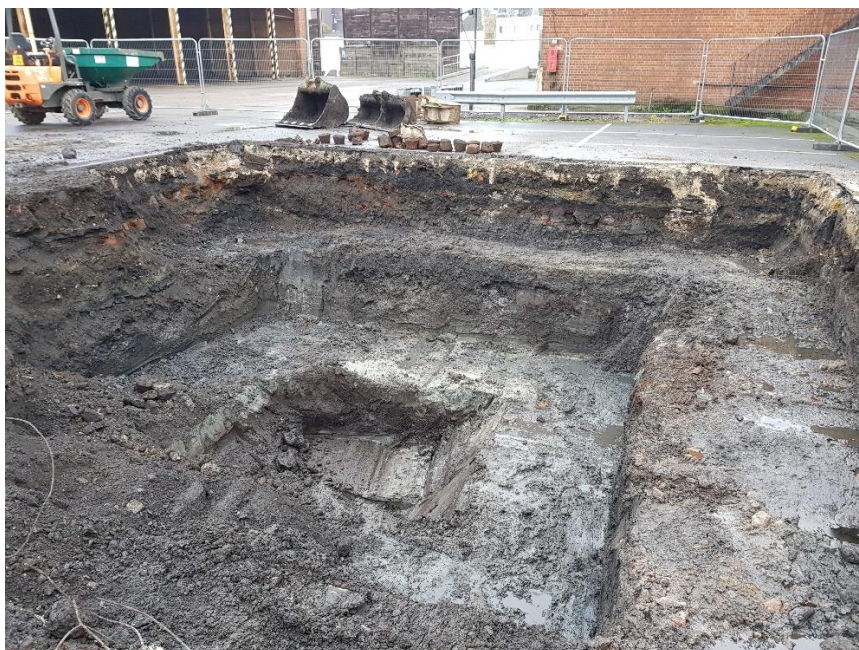
Plate 1: Trench 2, looking east
