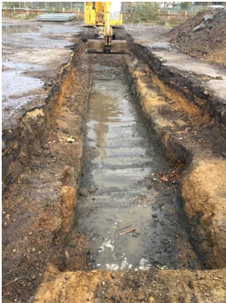
Plate 8: Trench 23 looking north
