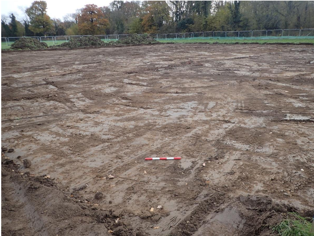
Plate 4 South tennis courts (Area 1) reduced to subsoil, facing south east.
