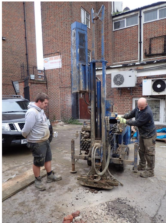
Plate 1: Geotechnical works on the site.
